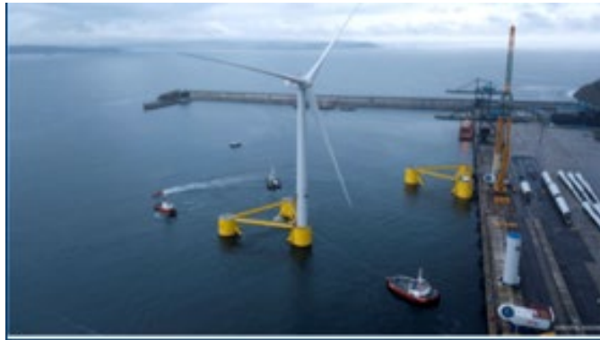
WTG Installation at Berth
