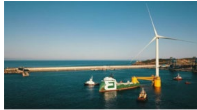
Tow to Installation Site
