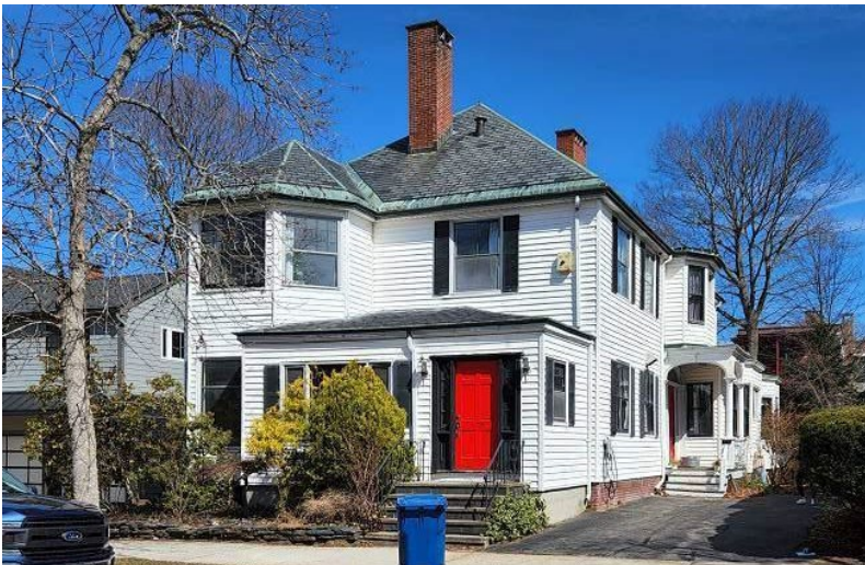
Figure 8: The current appearance of 175 Vaughan Street.
