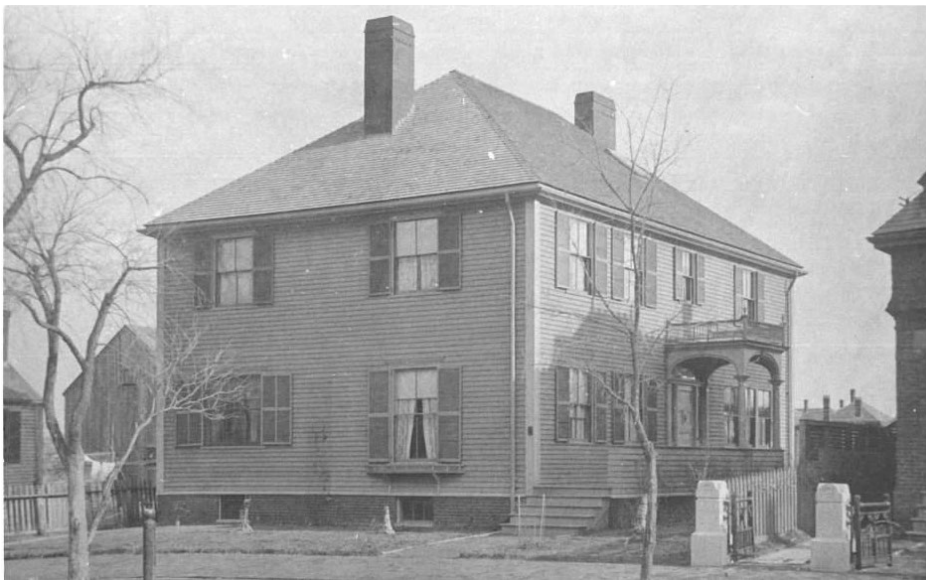
Figure 2: Undated Photograph (pre-1909) showing 175 Vaughan as originally designed by John Calvin Stevens for Cyrus F Davis, constructed in 1886.
