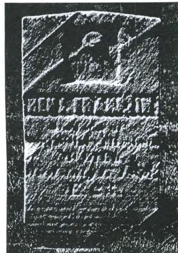
Deteriorated marble marker
