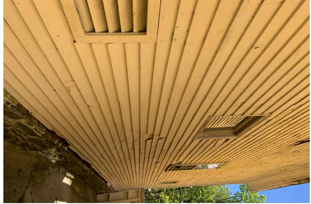
22 | East Elevation - main block - detail near center
