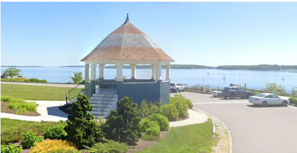
Figure 3: 2019 Google Street View image of the Eastern Promenade Gazebo.
