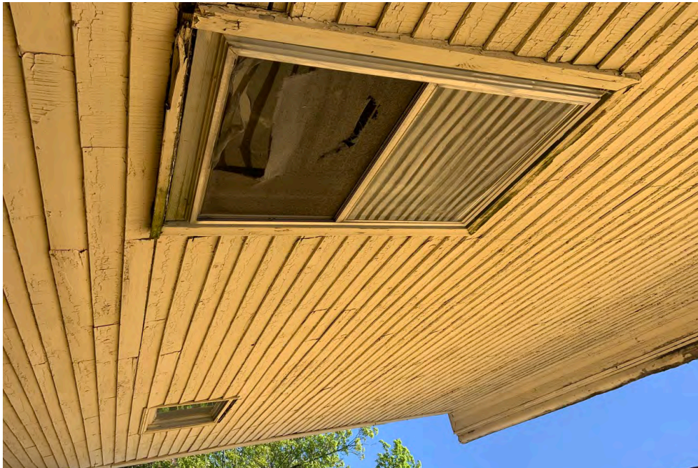
23 | East Elevation - main block - detail at northern end
