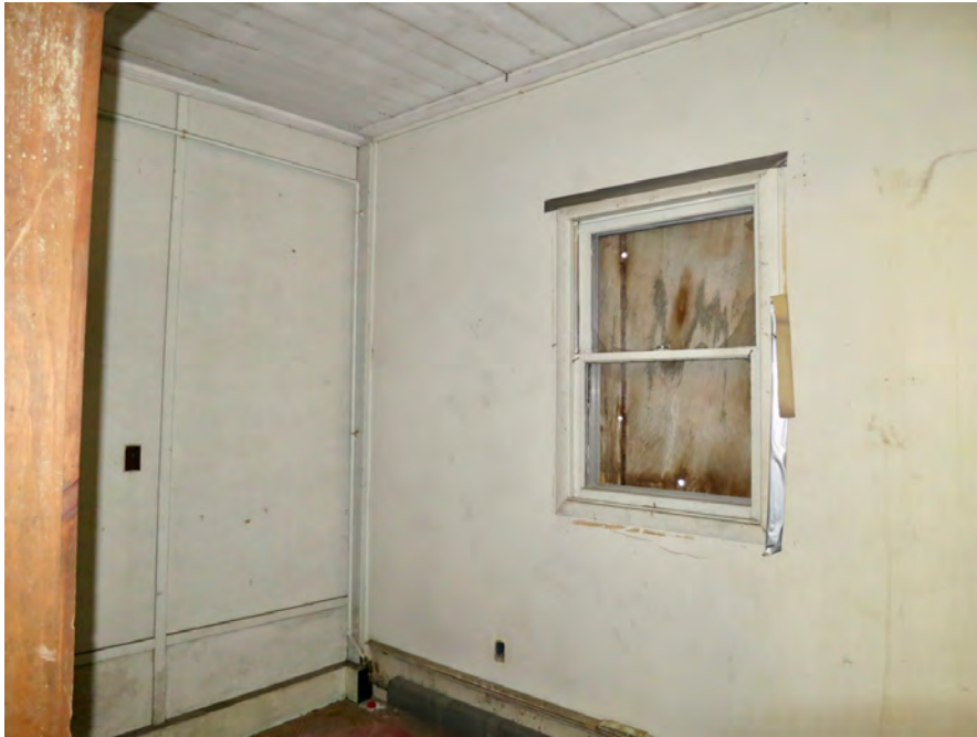
33 | First Floor - room in south corner of main block
