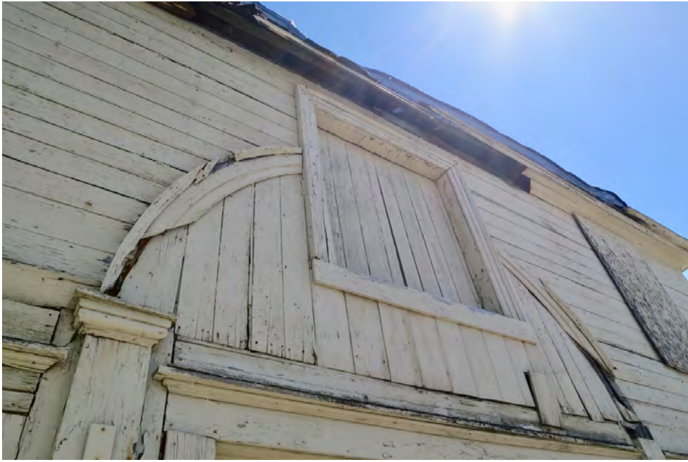
5 | West Elevation - detail of loading bay at second floor
