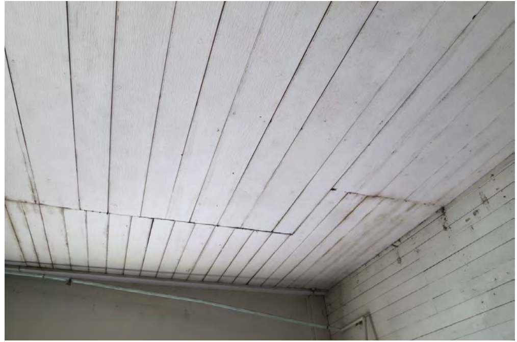
38 | First Floor - typical patched planking at ceiling
