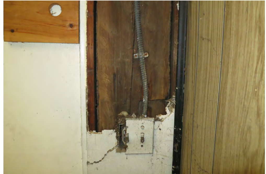
34 | First Floor - view of beam recovered with drywall (wood casing remains on sides)
