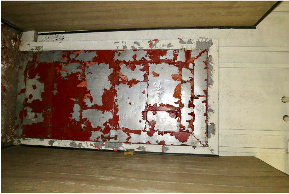
37 | First Floor - added fire door into addition
