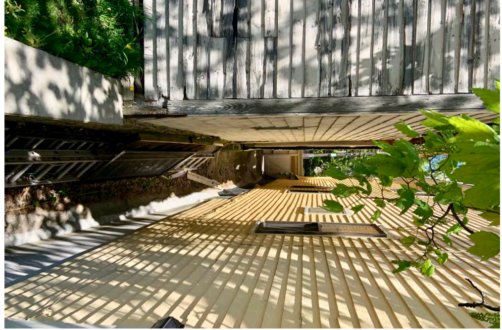
18 | View along alleyway between the carriage house (left) and neighboring house
