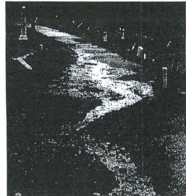
Erosion on southwest perimeter avenue
