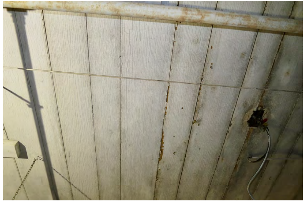
40 | First Floor - typical wood plank ceiling
