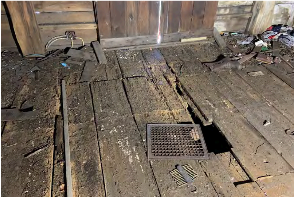
57 | Second Floor - detail of flooring in front of sliding loading doors
