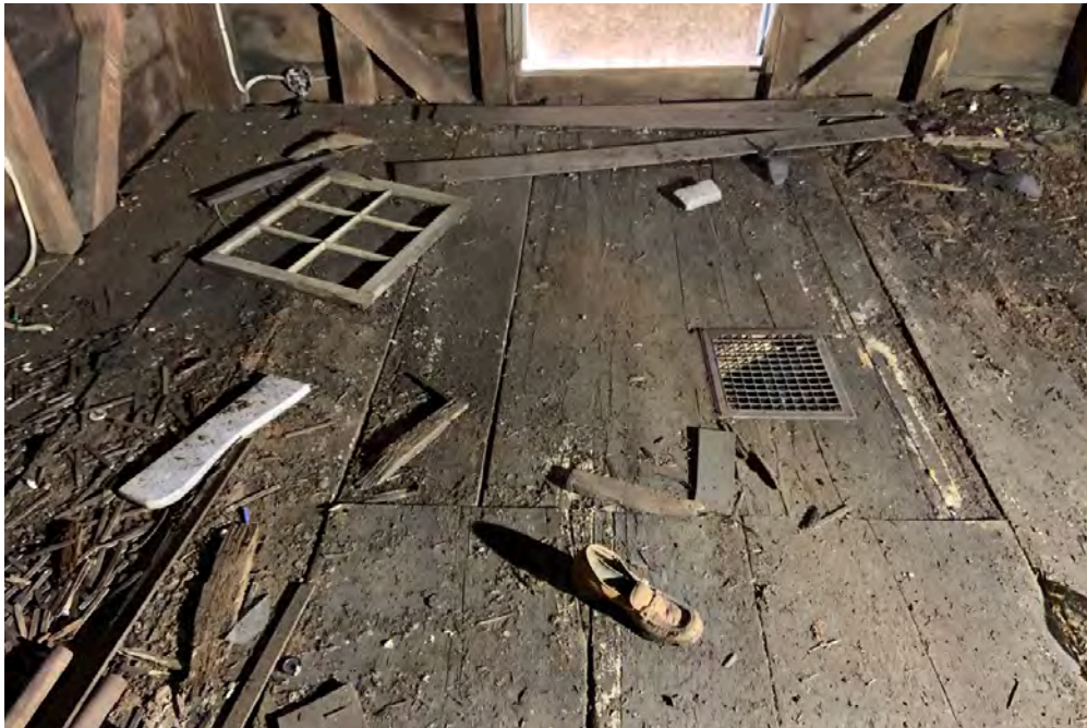
55 | Second Floor - detail of flooring in south corner
