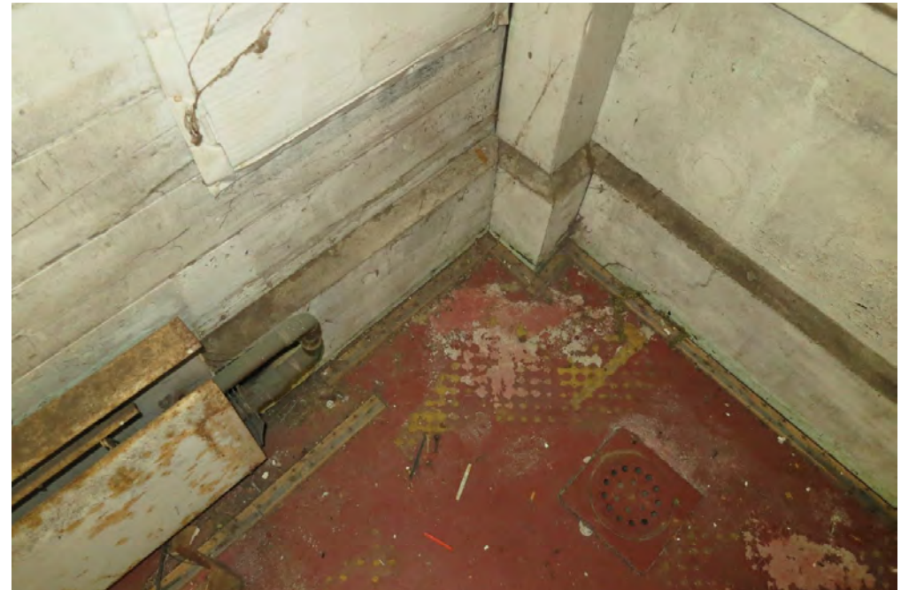
36 | First Floor - room in east corner of main block - detail of typical original baseboards
