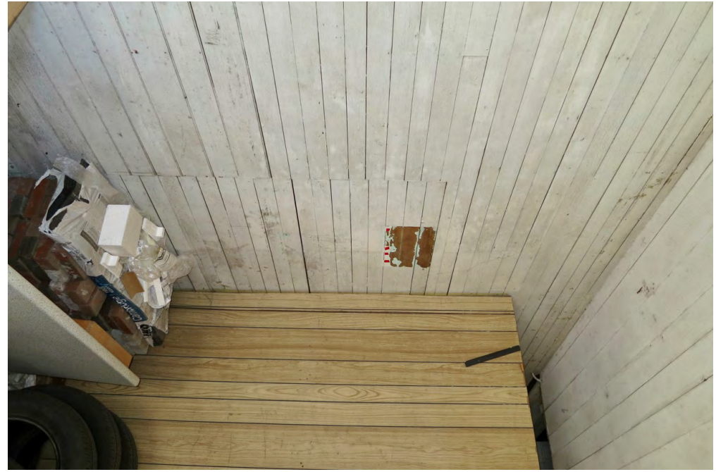
26 | First Floor - view along north wall showing infilled entry
