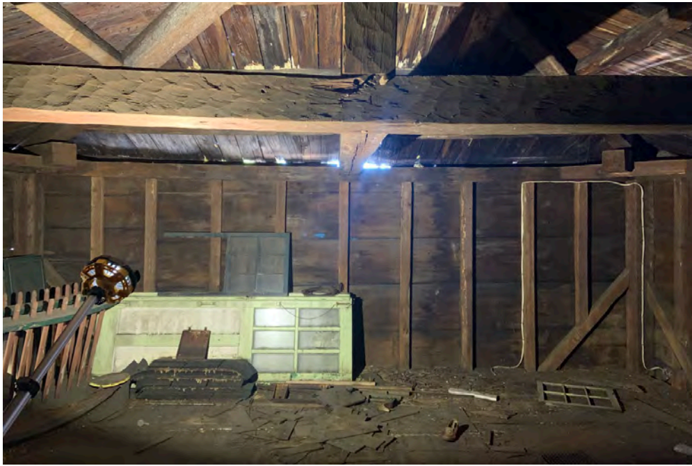
51 | Second Floor - view toward southeast wall
