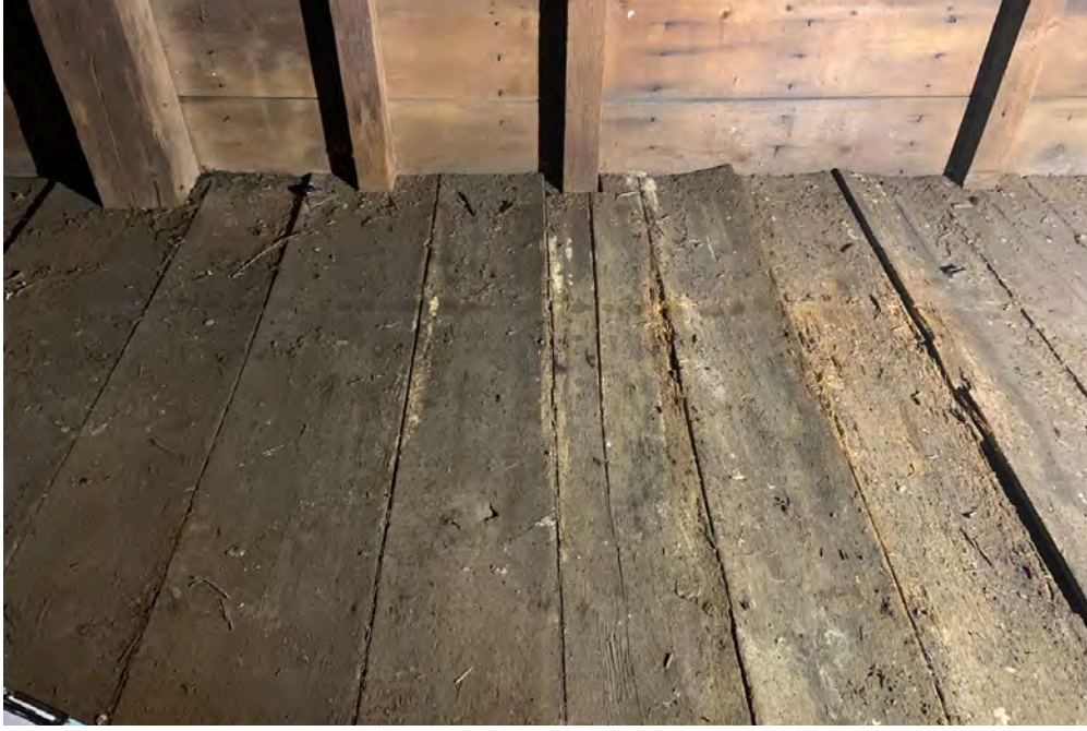
61 | Second Floor - detail of flooring along northeast wall
