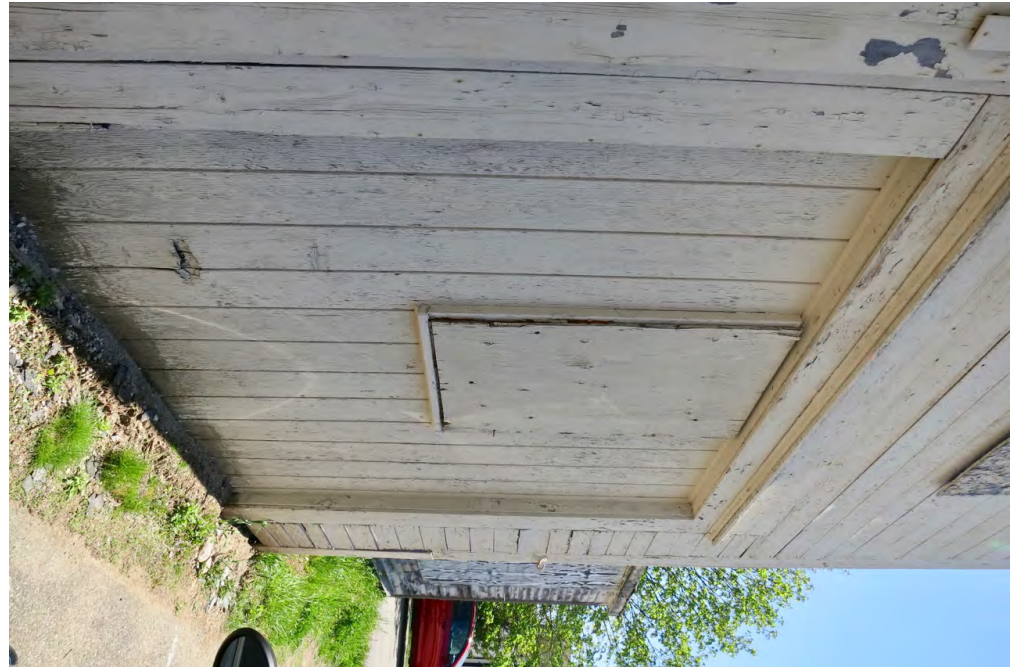
6 | West Elevation - added/infilled vehicle bay at south end
