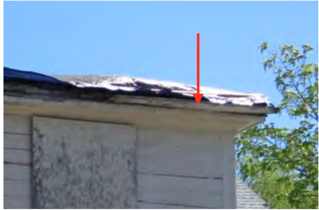
66 | West Elevation - detail at roof edge showing surviving section of wood gutter
