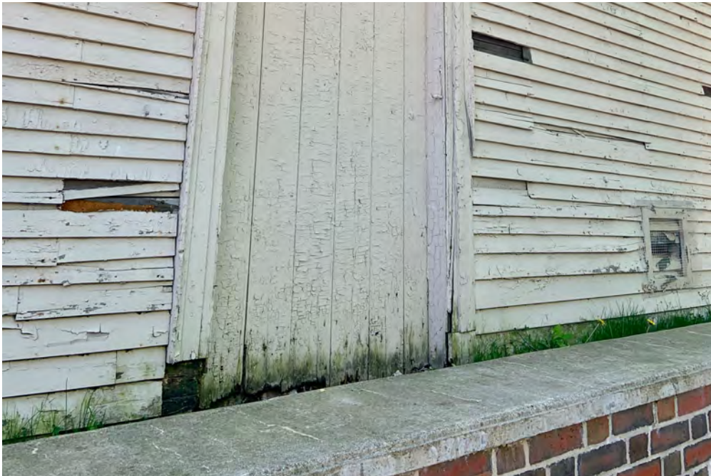
71 | Detail at base of north elevation
