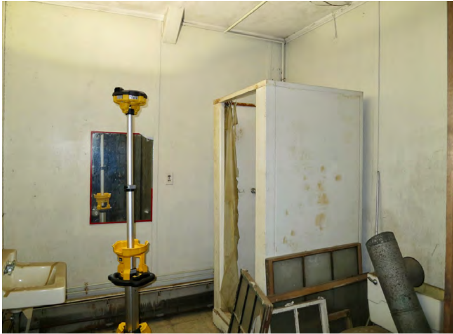
45 | First Floor - bathroom in addition
