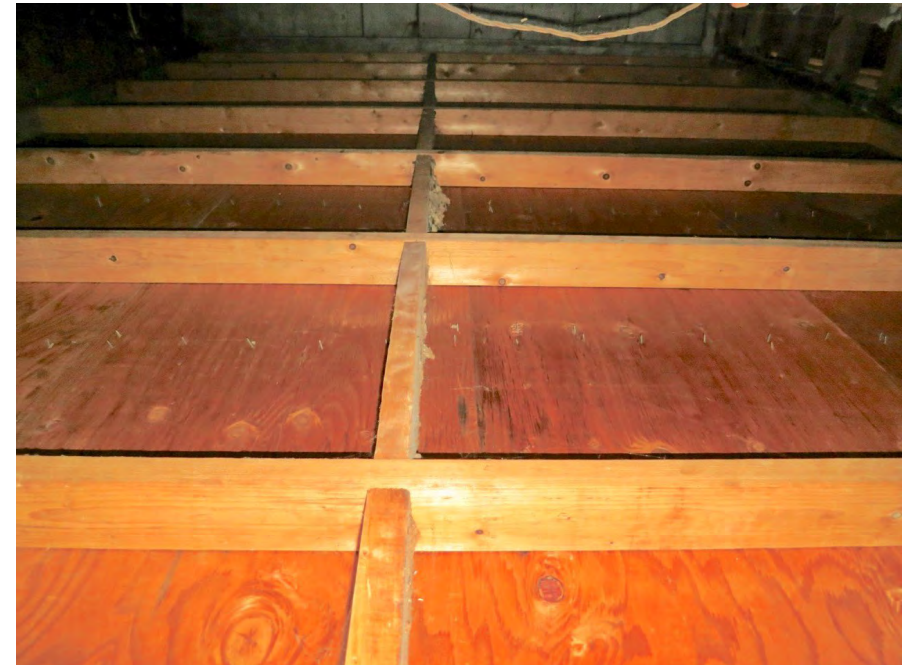
48 | First Floor - added stud wall enclosing southeast side of addition (built when connector to main house was demolished)
