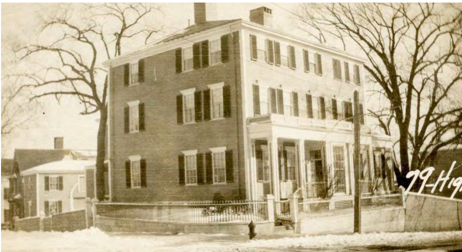
Figure 3: 1924 Tax Photo of 71-79 High Street showing the carriage house at 100 Pleasant Street in the rear at left.
