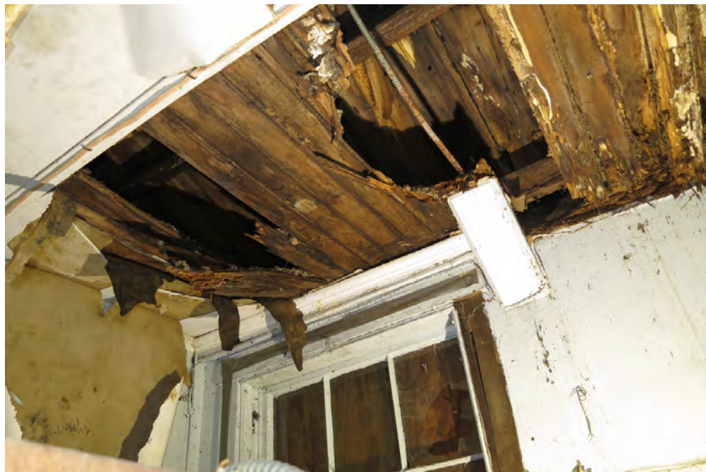
44 | First Floor - view of original ceiling in addition entry hall
