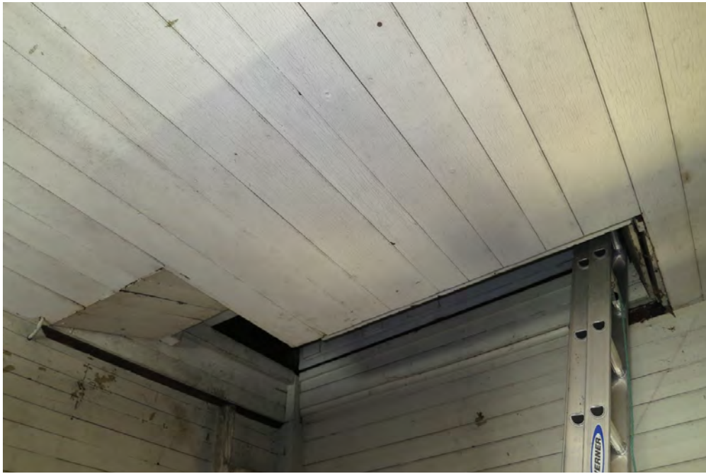
39 | First Floor - detail at access hatch to second floor
