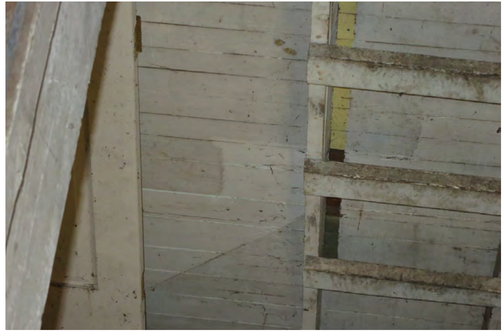
28 | First Floor - view in northeast corner showing shadow of old staircase
