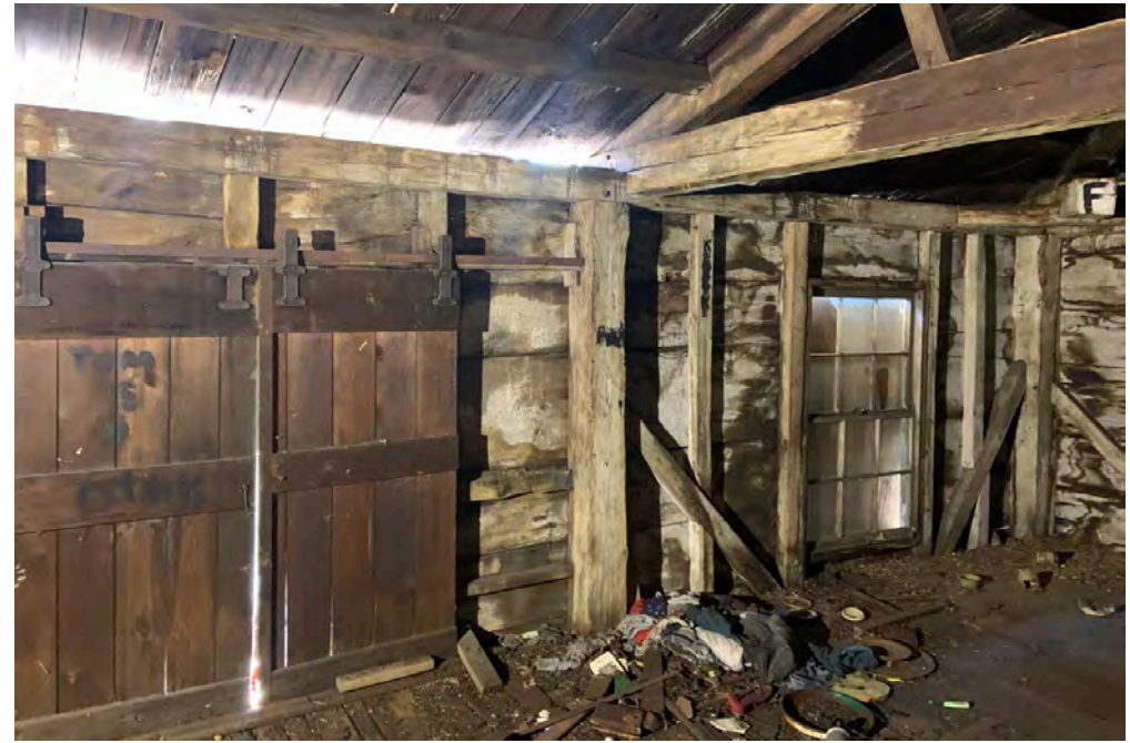
52 | Second Floor - view along southwest wall
