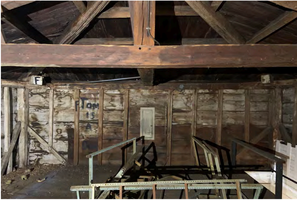
49 | Second Floor - view toward northeast wall
