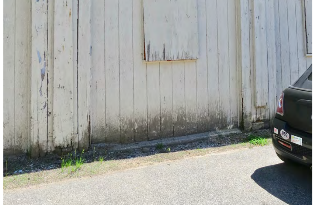
74 | Detail at base of west elevation - at center
