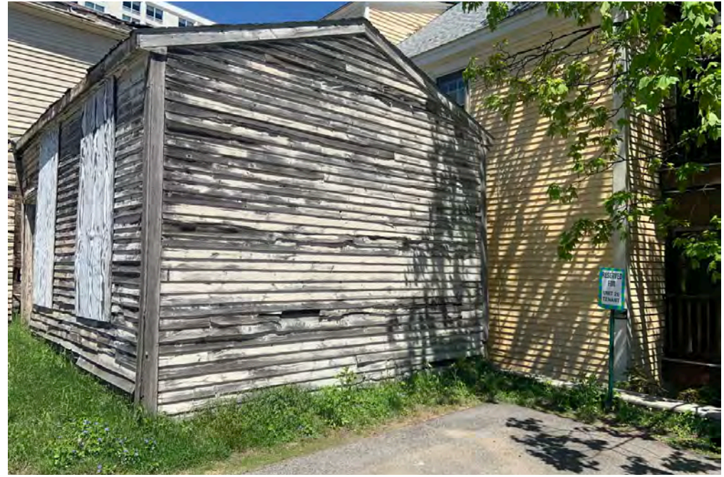
14 | South Elevation - addition
