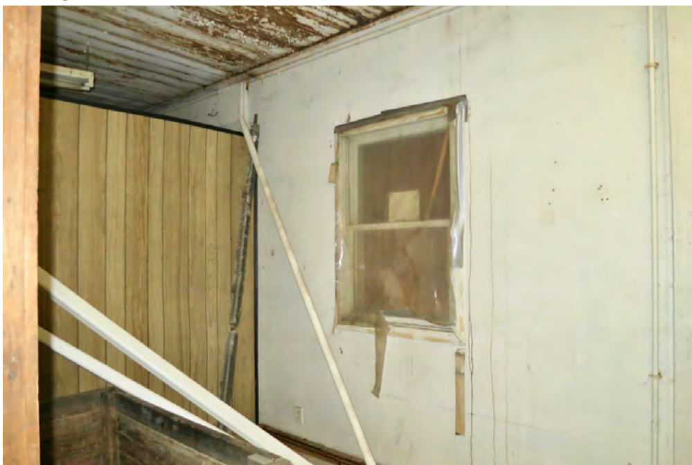
31 | First Floor - central room along southwest wall
