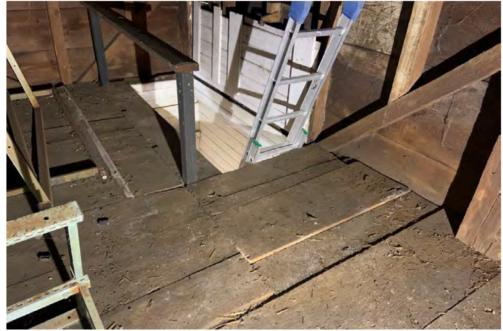
50 | Second Floor - view toward hatch to first floor
