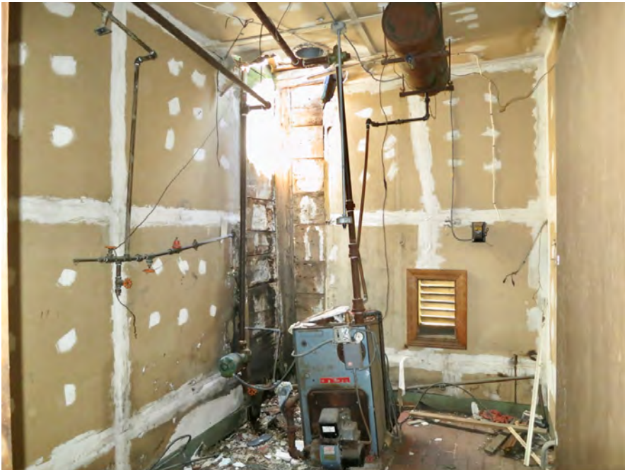
47 | First Floor - mechanical room in addition
