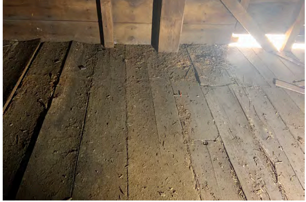
62 | Second Floor - detail of flooring along northeast wall
