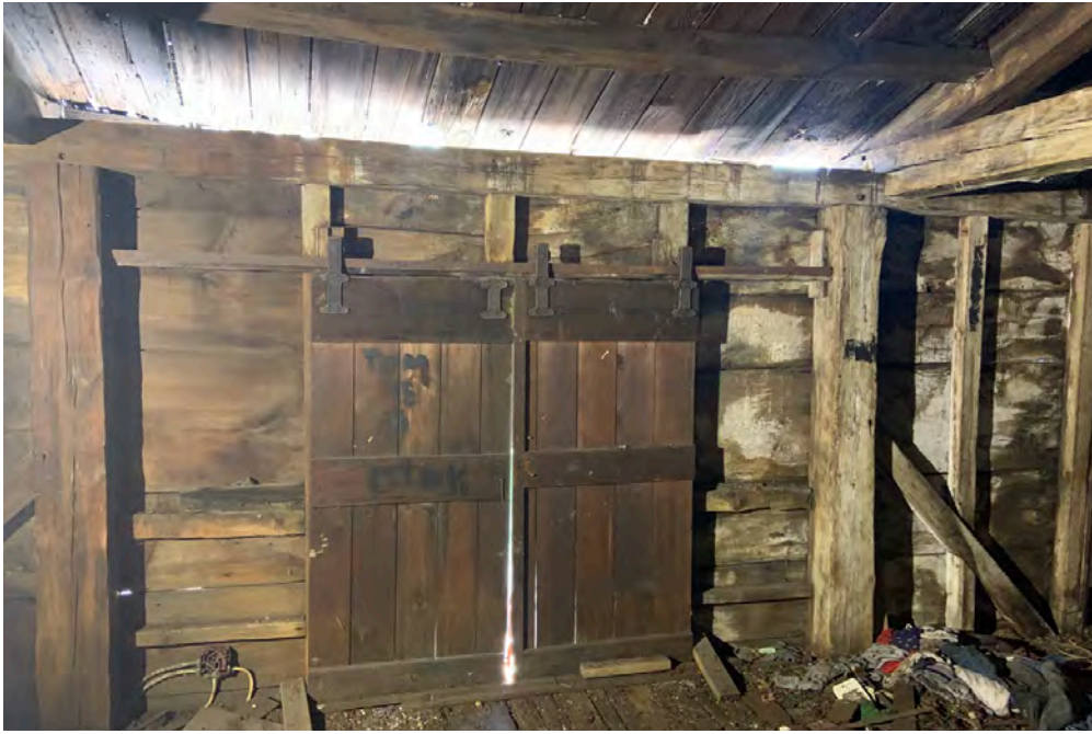
53 | Second Floor - sliding loading doors at center of southwest wall
