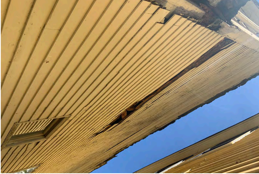
21 | East Elevation - main block - detail at southern end
