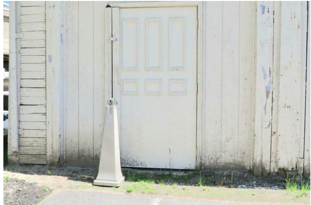
72 | Detail at base of west elevation - north end
