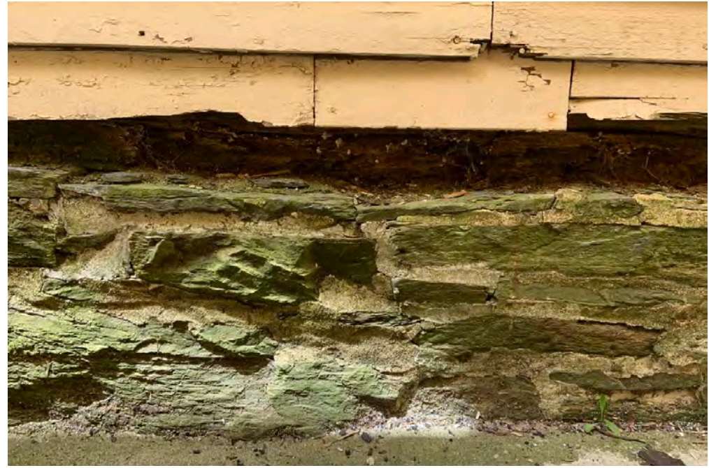
70 | Detail of stone foundation at east elevation
