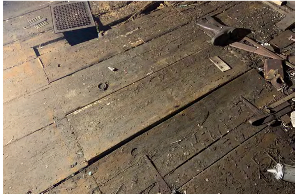
58 | Second Floor - hatch in floor near loading door
