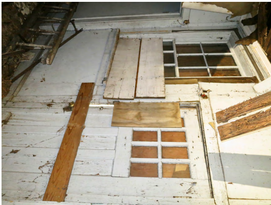
43 | First Floor - exterior entry to addition
