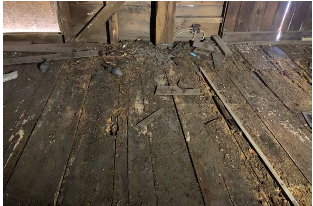
56 | Second Floor - detail of flooring along southwest side
