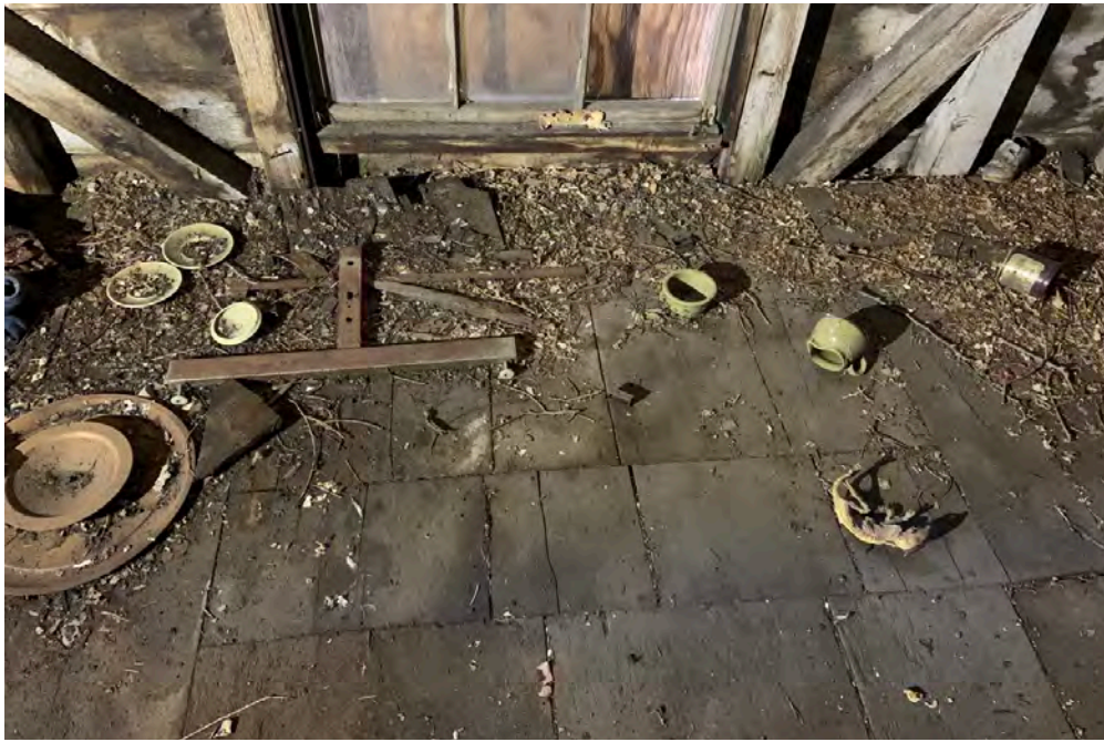
59 | Second Floor - detail of flooring near west corner
