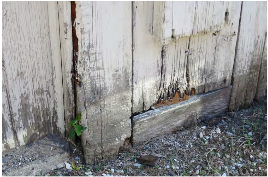
8 | West Elevation - detail at base of pilaster in central carriage bay
