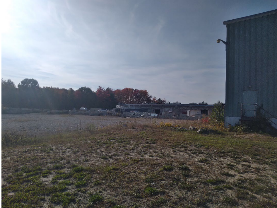
Figure 3. Facing west, looking at old foundation and site of new warehouse.
