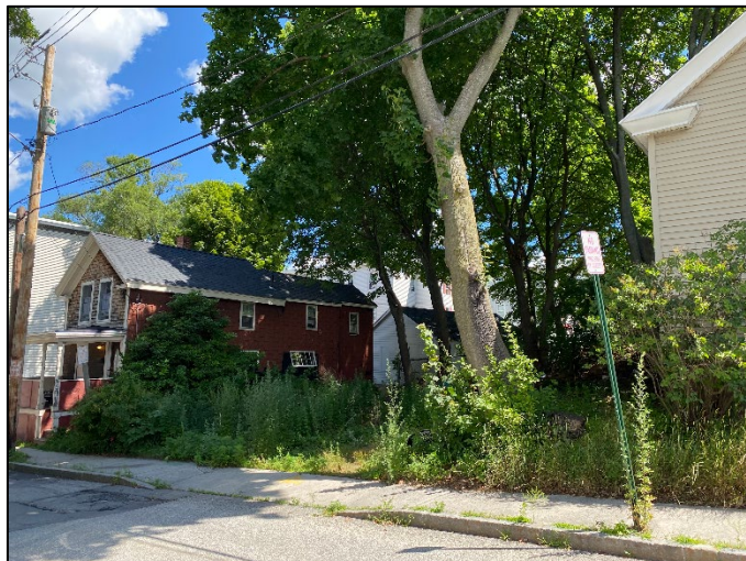
Figure 2. 31 Forest Street, Existing Conditions
