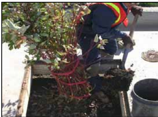
3. Removal of debris, trash and mulch
