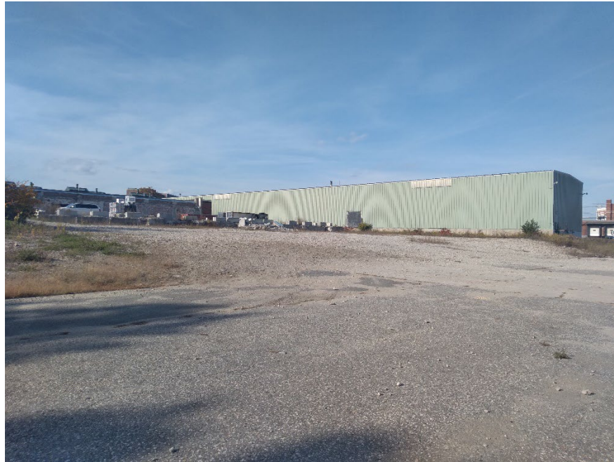
Figure 1. Existing 182 Read Street and site of new warehouse, facing north
