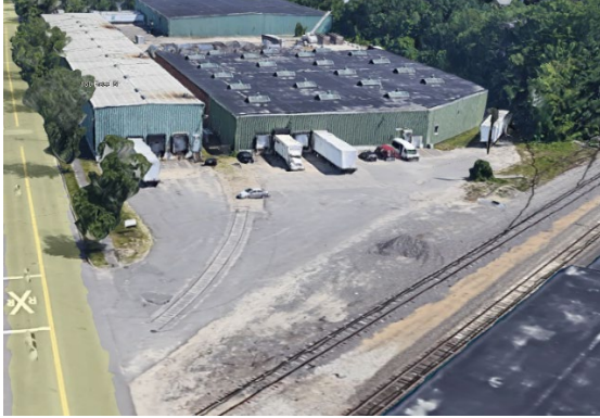
Image 3. Google Earth view of 180 Read from the northwest.
