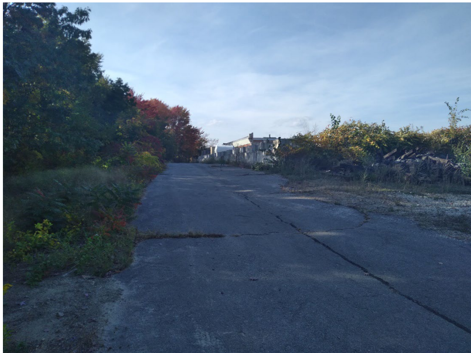
Figure 4. Existing paved drive, not in use, facing northwest.
