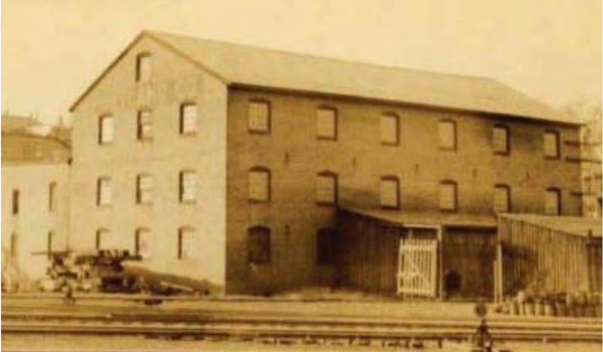
Figure 4: Undated photograph of Building 12 with Building 11 to the back left, and a lean-to addition at the south elevation, generally in the location of the mechanical enclosure and patio structure.
