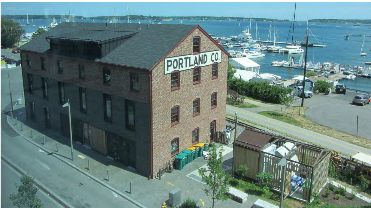
Figure 3: 2022 view of the relocated Building 12 looking southeast from inside the newly constructed office building at 110 Thames Street. Note the dark gray brick infill and modern windows at the north elevation where Building 11 had originally been connected to Building 12 (Historic Preservation Staff)
