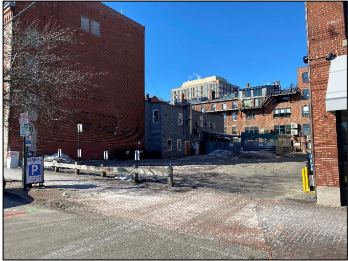
Figure 2. 185 Commercial Street, Existing Conditions
