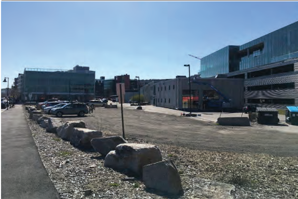
Subject property site with new WEX office building and parking garage complex in the background
