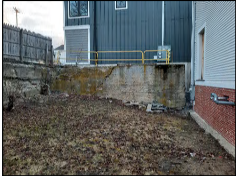
13. REAR VIEW Looking West
