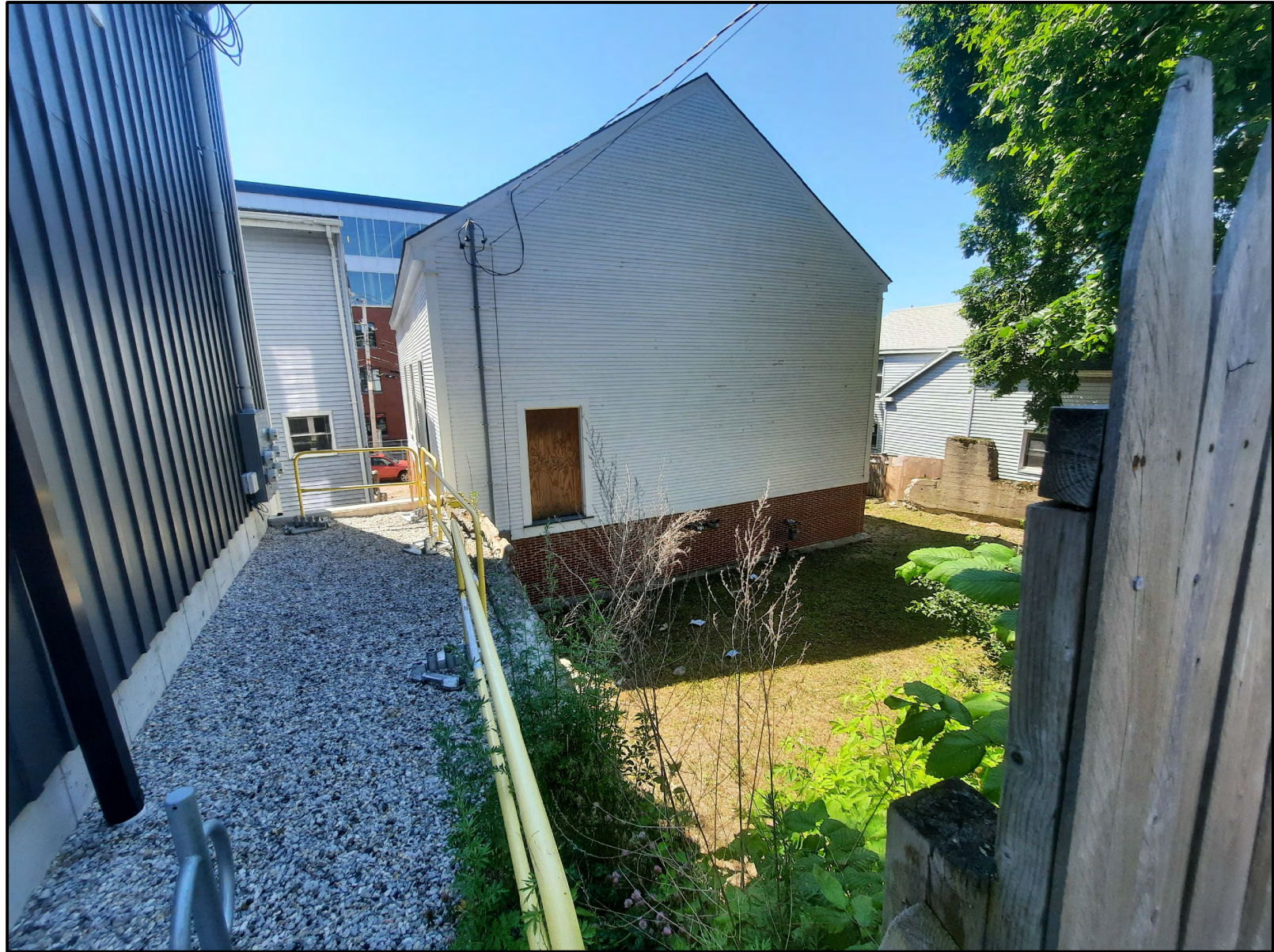
10. VIEW FROM FEDERAL STREET SIDEWALK
