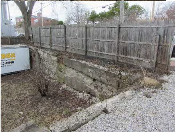
Figure 6: Existing Conditions (rear,) 2/16/2023
