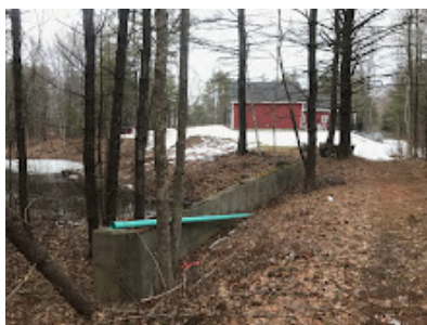
Concrete Bridge to Haverly Way.JPG 4088K
