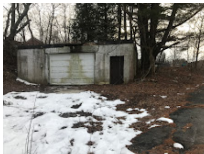
Haverity Field - Abandoned Garage Building.JPG 3808K
