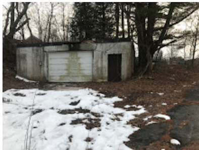
Haverly Field - Abandoned Garage Building.JPG 3808K
