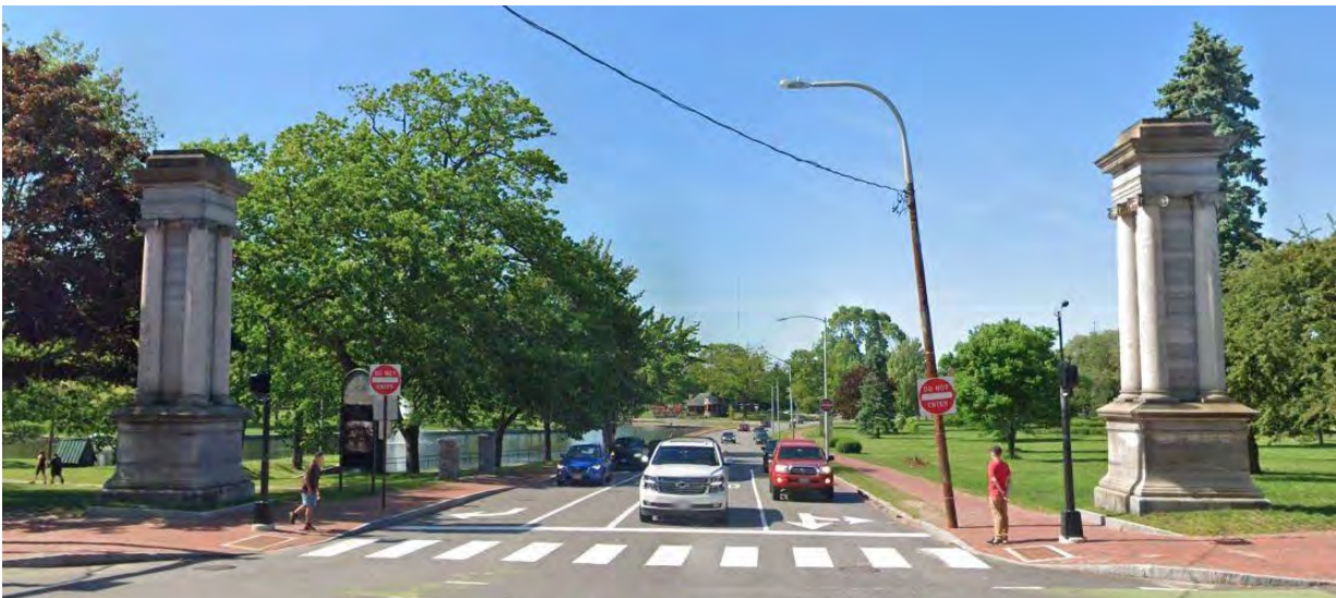
Figure 3: 2019 view of the State Street piers in their present condition without the original lights. (Google Earth)
