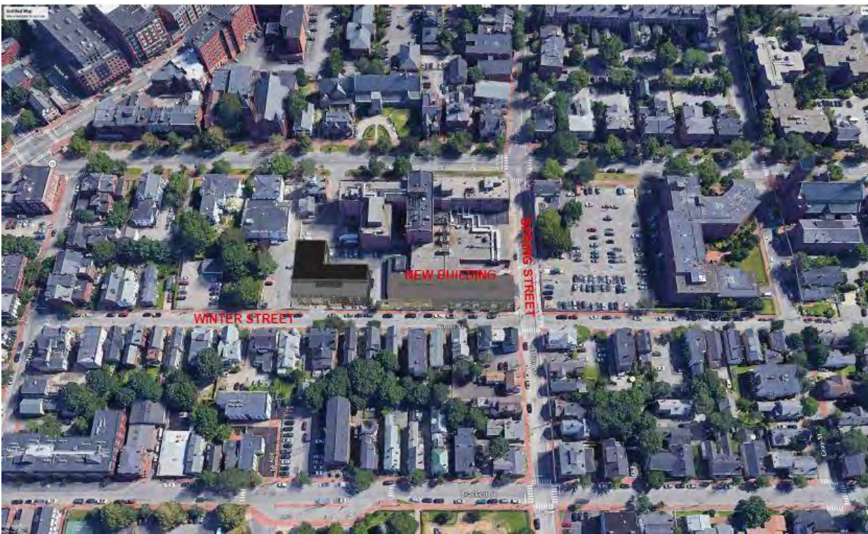
Figure 1: Aerial view of the Mercy complex and the context, showing location of 73 Winter Street.
