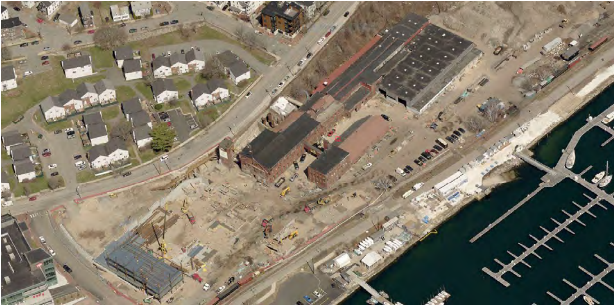
Figure 4: 2021 aerial view of the Portland Company site showing Block 1 under construction at the western edge of the site (bottom left).
