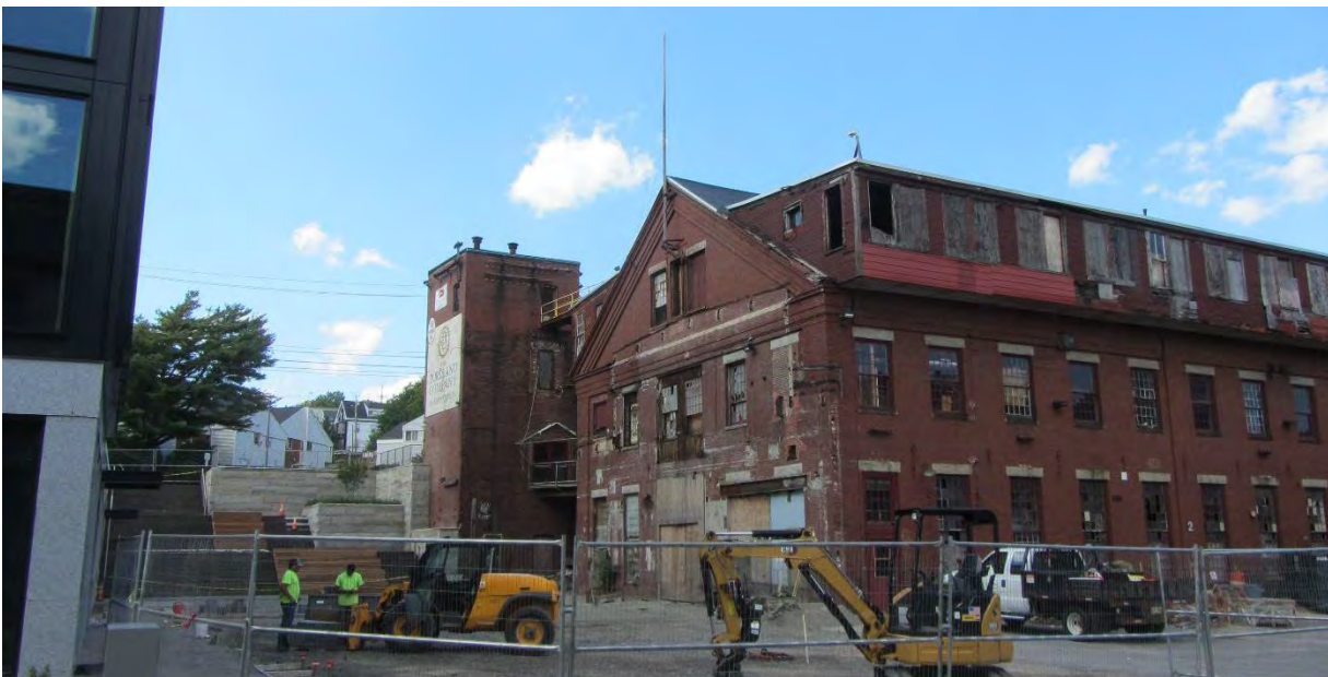
Figure 6: 2022 view of the Buildings 2 & 24. Block 1, at left, was nearing completion with sitework being completed in the foreground.
