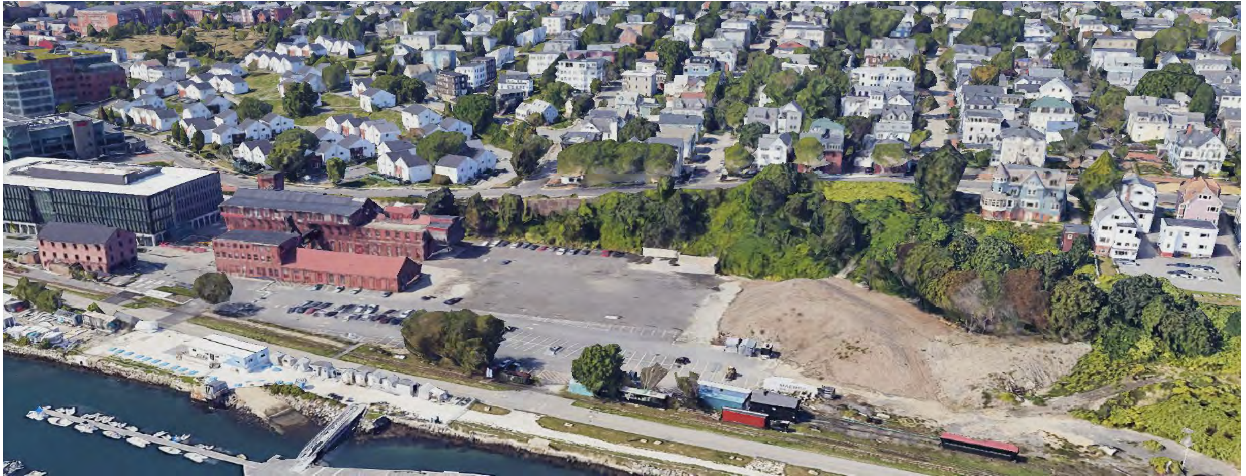
Overall site looking North
