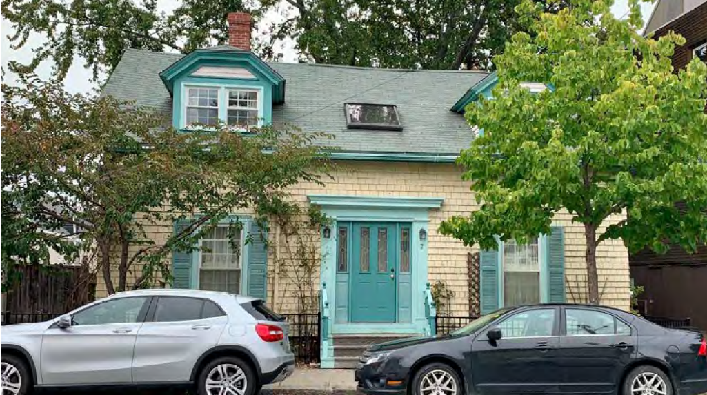
Figure 4: An example of an early, though somewhat altered, cape type house, which would have been common in the early- to mid-nineteenth century (7 Lafayette Street).
