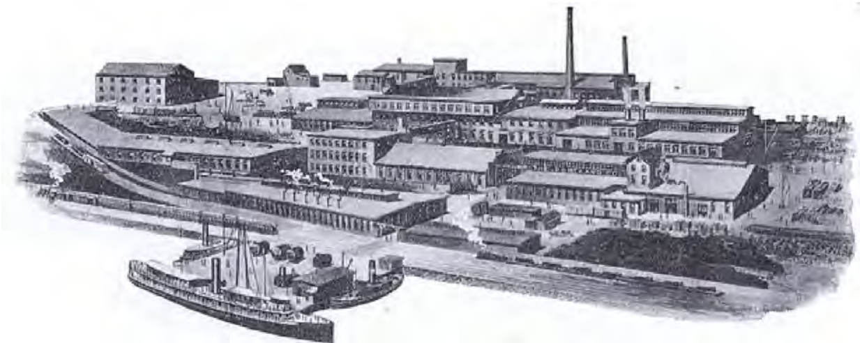
Figure 3: 1920 sketch image of the Portland Company site showing the scale of the sprawling complex. (Maine Preservation Commission)
