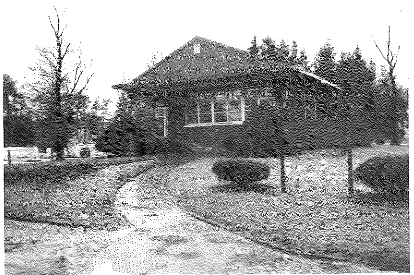
The present office building is functional but lacks the historic integrity of the original structure.
