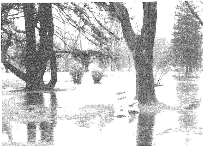
Because of the lack of a comprehensive drainage system throughout Evergreen, there is a great deal of uncontrolled water in the cemetery.
