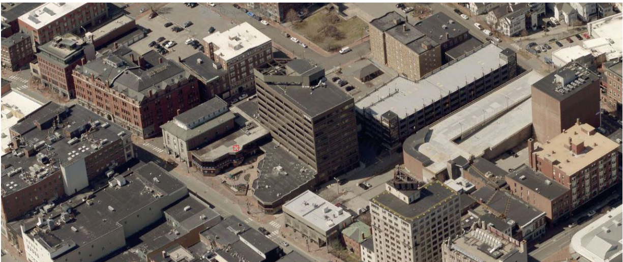
Figure 2: Aerial view of 511 Congress Street, looking north.
