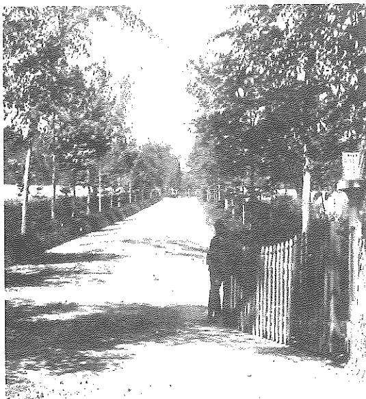
The original entrance created a ceremonial experience with focused views into the cemetery.
