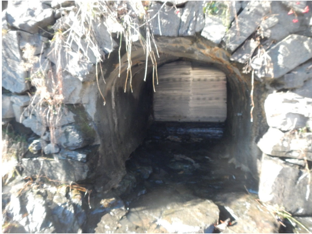
Photo 29: Sluiceway, following closure of Aluminum Slide Gate
