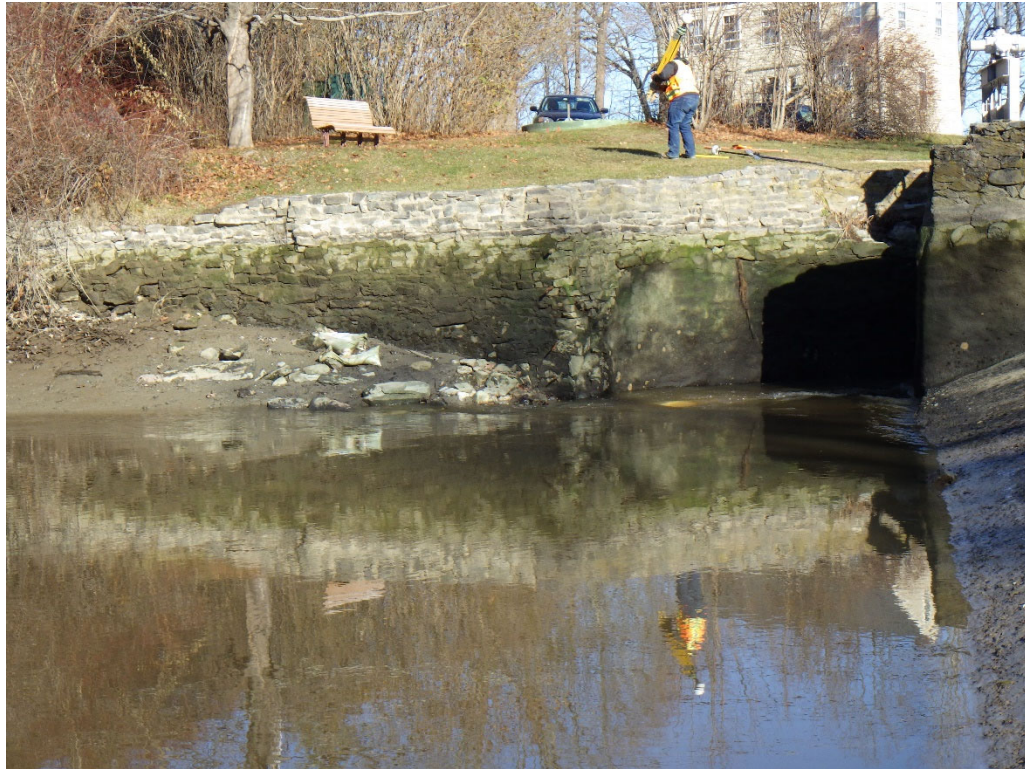
Photo 17: Left abutment training wall
