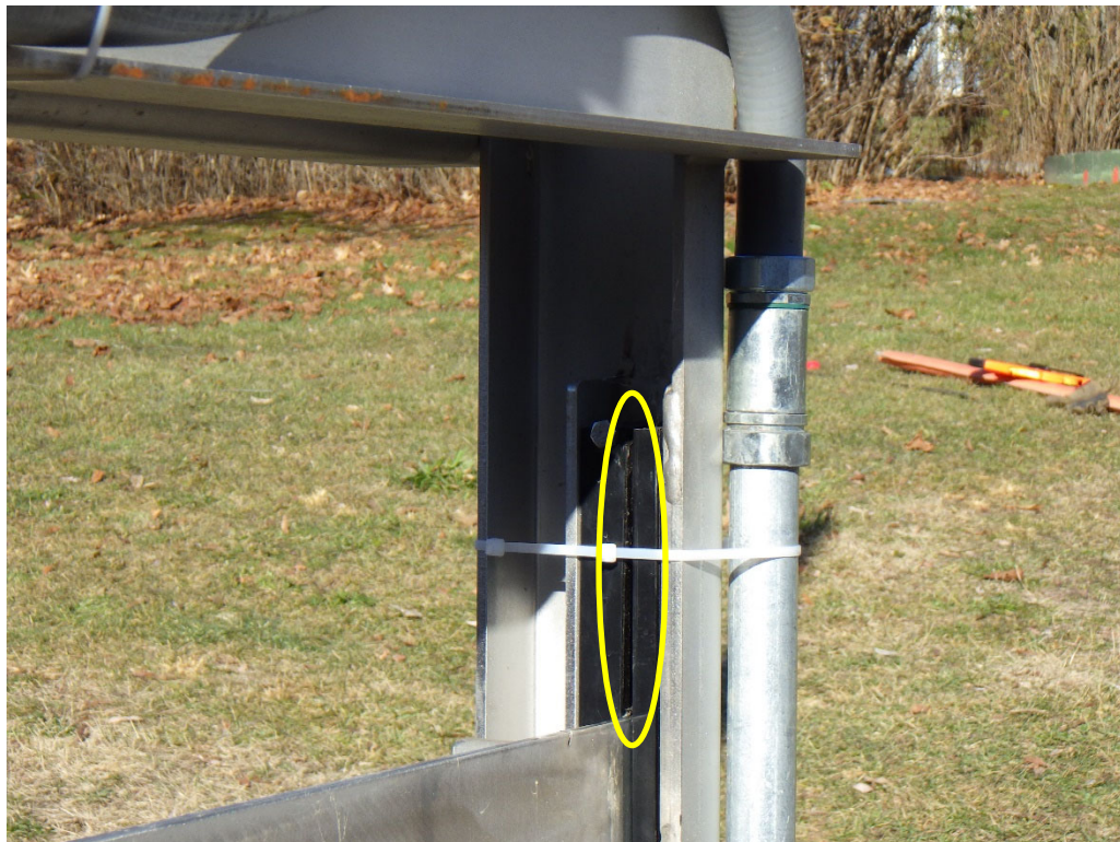
Photo 16: Guide strip slot clearance of Aluminum Slide Gate
