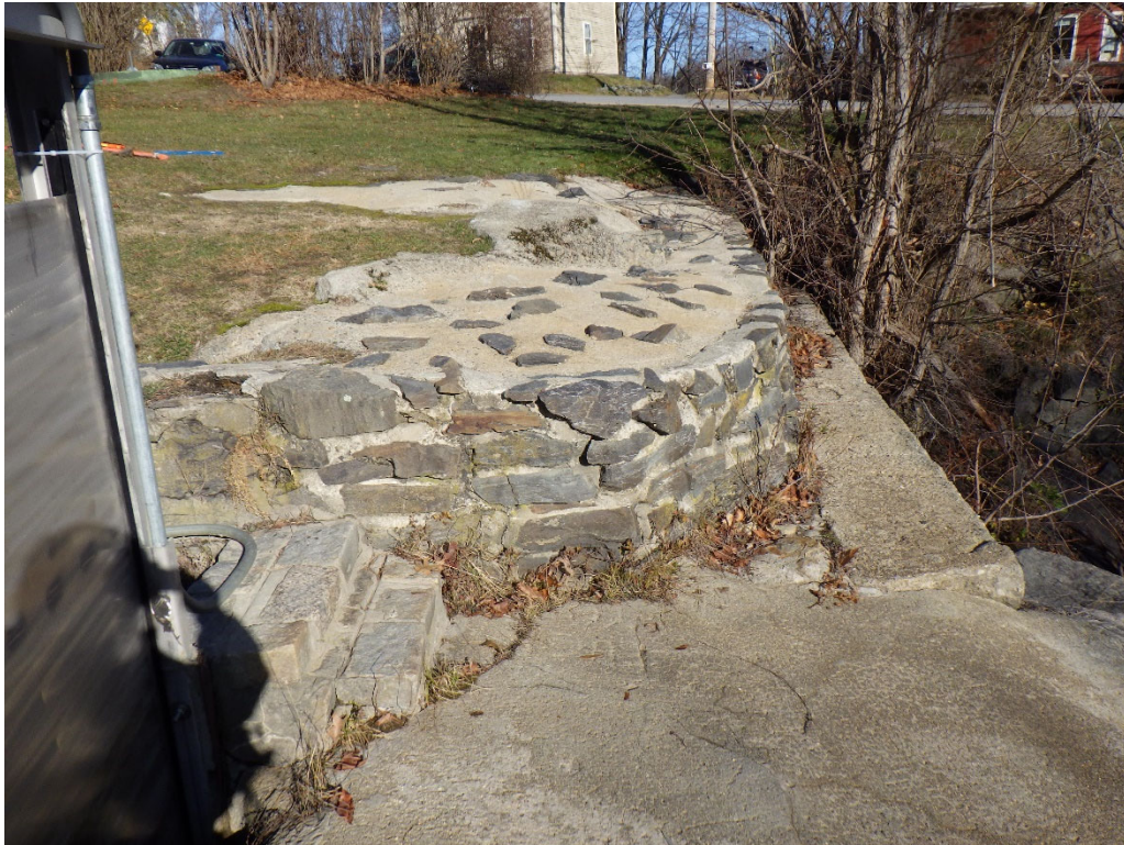
Photo 25: Concrete fill in historic low part of dam crest (downstream edge of Left Abutment)
