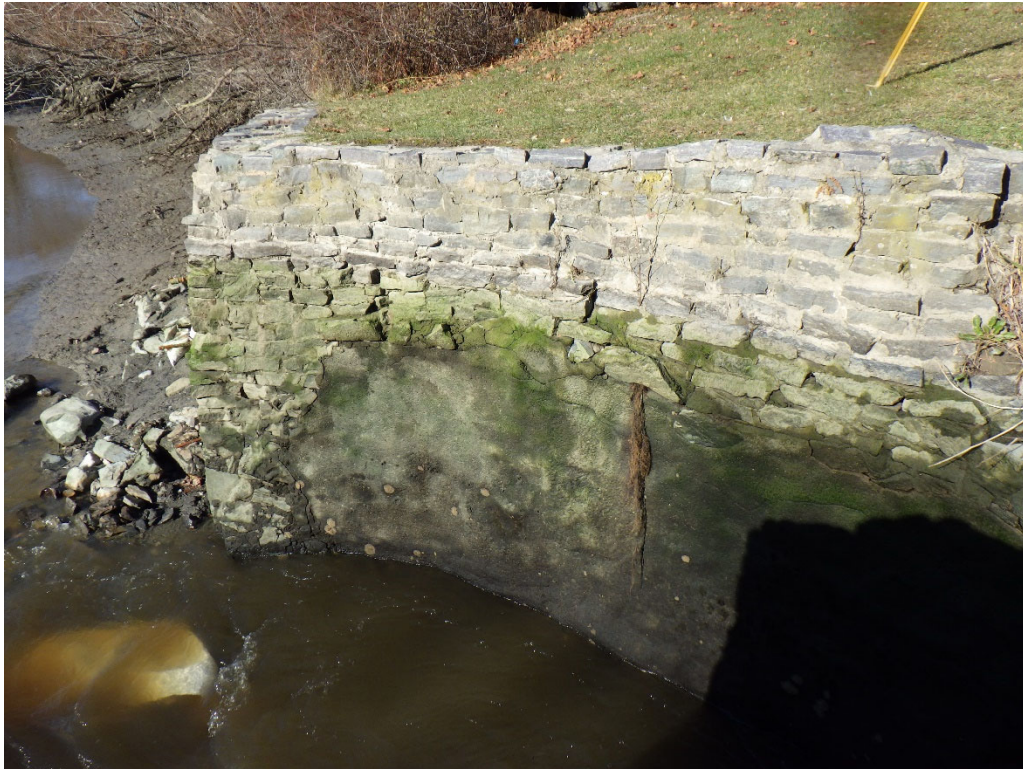
Photo 19: Upstream end of low-level outlet approach / upstream corner of left abutment training wall
