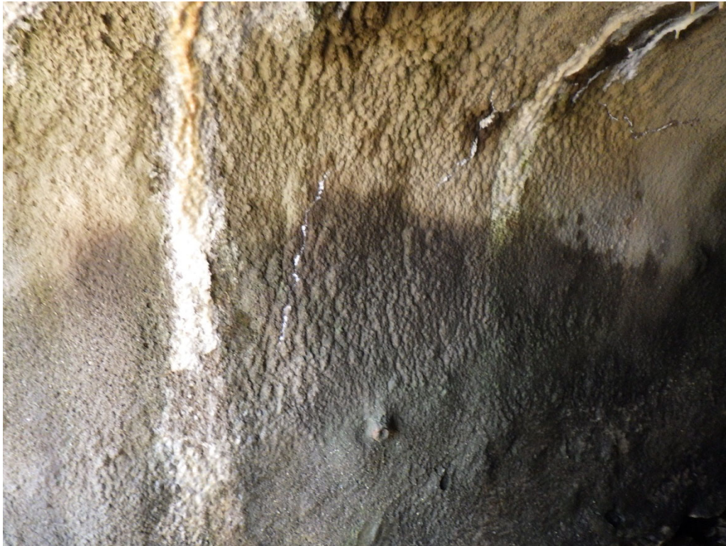
Photo 31: Condition of shotcrete overlay of Sluiceway left side
