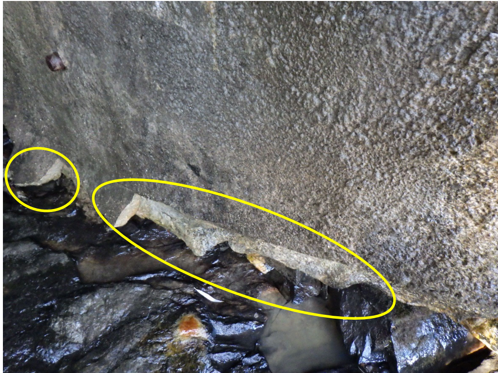
Photo 33: Interface between bedrock foundation and shotcrete overlay of Sluiceway
