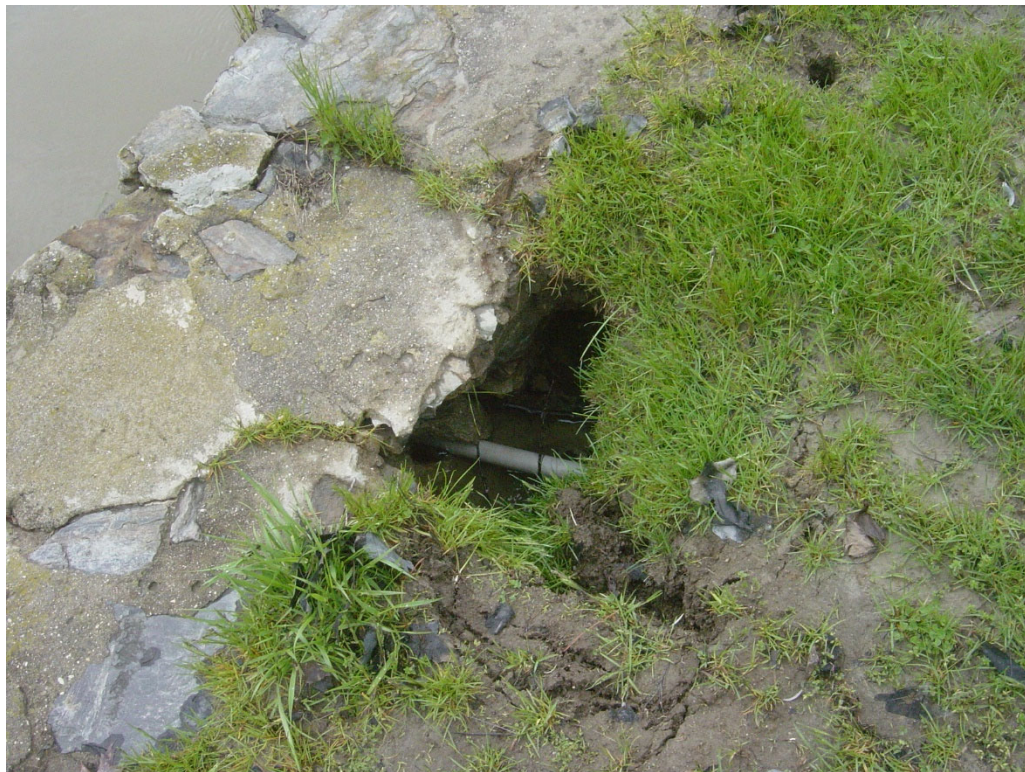
[Historic] Photo 22: Left Abutment sinkhole on May 16, 2006 (subsequently filled)
