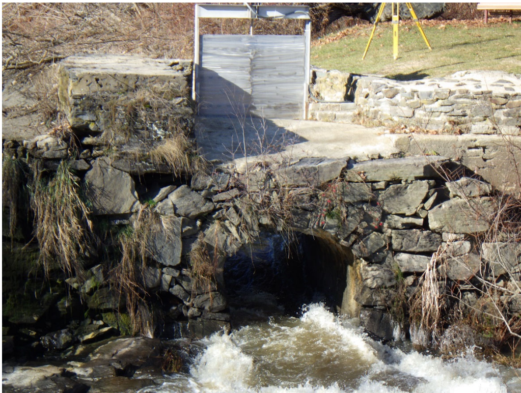
Photo 28: Sluiceway outlet at time of inspection
