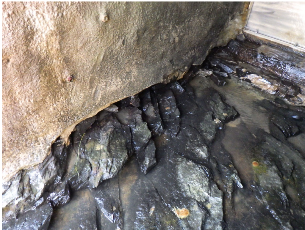
Photo 36: Interface between bedrock foundation and shotcrete overlay on right side of Sluiceway
