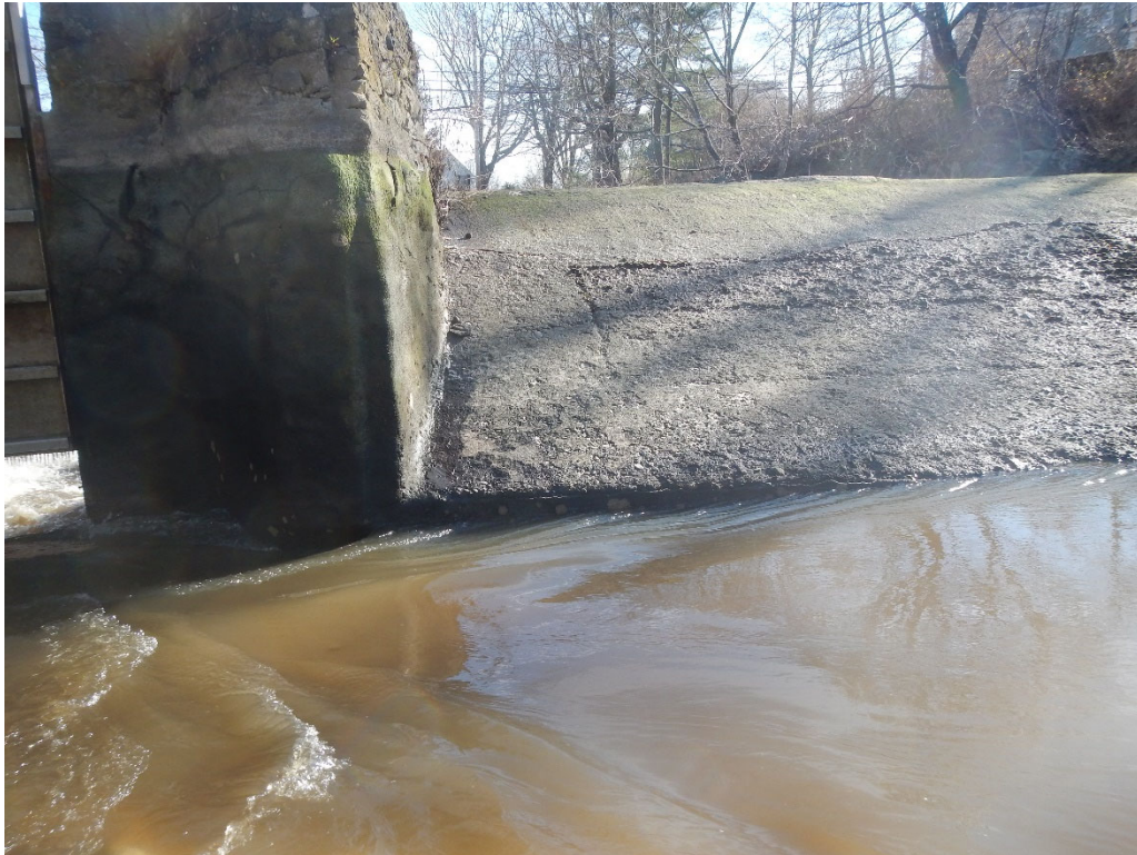
Photo 13: Divider pier and interface with upstream face of Primary Spillway
