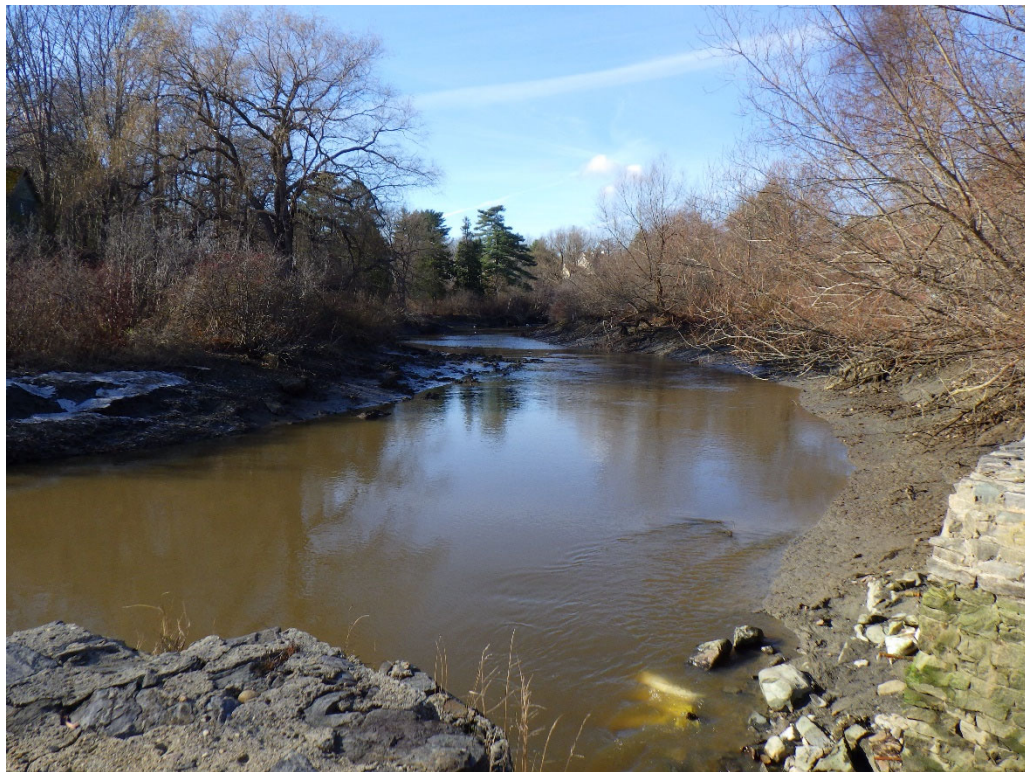
Photo 2: Reservoir at time of inspection (looking upstream from dam)
