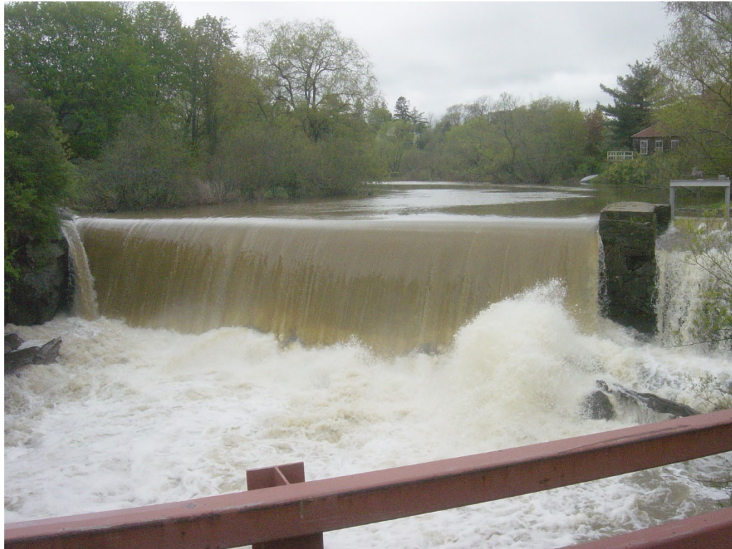
[Historic] Photo 3: Dam spillage on May 15, 2006 (Mother's Day Flood) – NOTE overflow of former steel slide gate acting as a sort of secondary spillway
