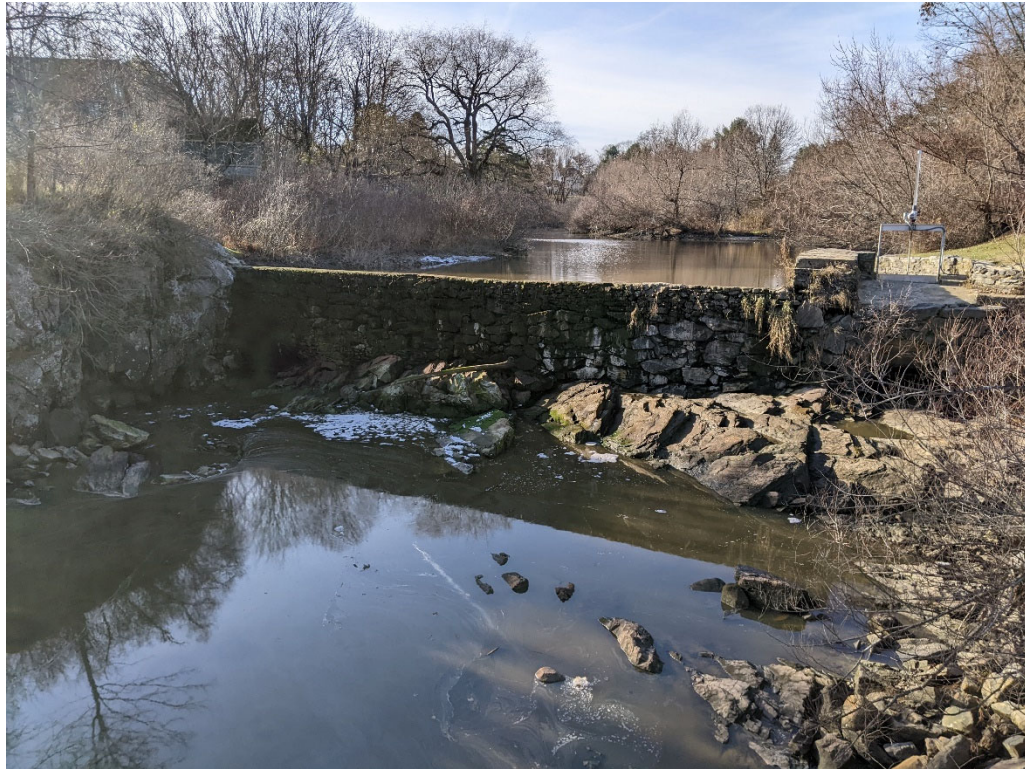
Photo 1: Downstream face of Stroudwater Dam from Westbrook Street Bridge (looking upstream)
