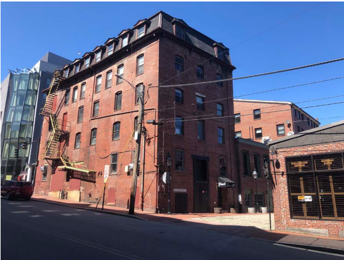
Photo 3 446 Fore Street Before Rehab. Corner of Union Avenue and Wharf Street.
