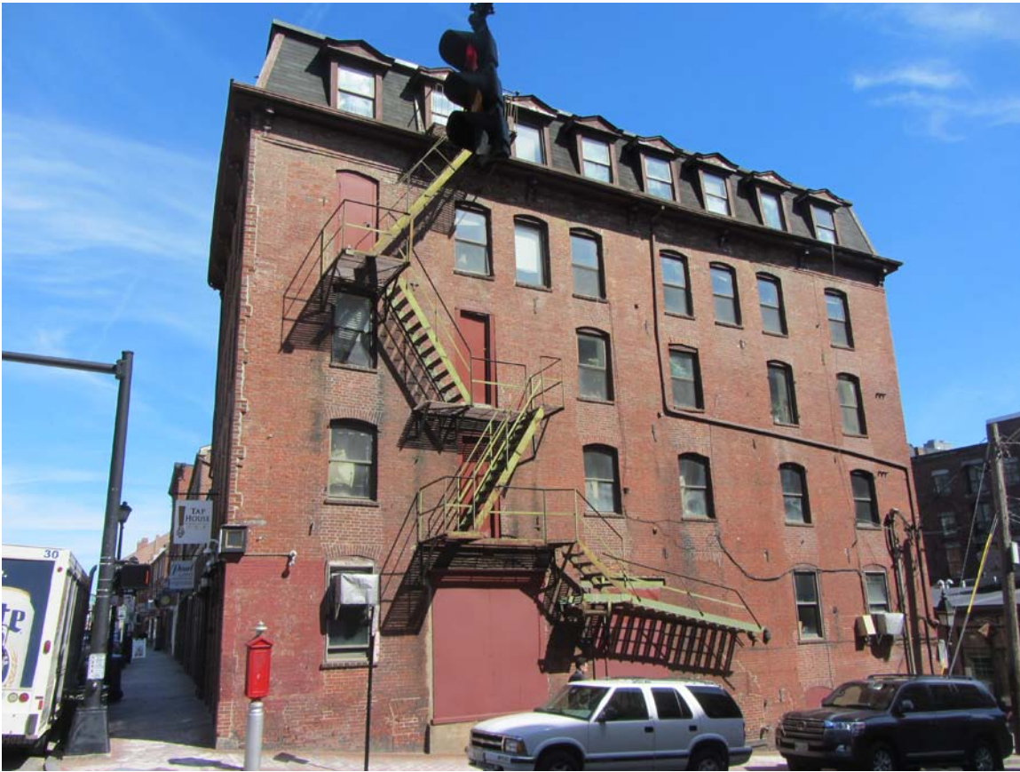
Photo 2 446 Fore Street Before Rehab. Union Avenue Elevation.
