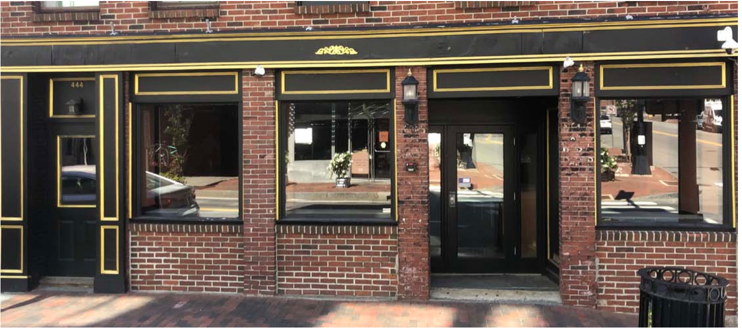
Photo 7 Primary Front Entry Recessed entry of 1st floor commercial space. Recessed entry constructed sometime after 1981. Before Rehab. Fall 2022
