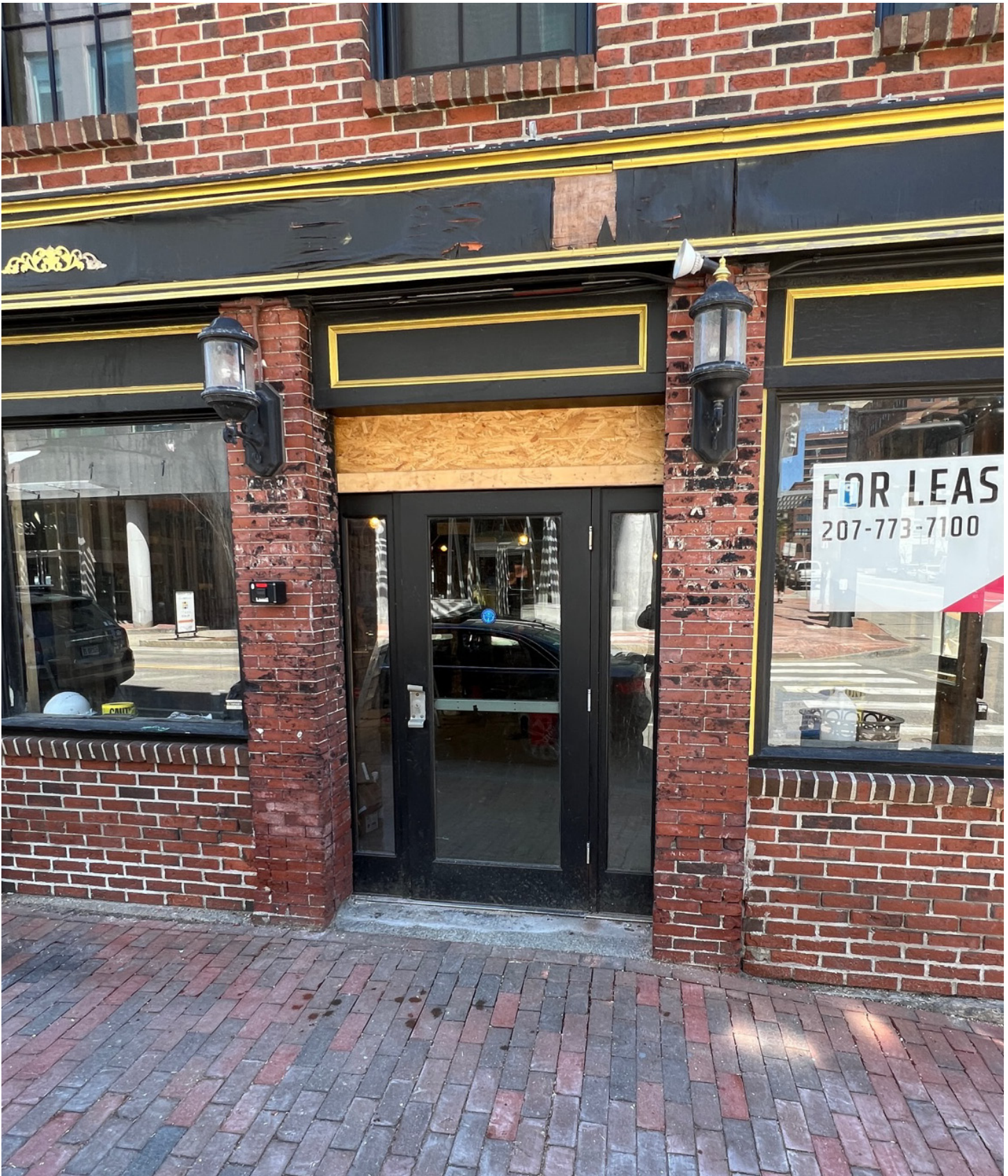
Photo 9 Primary Front Entry Existing door temporarily installed as street place for closure
