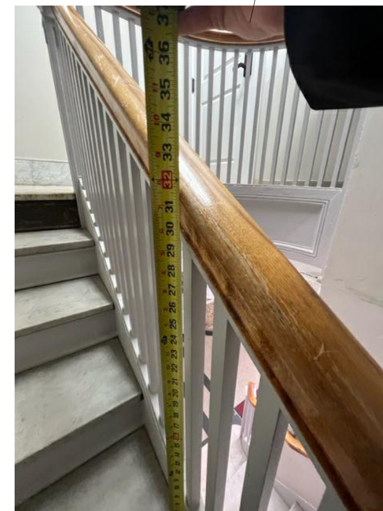
EXISTING GUARDRAIL ON STAIR 1B
