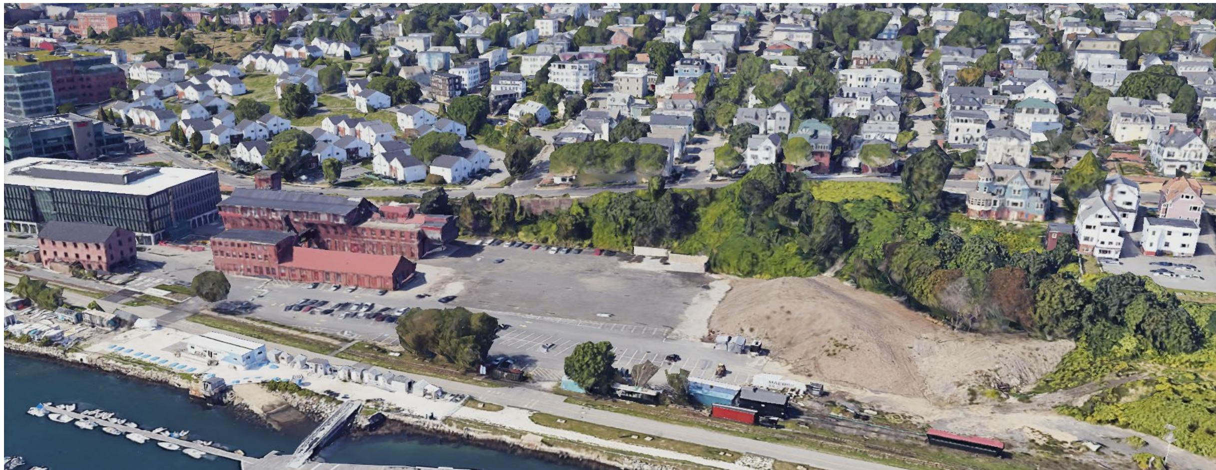
Overall site looking North
