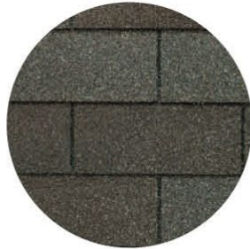
Three-Tab Asphalt Shingle Pitched Roof
