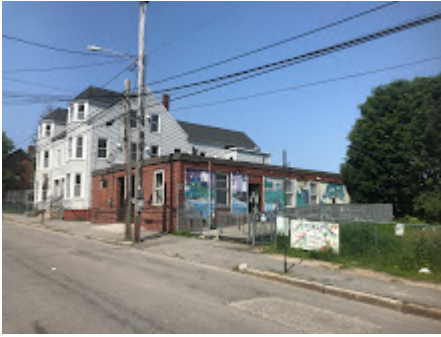
Empty-Mothballed Oxford Street Shelter - Looking West.JPG 3082K
