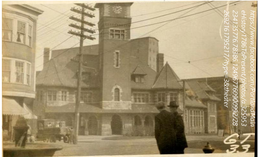
Grand Trunk Station at Fore & India
