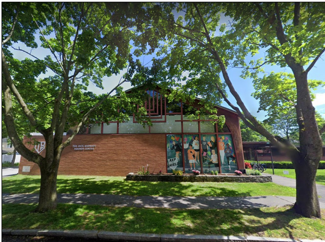
Figure 1: Existing Portland Community Squash Building Located at 76 Noyes Street
