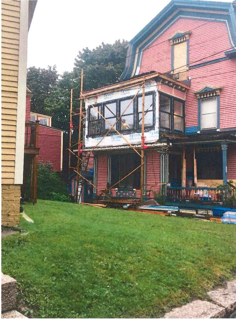
Taken from directly across Mellen Street with an angle that reveals the most of the visible south aspect
