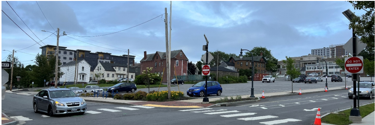
Figure 3: Photo of the project site looking northeast at the intersection of Elm & Lancaster Street
