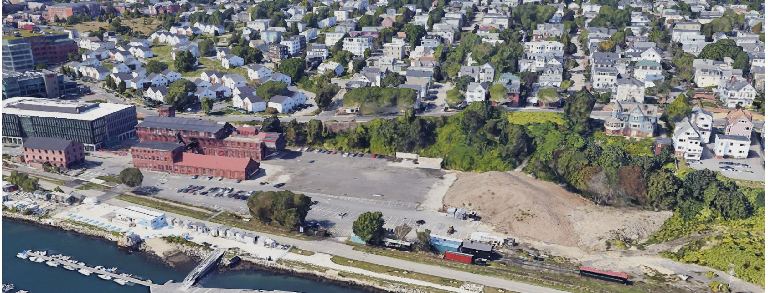
Overall site looking North
