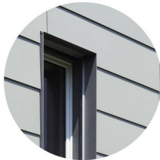
FIBER CEMENT PANELS- TAN LOCATION: Residential Towers
