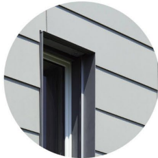
FIBER CEMENT PANELS- TAN LOCATION: Residential Towers
