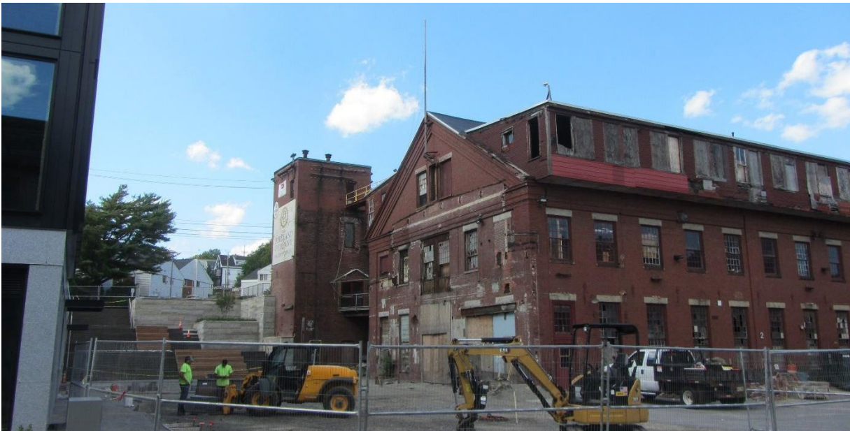
Figure 6: 2022 view of the Buildings 2 & 24. Block 1, at left, was nearing completion with sitework being completed in the foreground.
