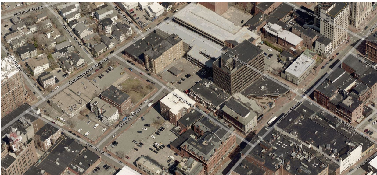
Figure 2: 2022 Aerial view of 48 Brown Street, looking north.
