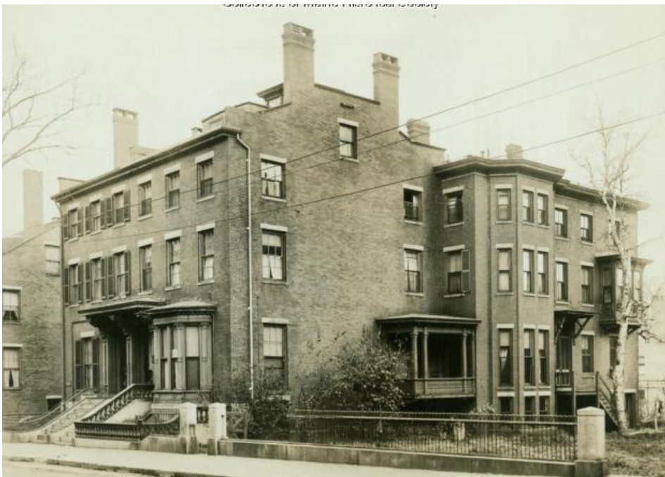
The south side of Free Street was once lined with brick homes such as this one that stood at 134 Free.
