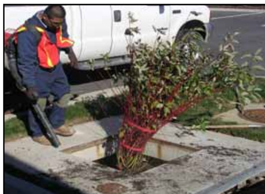
5. Clean area around Filterra
