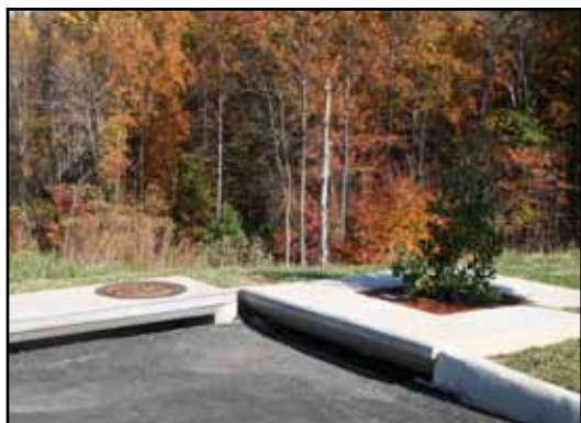
1. Inspection of Filterra and surrounding area
