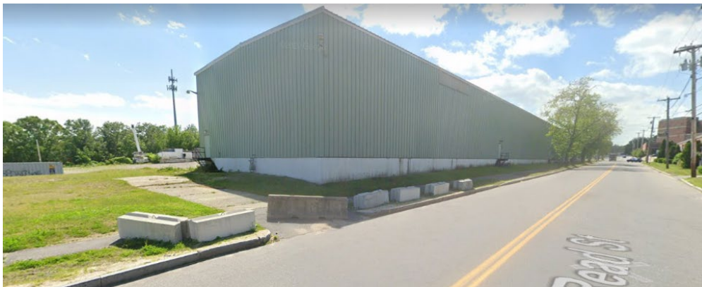
Figure 2 180 Read Street Eastern Entrance
