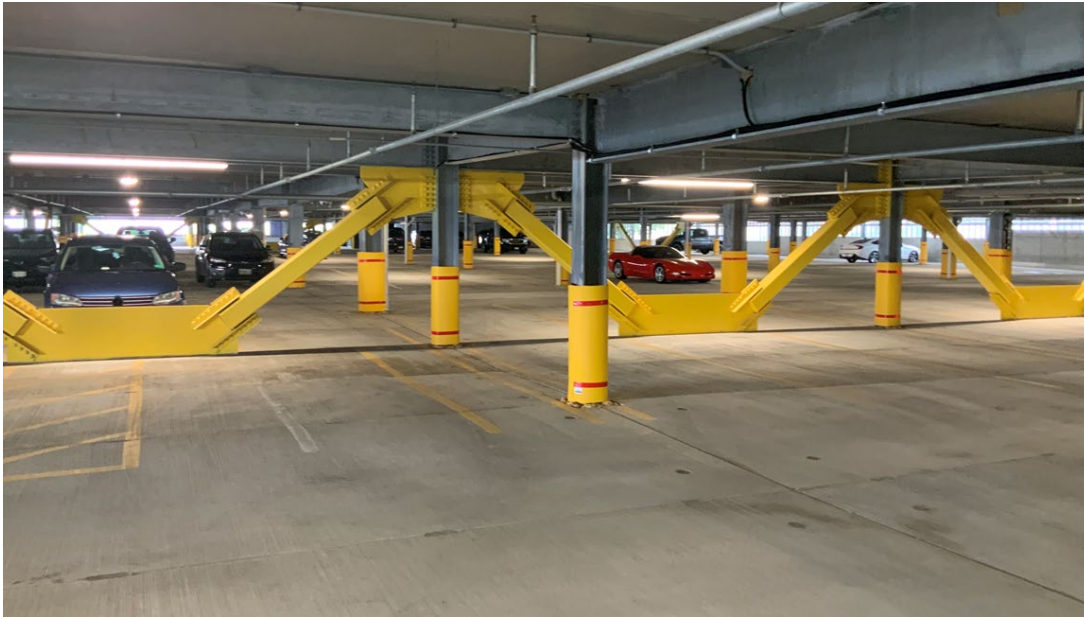
100 Fore St garage P1 level 10:00 am 07/21/23
