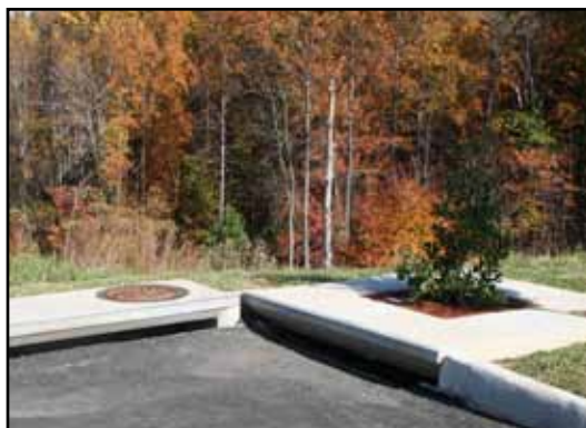
1. Inspection of Filterra and surrounding area
