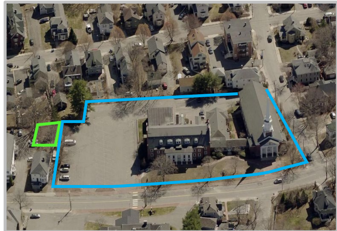
Figure 1: Aerial View of 182 Rear (Outlined in Green) and 186 (Outlined in Blue) Woodford Street
