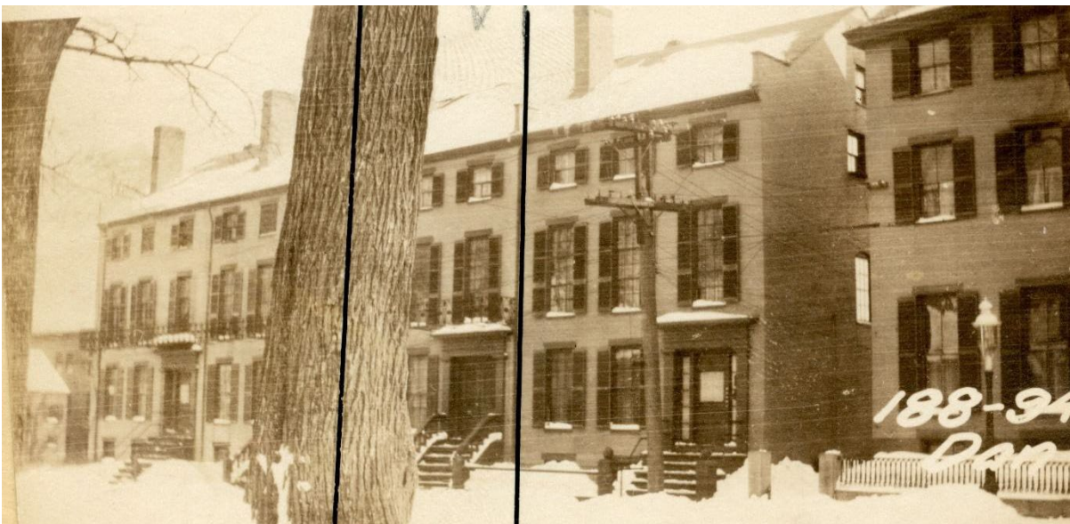
Figure 2: 1924 Tax Photo of 192 Danforth Street ( https://www.mainememory.net/record/45562/image/46261 ).
