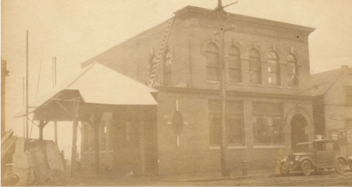
Figure 2: 1924 Tax Photo for 84 Commercial Street ( https://www.mainememory.net/record/86887 ). The scales were contained in the wood frame structure to the left of the building which is no longer extant.
