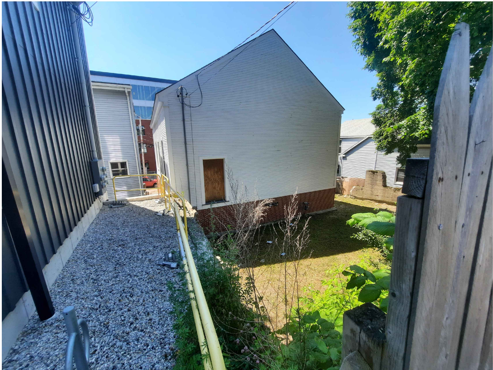
10. VIEW FROM FEDERAL STREET SIDEWALK
