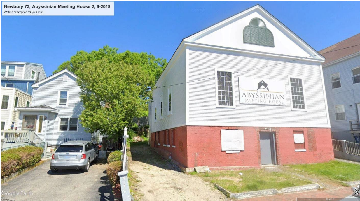
Figure 4: Appearance in 2019, prior to masonry and door work on the ground floor
