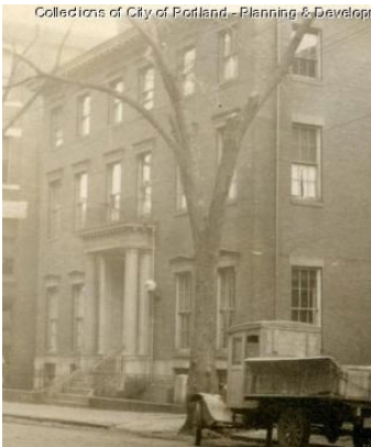
120-24 Free Street Demolished after 1960
