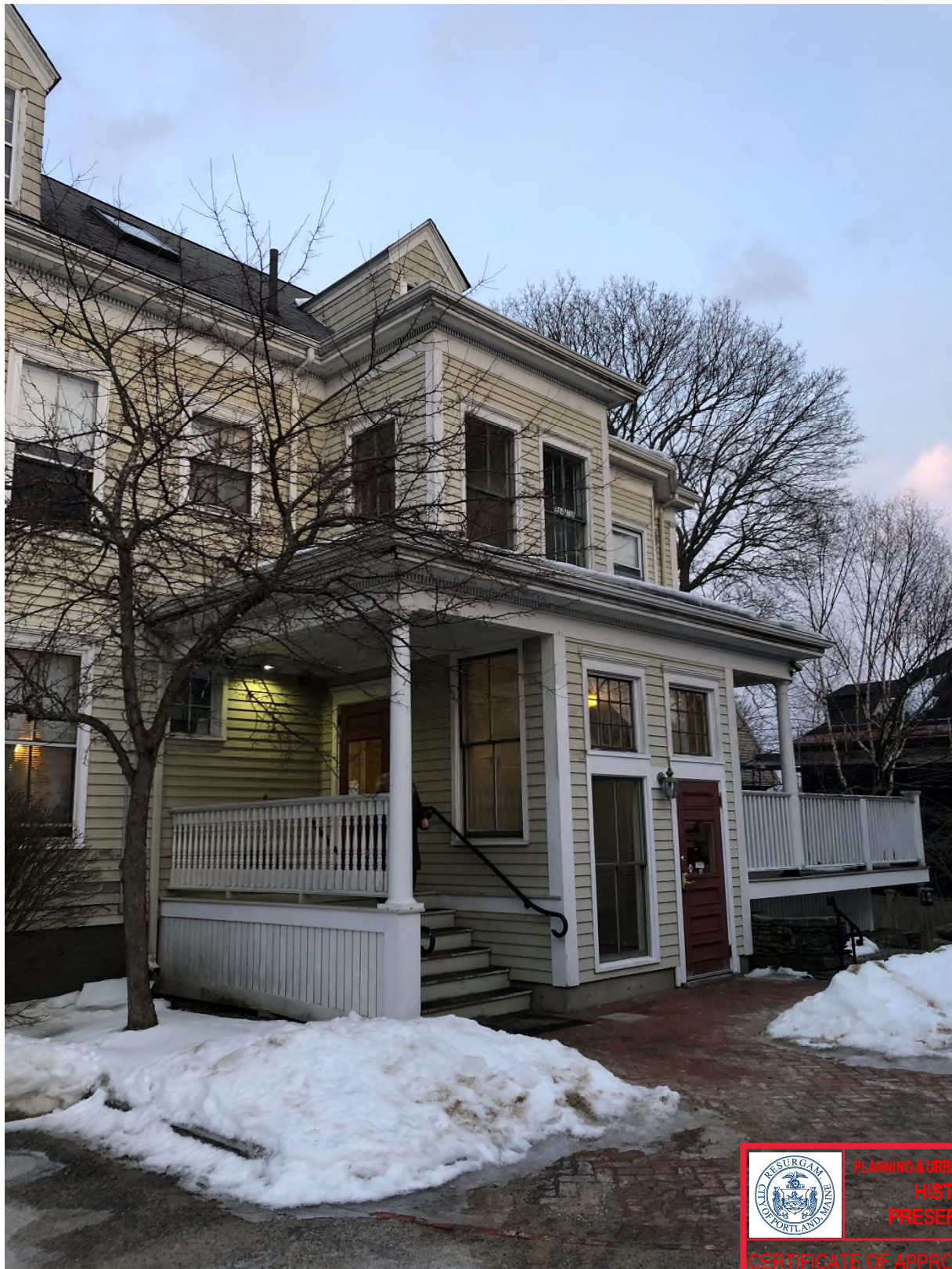
Figure 6: 1994 Addition to the main house, garage side
