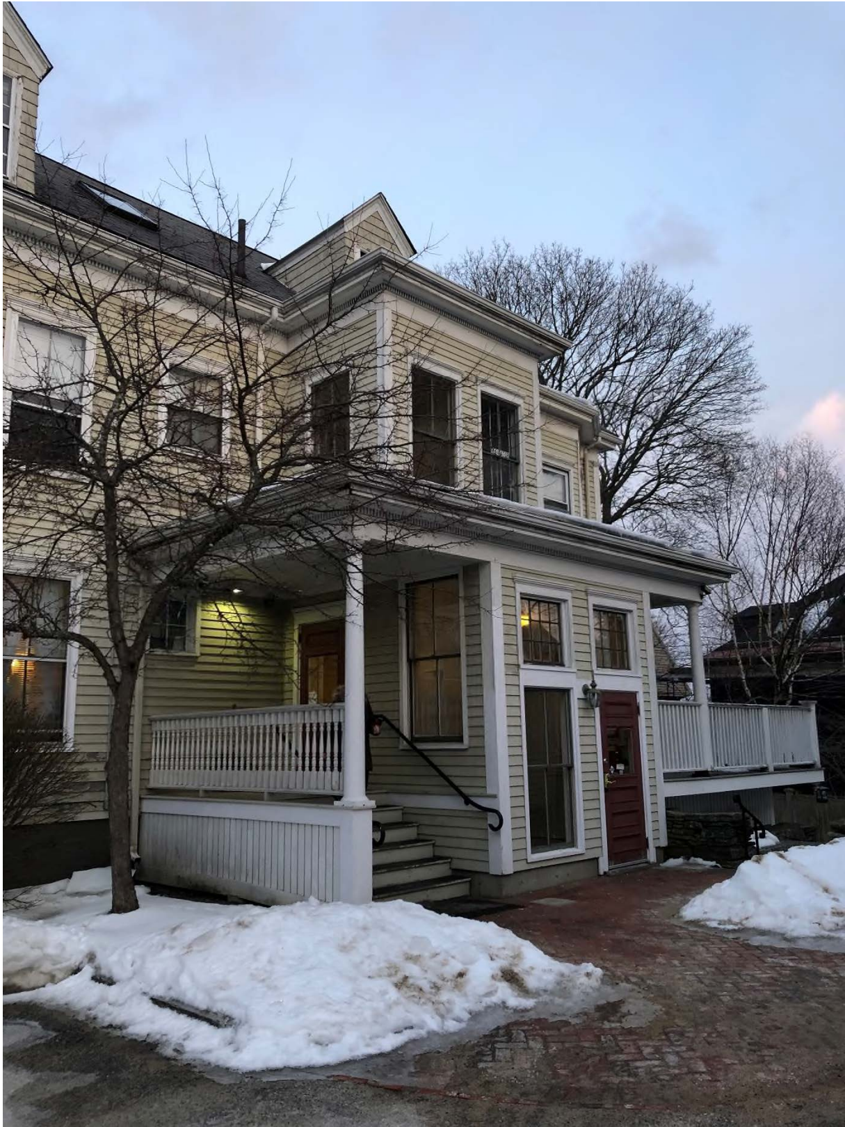
Figure 6: 1994 Addition to the main house, garage side
