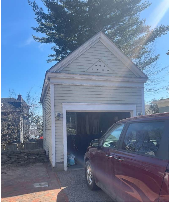
Figure 7: 1994 Garage structure - front view
