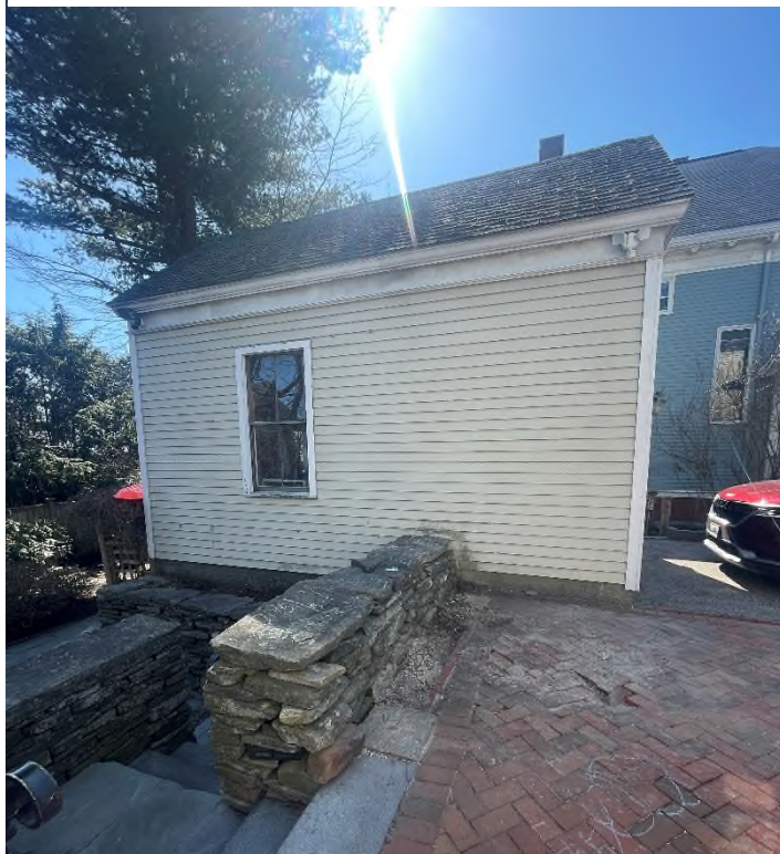
Figure 8: 1994 Garage structure – house-side view
