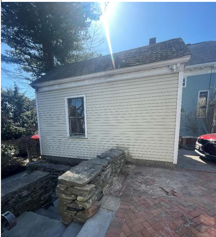
Figure 8: 1994 Garage structure – house-side view
