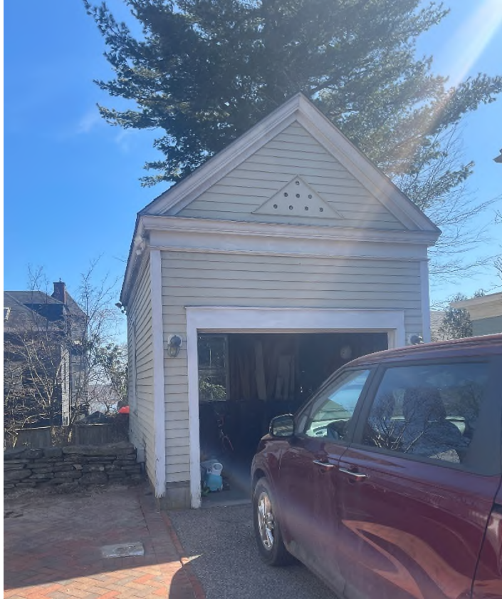
Figure 7: 1994 Garage structure - front view
