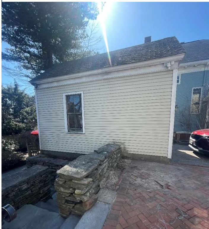
Figure 8: 1994 Garage structure – house-side view
