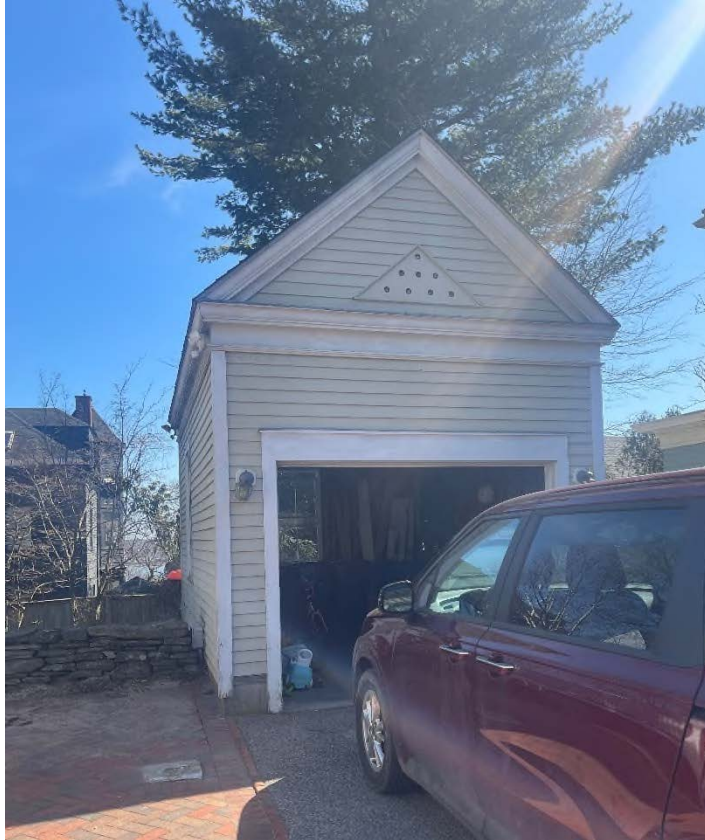
Figure 7: 1994 Garage structure - front view
