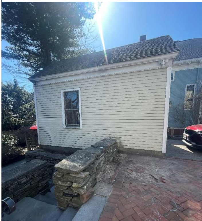
Figure 8: 1994 Garage structure – house-side view
