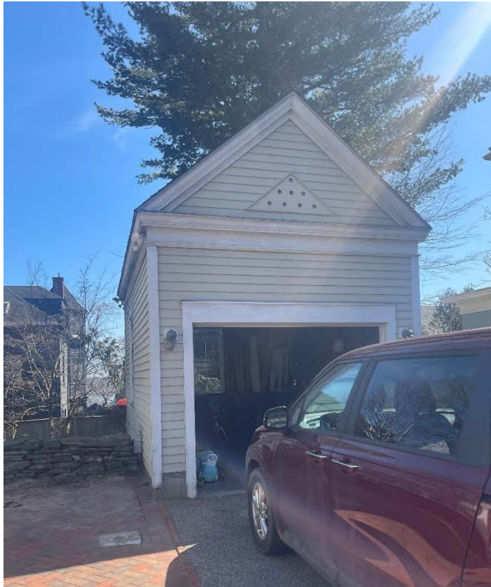
Figure 7: 1994 Garage structure - front view
