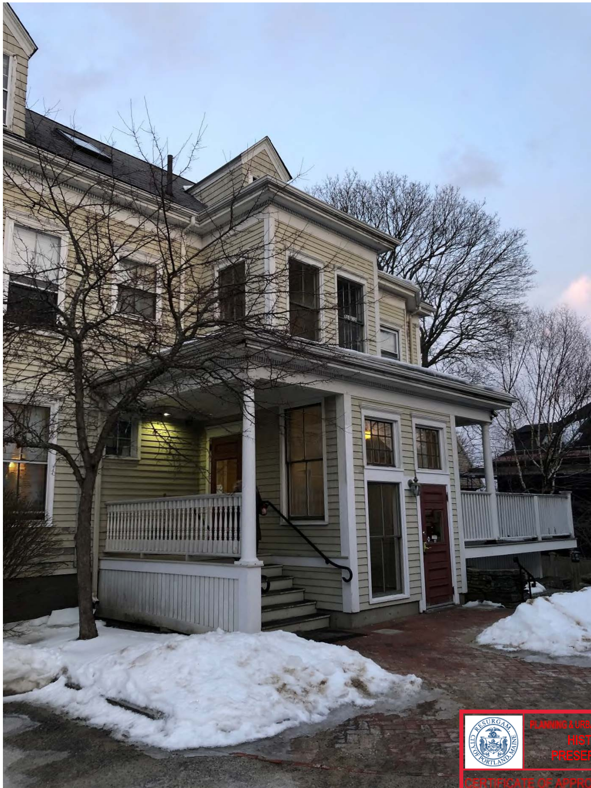
Figure 6: 1994 Addition to the main house, garage side
