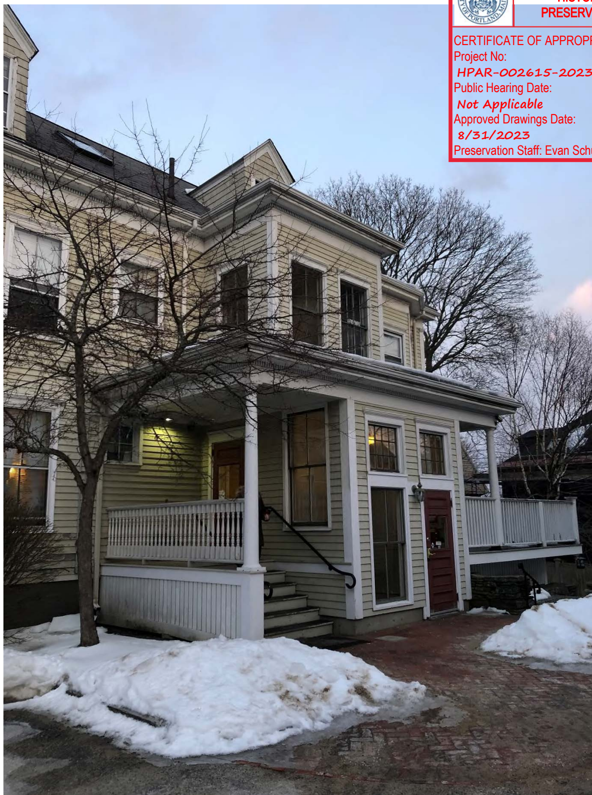
Figure 6: 1994 Addition to the main house, garage side
