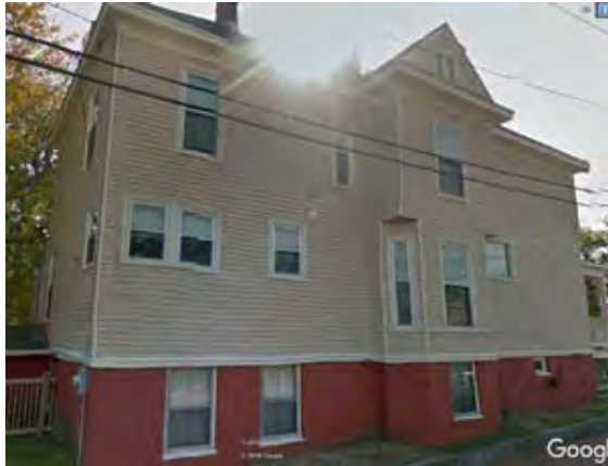
89 North Street MONTREAL STREET FACING West
