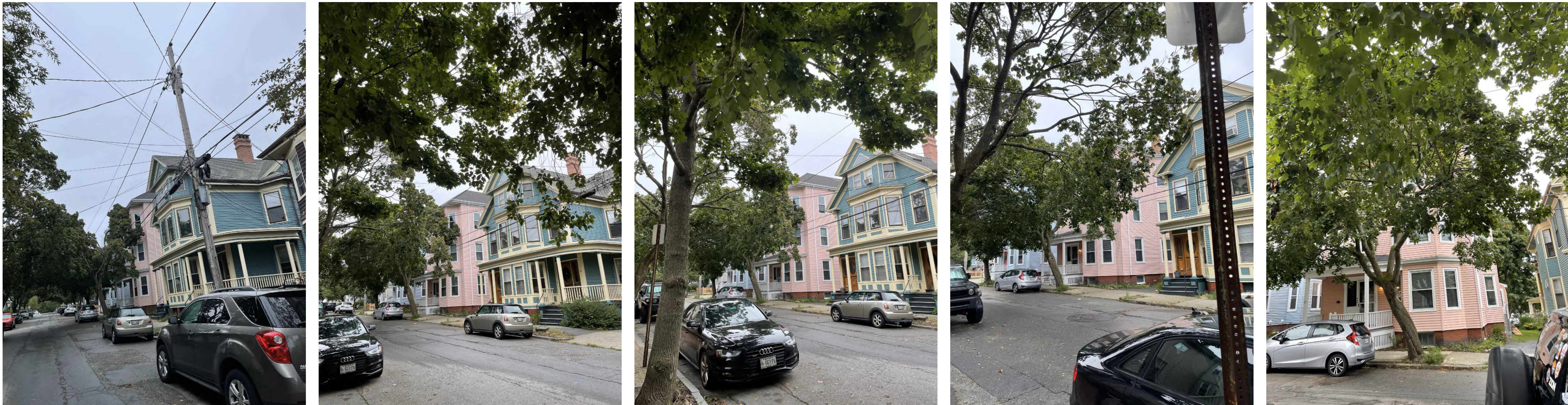
2 MORNING STREET PHOTOS - WALKING NORTH ON MORNING STREET ON SIDEWALK ACROSS STREET
