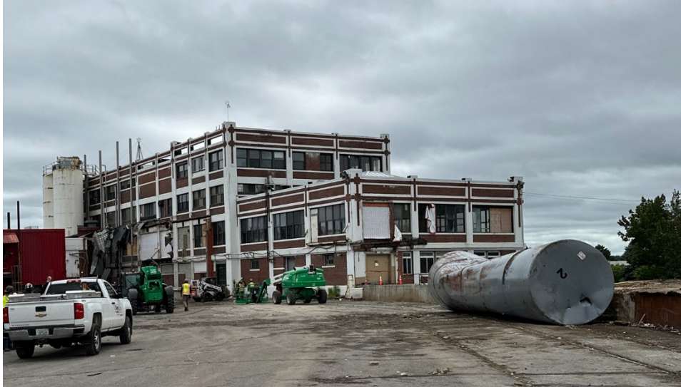
Existing conditions- north facade
