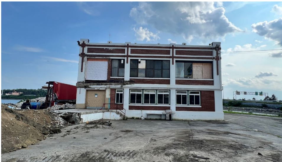
Existing conditions- north façade
