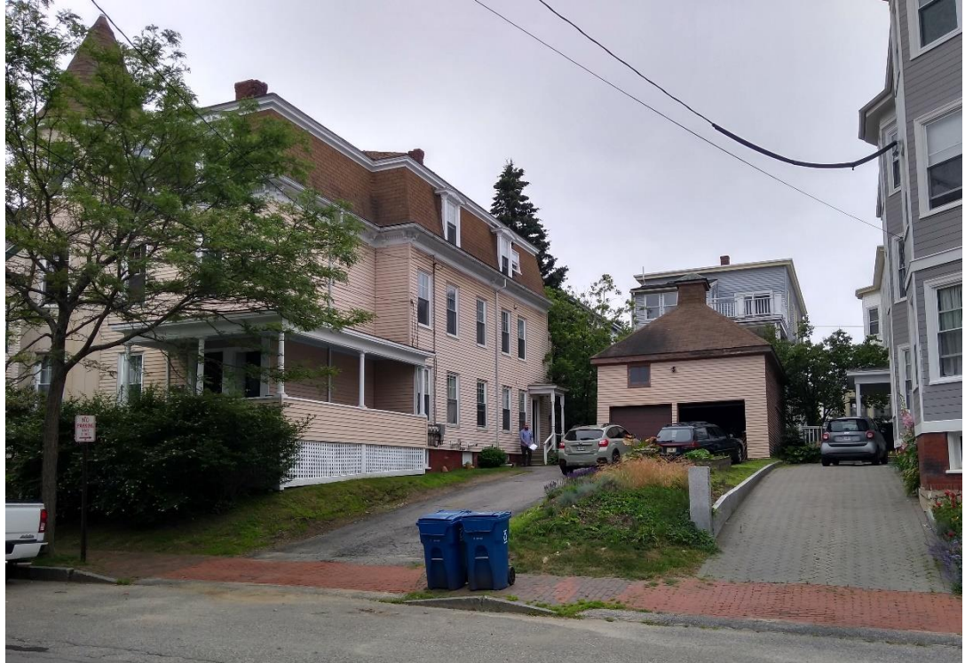
Existing Carriage House from Morning Street
