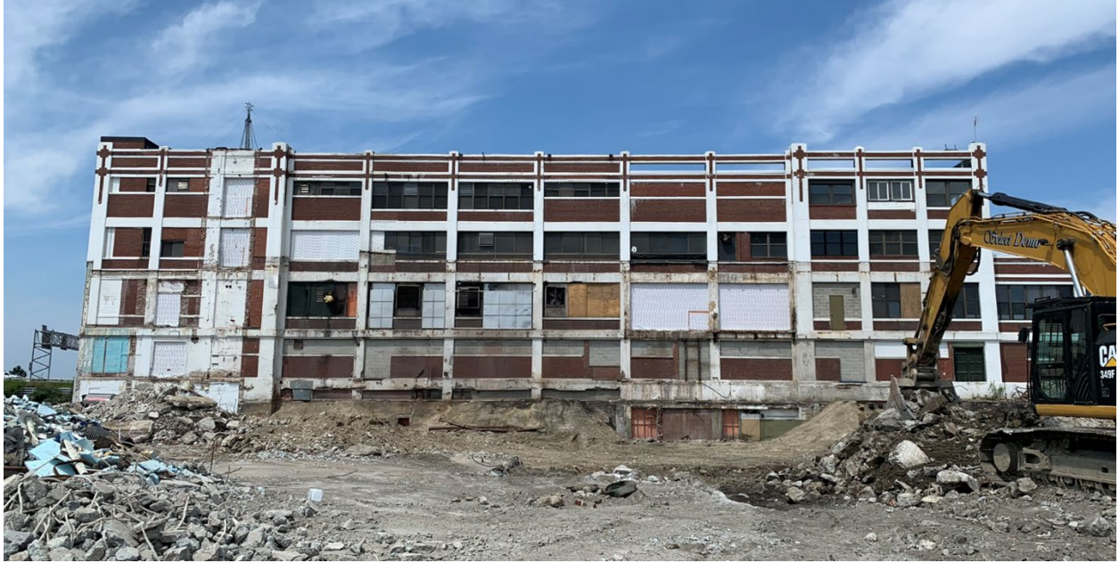
Existing conditions- east façade
