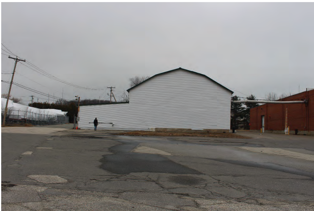
15. Site, Woodworking/Storage Building, looking northwest.
