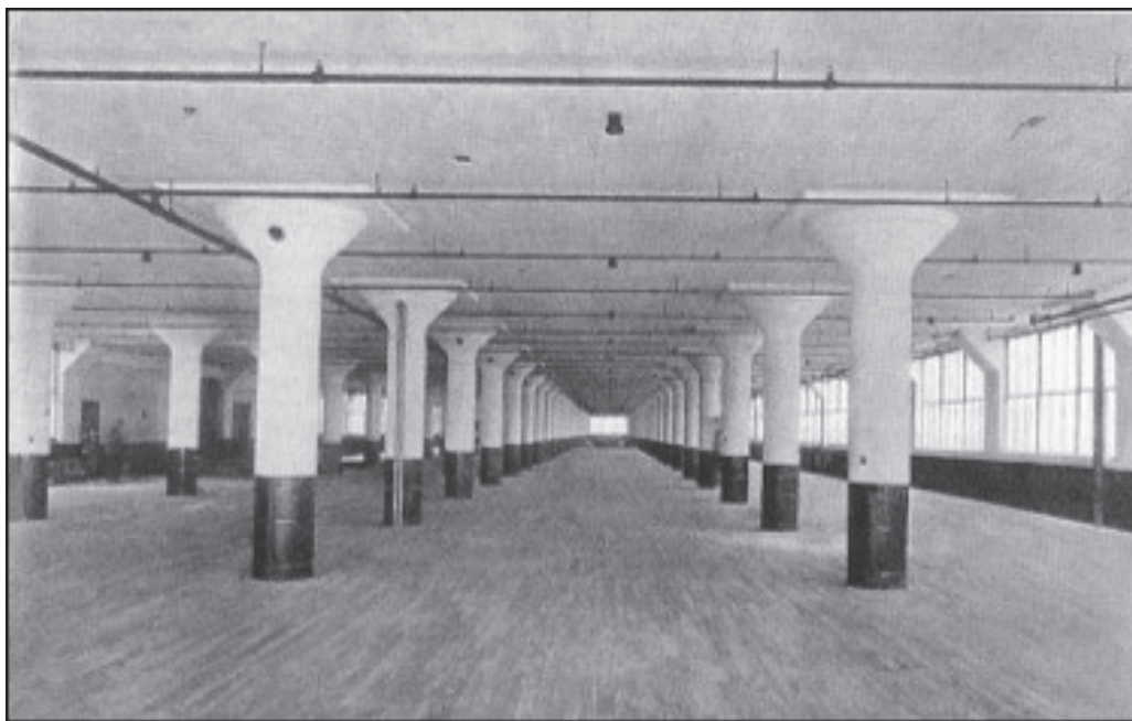
Figure 23: Union Switch & Signal Co. - Swissvale, PA - designed ca. 1905 by C.A.P. Turner (Image Source: Bradley, Betsy Hunter. The Works )
