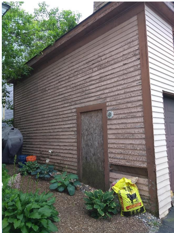
Carriage House Apartment Side
