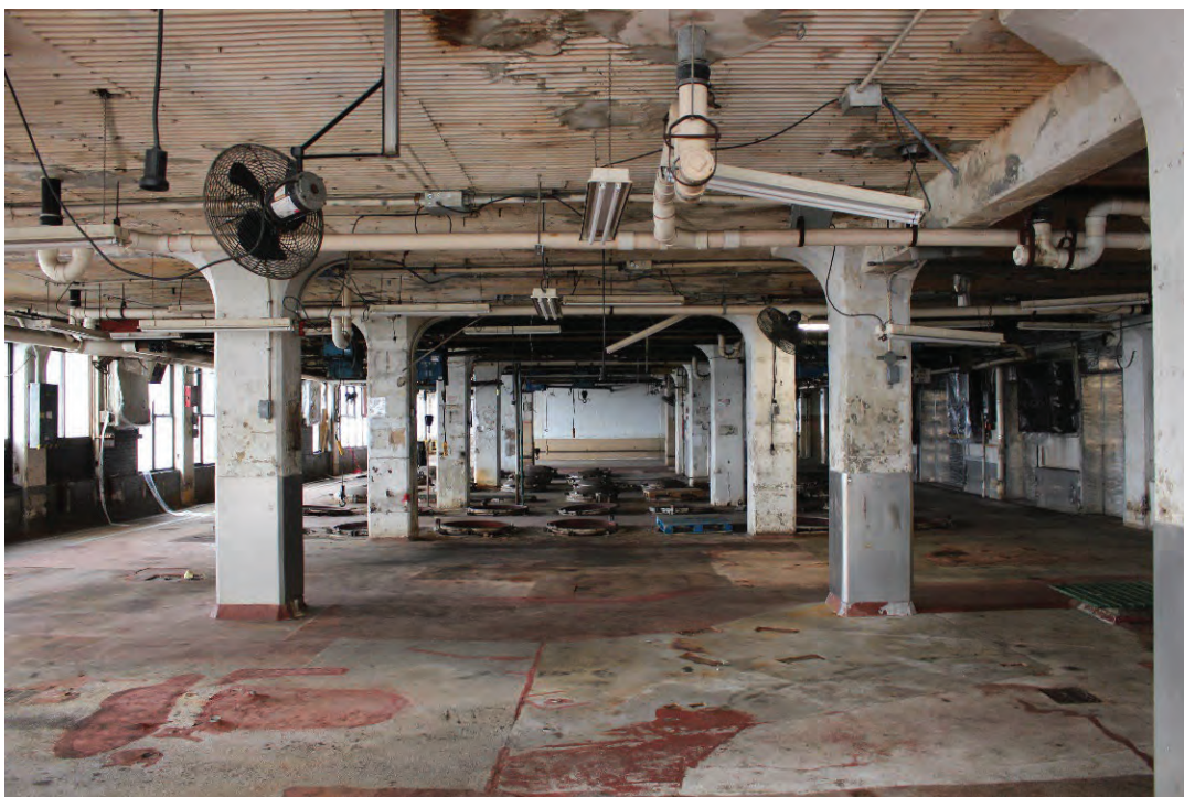
9. B&M Factory, Second Floor, looking north.
