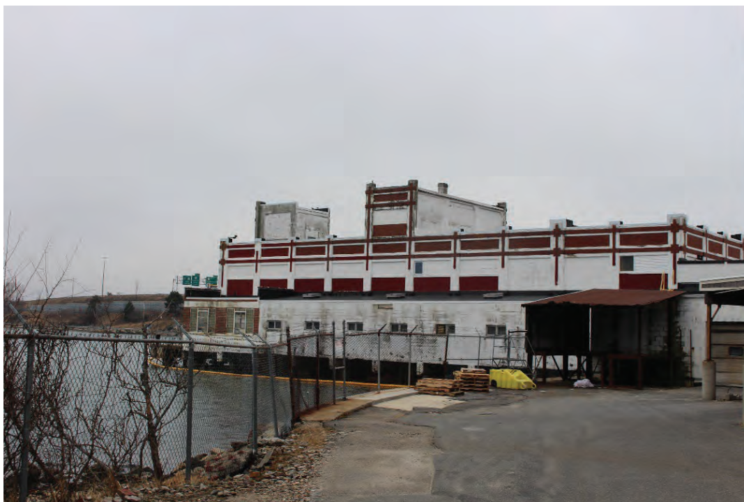
13. Site, Codfish Canning Building, looking southwest.
