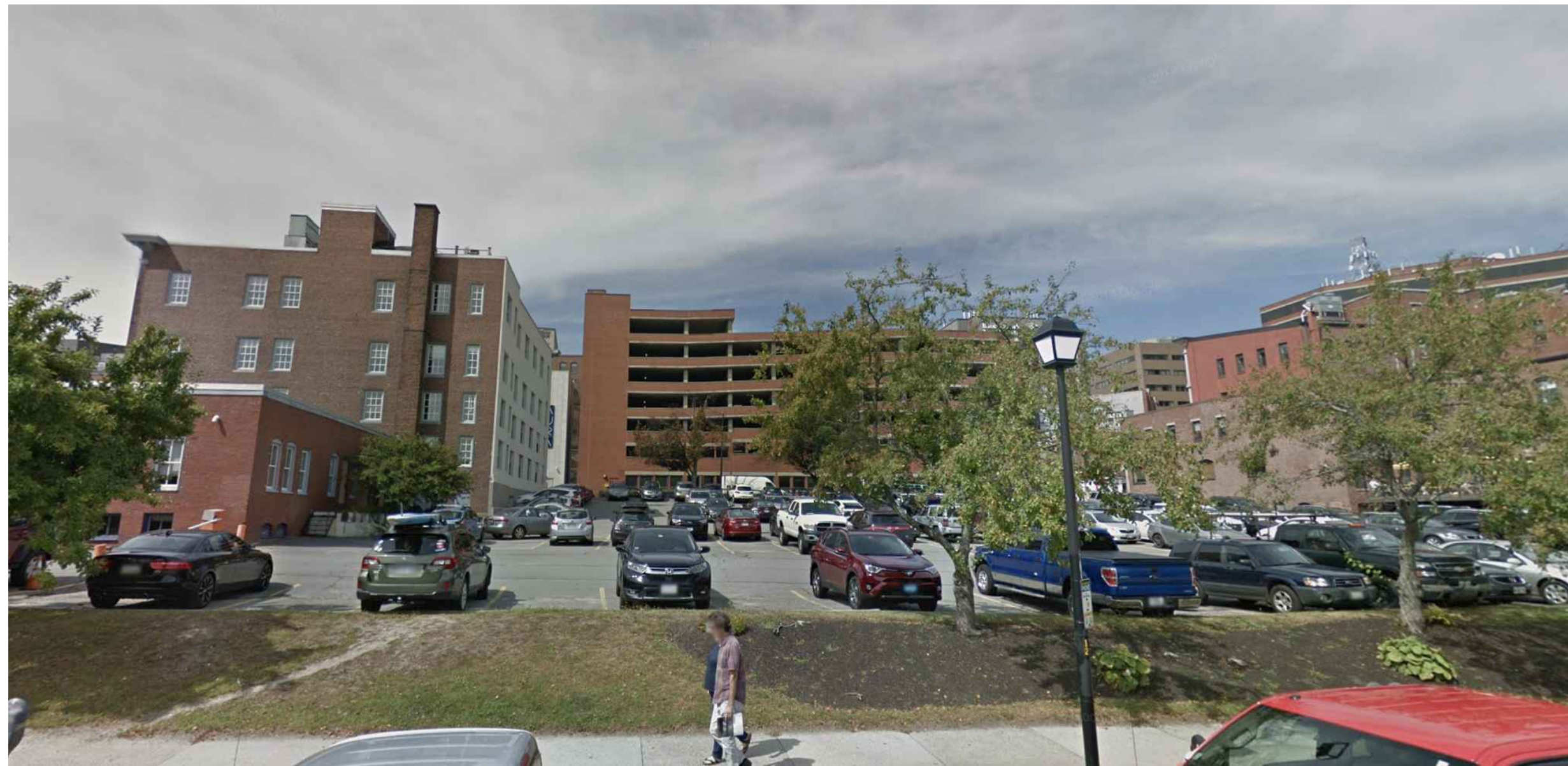
4 VIEW LOOKING WEST FROM SPRING STREET
