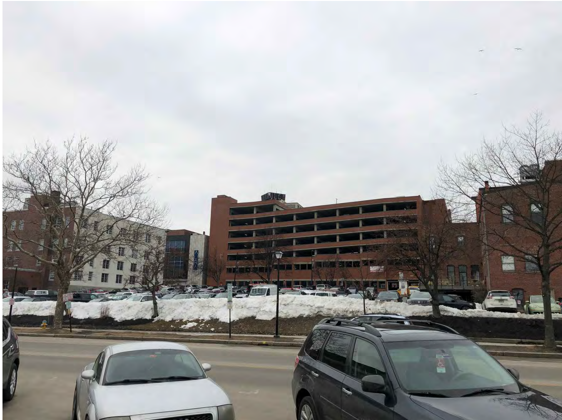
3 VIEW LOOKING WEST FROM SPRING STREET
