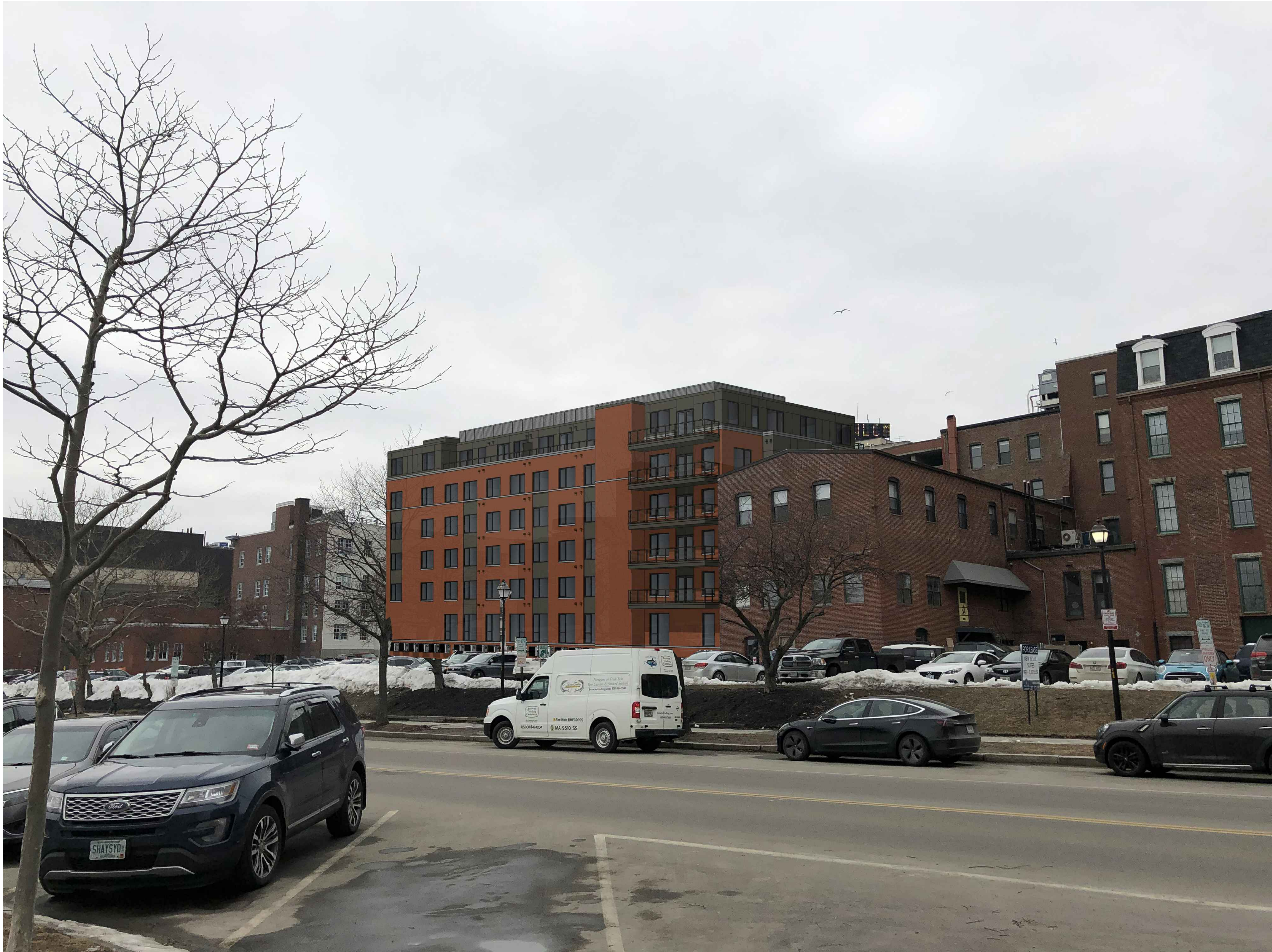
1 VIEW LOOKING WEST FROM SPRING STREET
