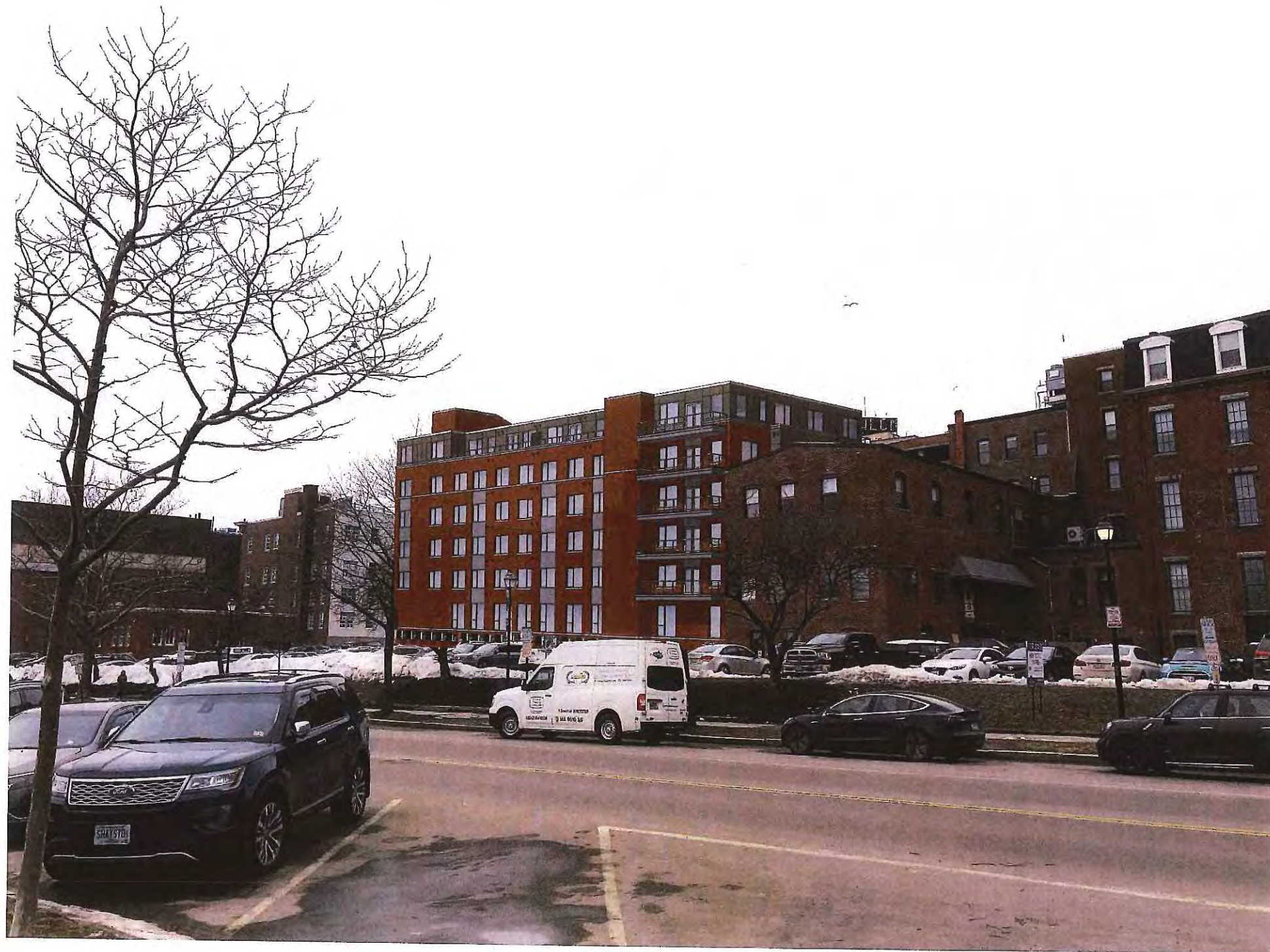
① VIEW LOOKING WEST FROM SPRING STREET
