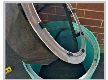
Bypass protection - Domed overflow with filter insert
