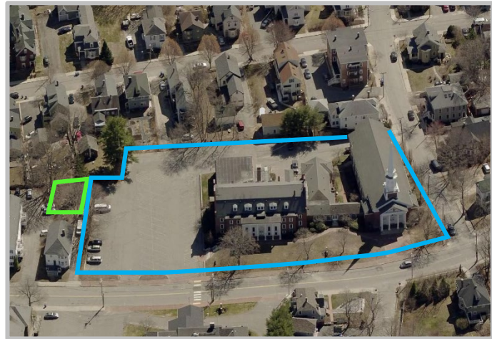
Figure 1: Aerial View of 182 Rear (Outlined in Green) and 186 (Outlined in Blue) Woodford Street
