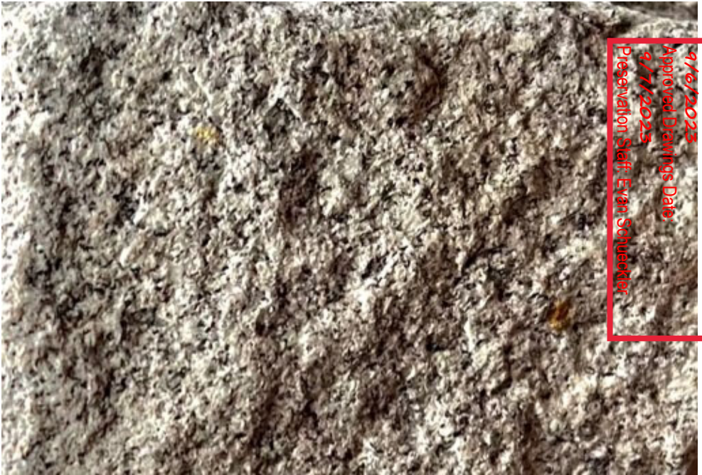
EXISTING GRANITE FACADE
