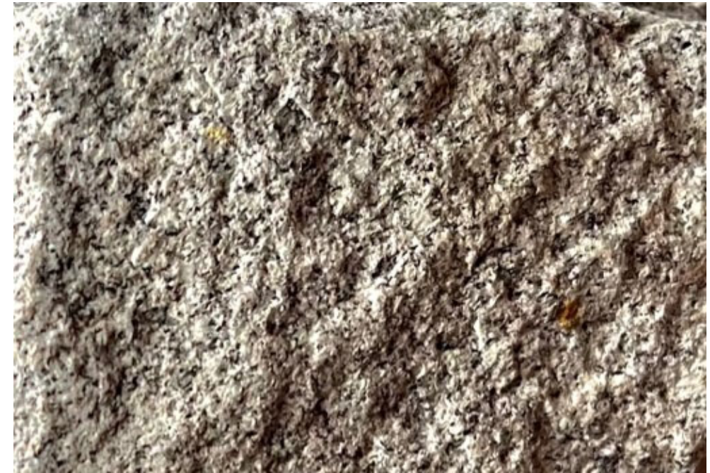
EXISTING GRANITE FACADE
