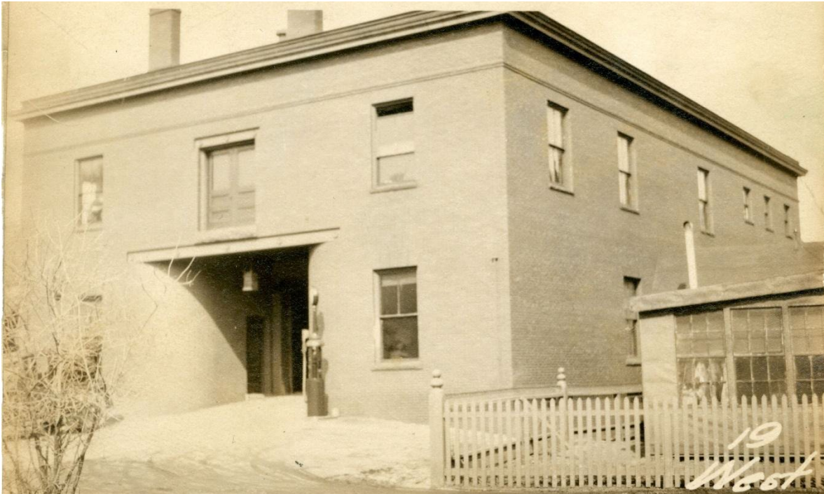
Figure 2: 1924 Tax photo showing the contributing garage structure at 19 West Street.
