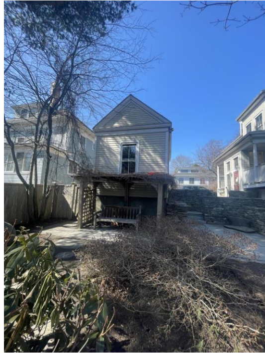
Rear of Garage
