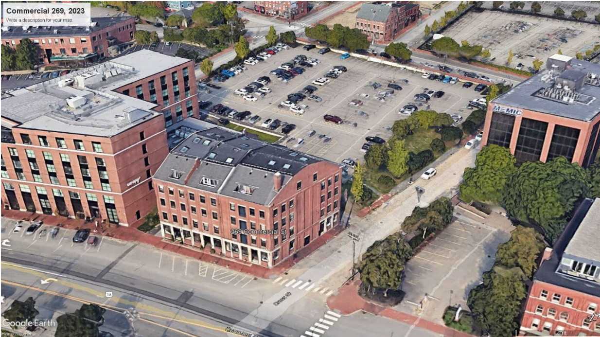
Figure #2: View of 269 Commercial Street, showing location of the existing chimney.
