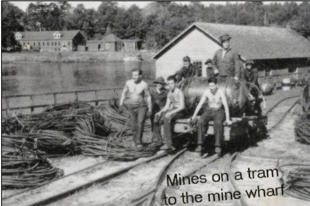
Tramway on Mine Wharf (ca. 1930) from collection of Fort McKinley Museum
