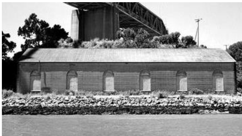
Yerba Buena Torpedo Storehouse - California built 1891; photo 1998
