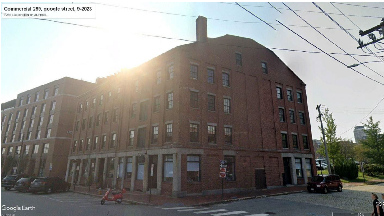
Figure #3: Street view of 269 Commercial Street, showing location of the existing chimney.
