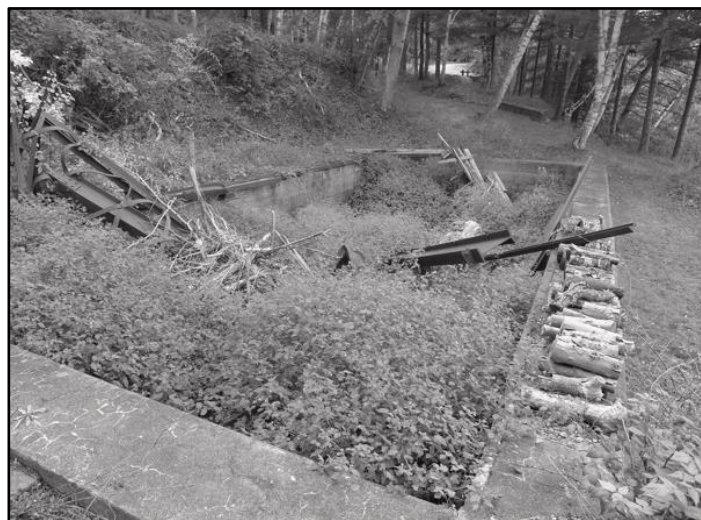
Foundation of Cable Tank Building
