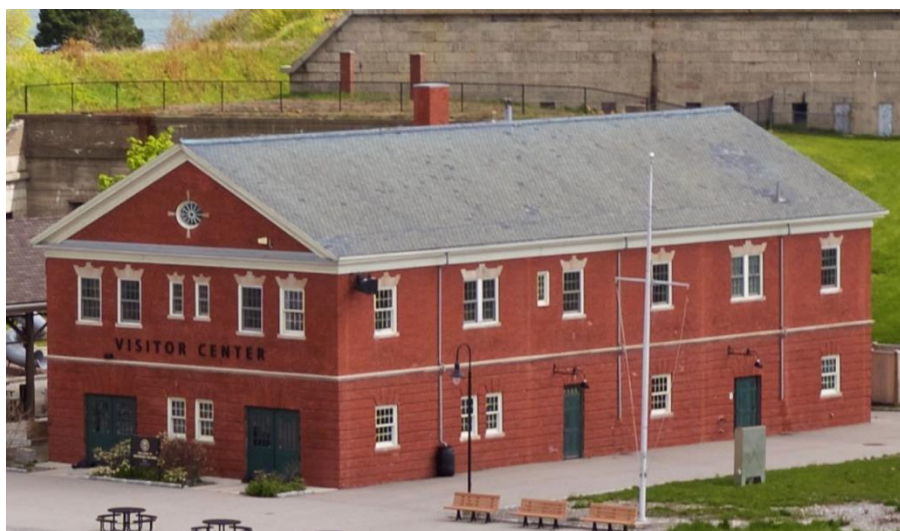
Fort Warren – Boston Harbor Former Torpedo Storehouse (built 1906)
