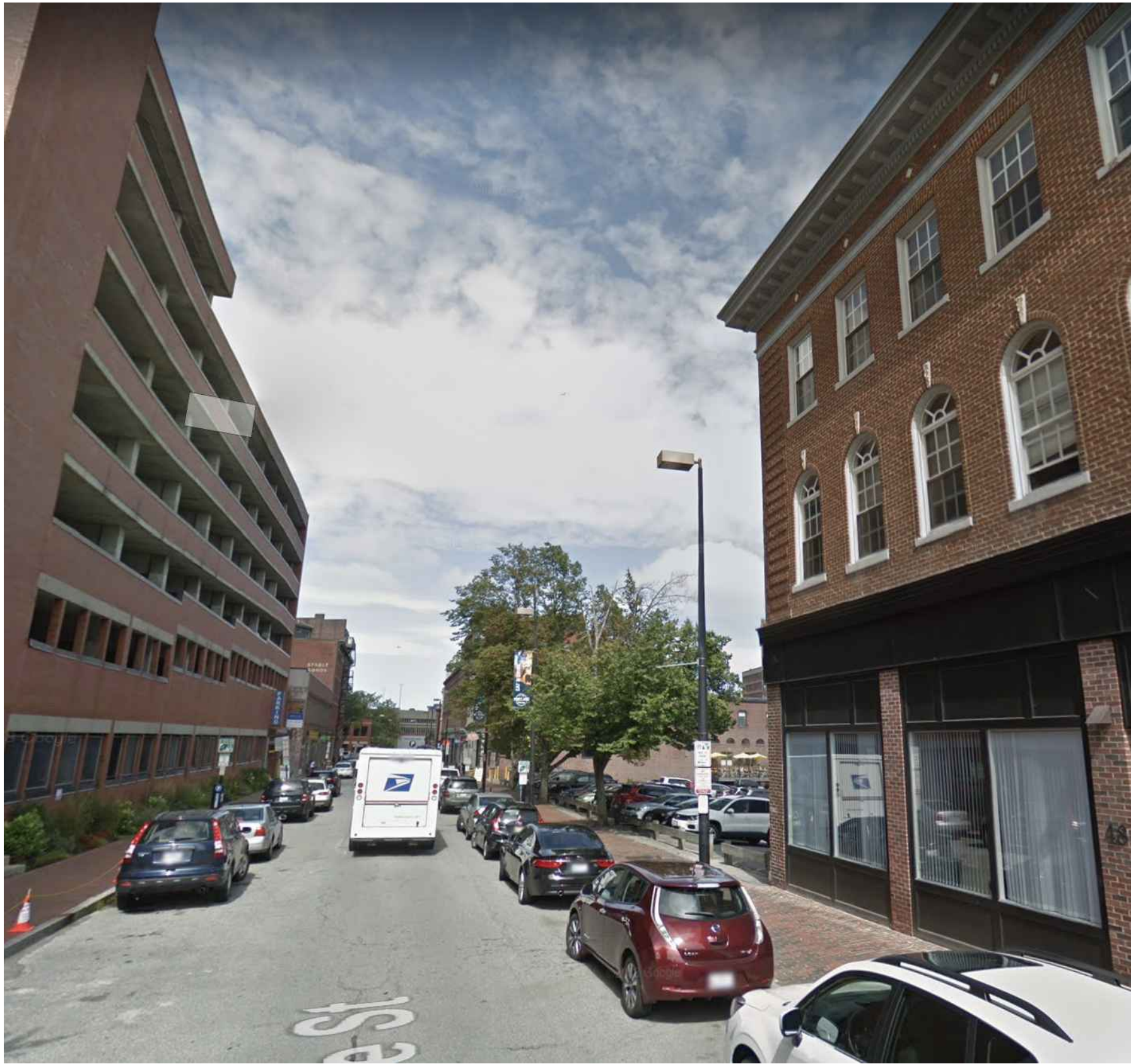
1 VIEW LOOKING NORTHEAST ON FREE STREET
