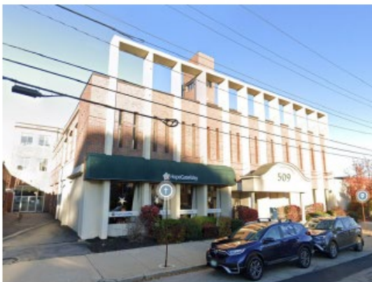
Figure 2: Existing Façade, photo provided by applicant.
