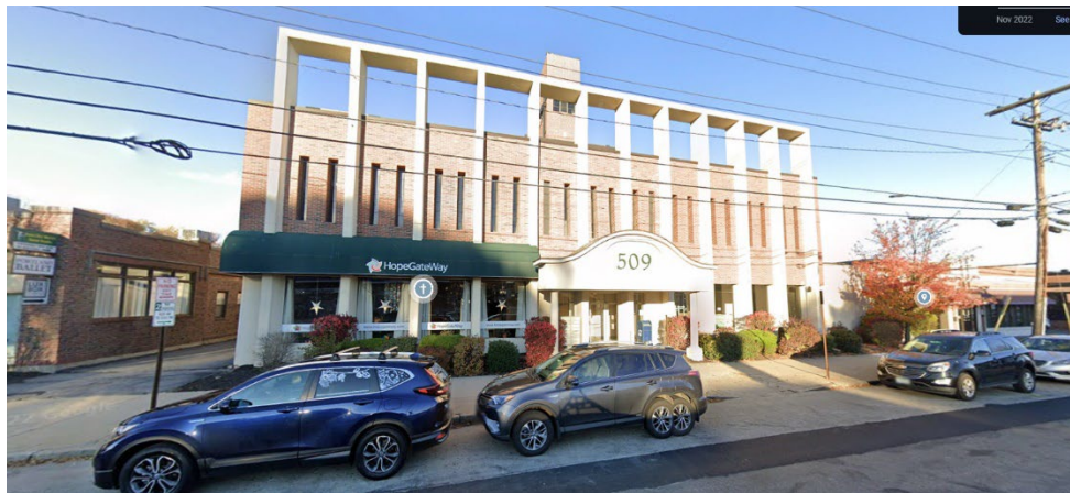
Figure 4 Streetview from Forest Avenue
