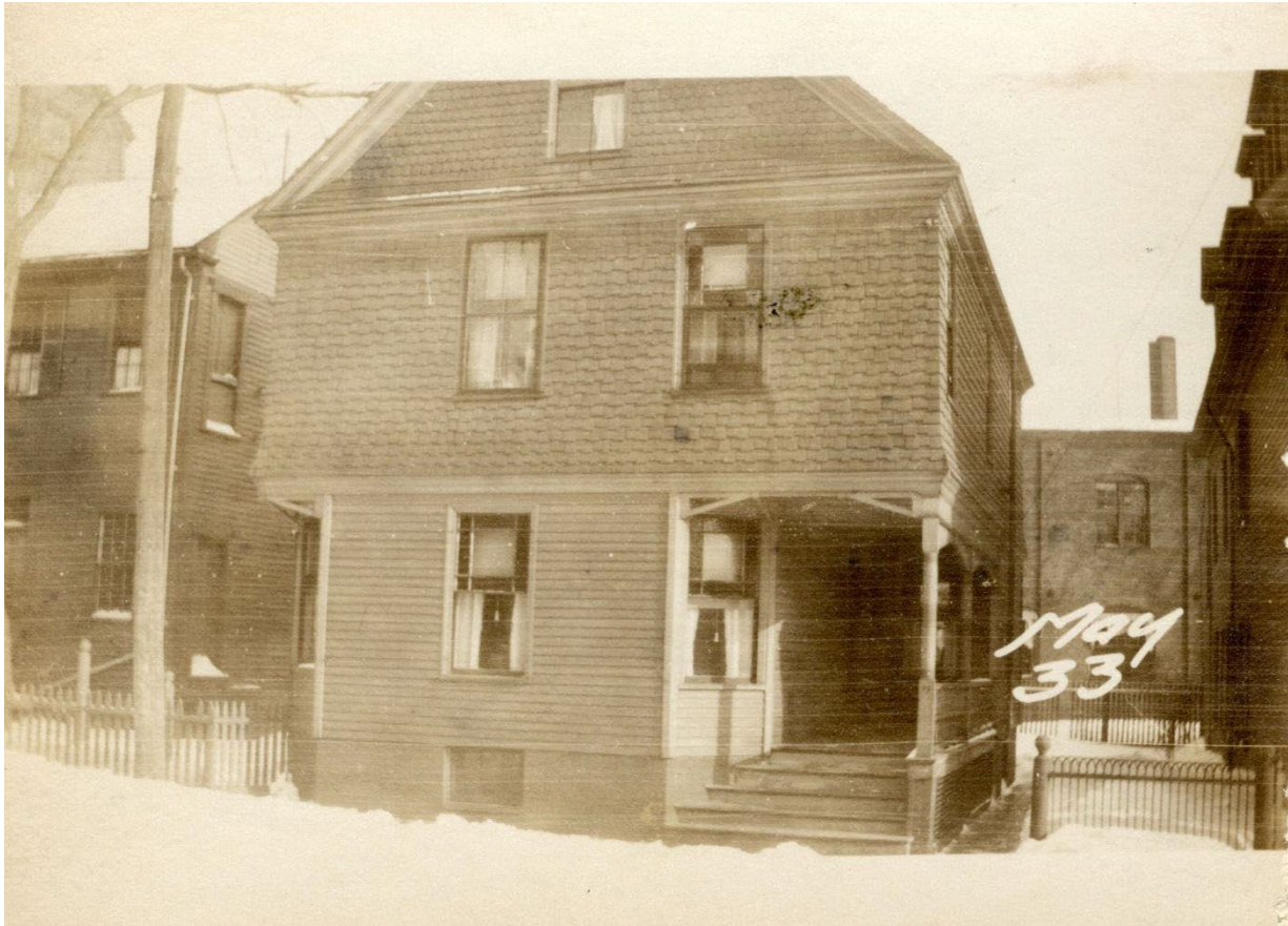
Figure #3: 1924 photo of 31-33 May Street
