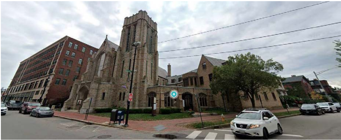
Figure 1: 2023 Google Street View showing the Williston-Immanuel United Church (Center) with the State Theater up High Street (left) and Deering Street to the west (right).
