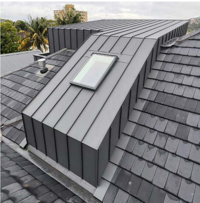
Dormer with standing seam walls and roof. (We intend a slightly more pronounced eave and rake clad in metal.)
