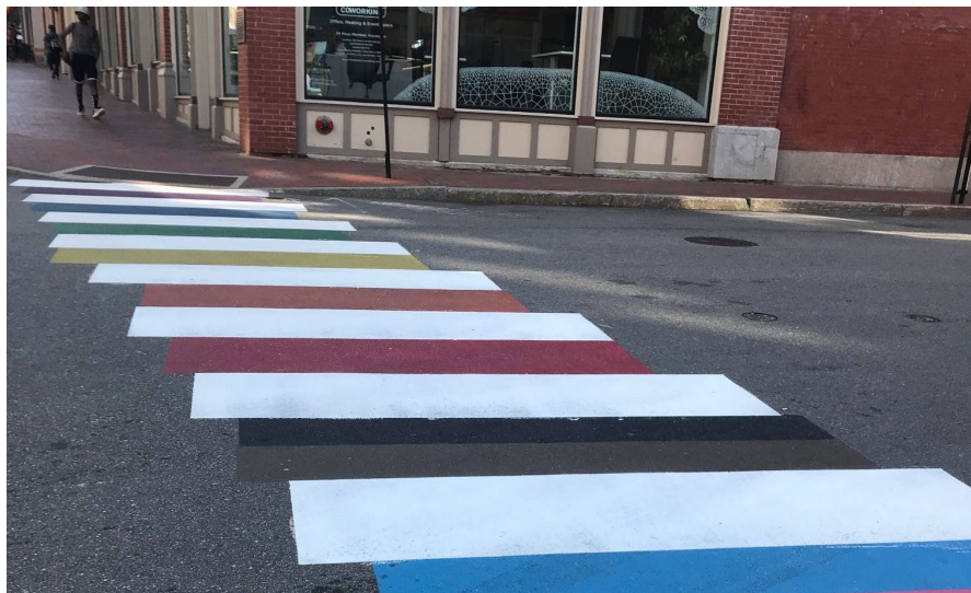
Figure 14: Temporary crosswalk painting
