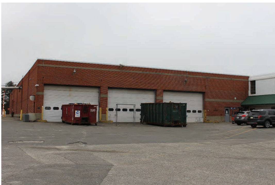
14. Site, Storage/Labeling Building looking northwest.
