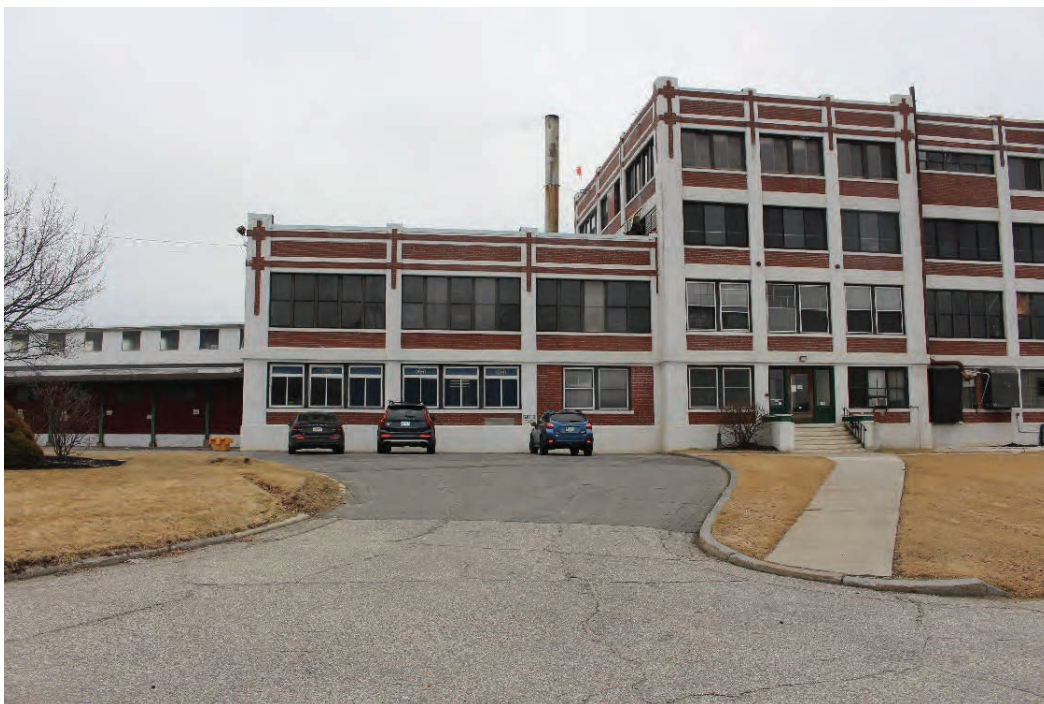
2. B&M Factory, West Elevation, looking east.
