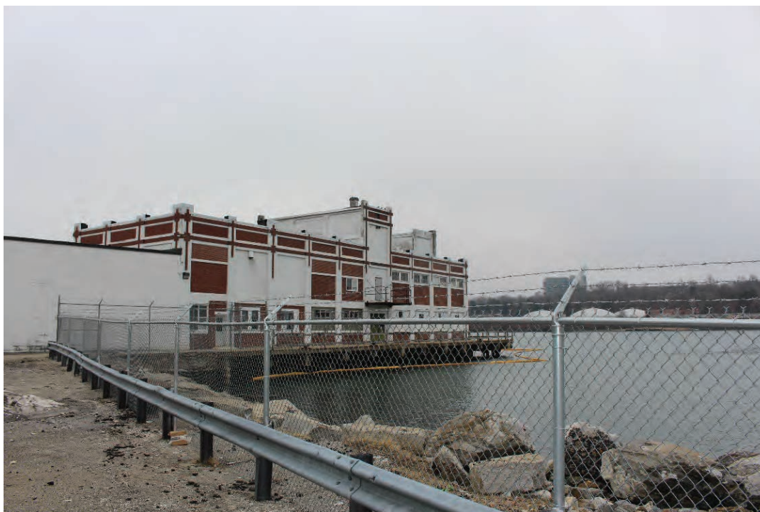
11. Site, Codfish Canning Building, looking southeast.
