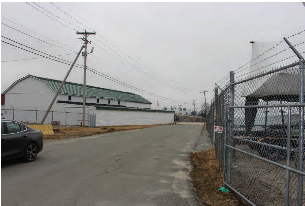
16. Site, Entrance and Woodworking/Storage Building looking south.
