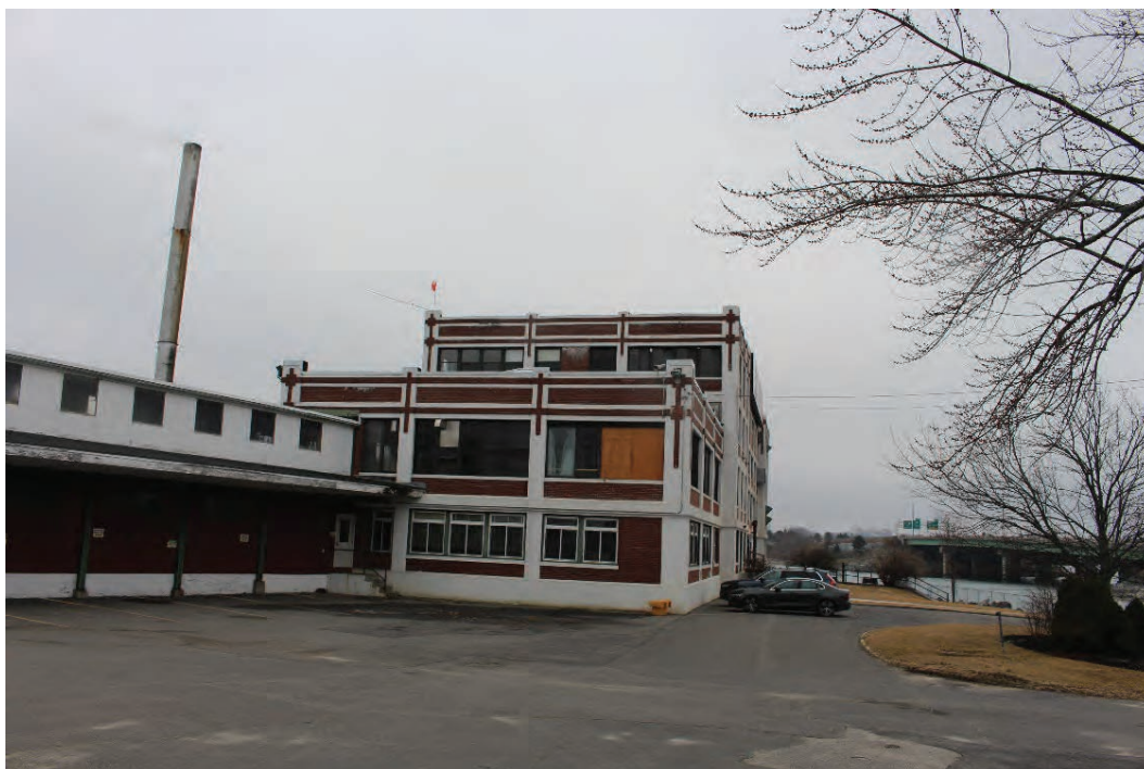
4. B&M Factory, North Elevation, looking south.
