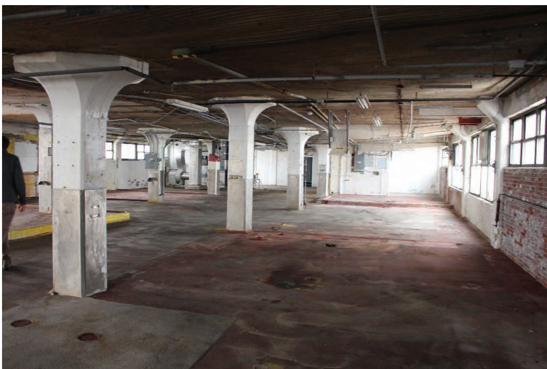
10. B&M Factory, Fourth Floor, looking south.
