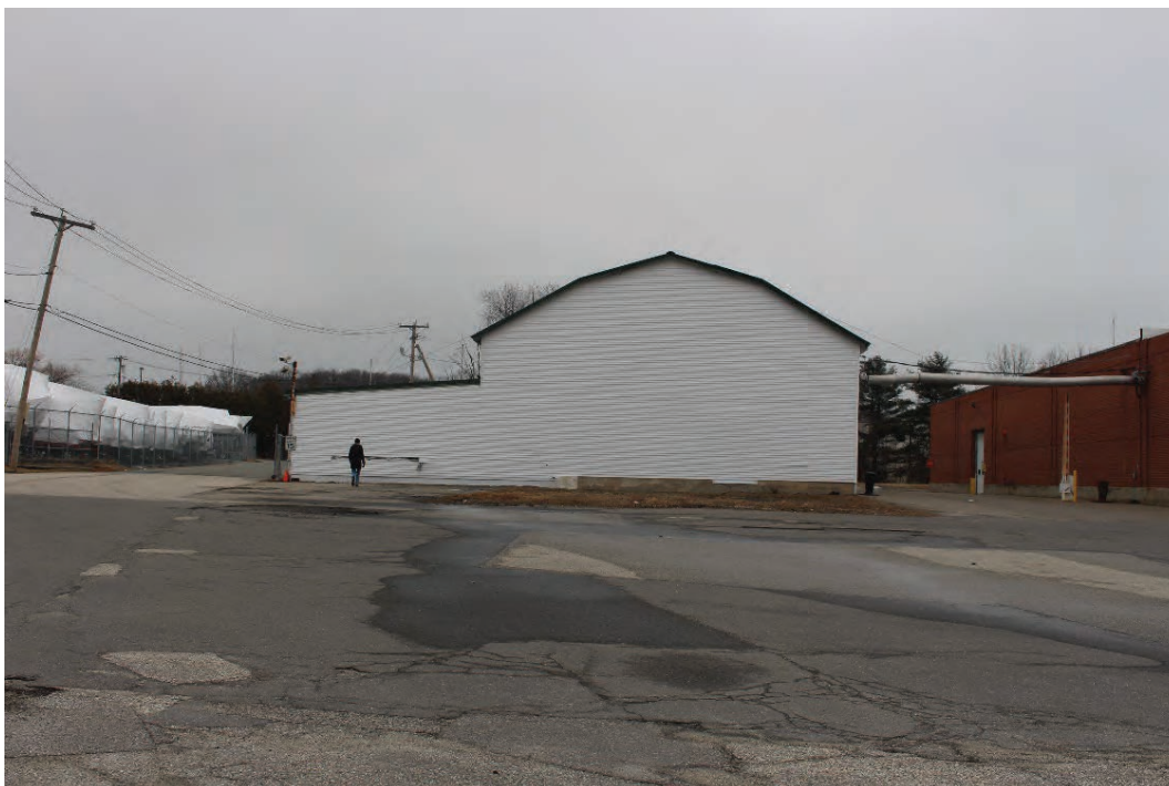
15. Site, Woodworking/Storage Building, looking northwest.
