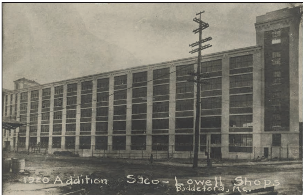
Figure 24: Saco-Lowell Shops Building 30 - Biddeford, Maine
