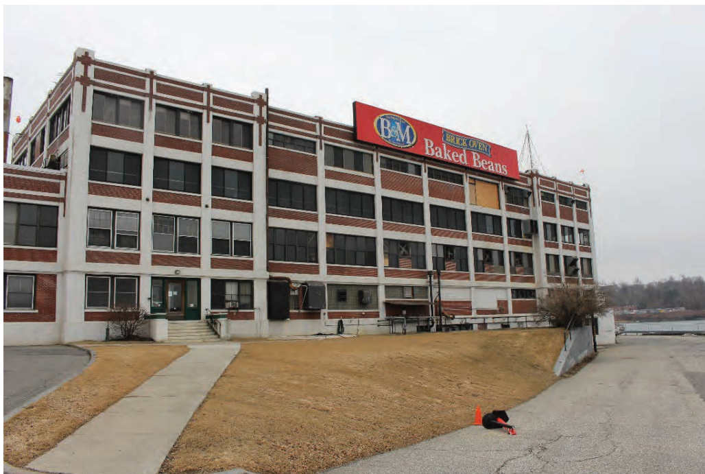
1. B&M Factory, West Elevation, looking southeast.
