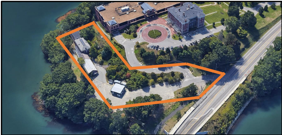
Figure 2: The existing site
