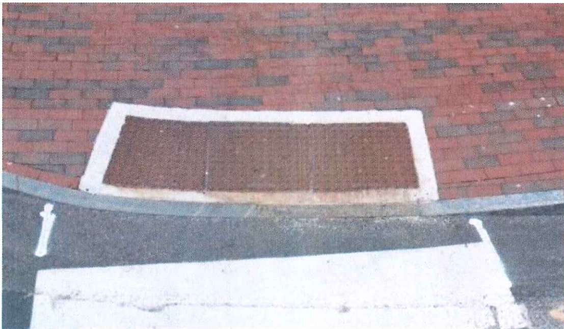
Photo Description: Uncoated cast iron detectable warning panels proposed for the curb ramps. Proposed brick and granite curbing to match the above photograph.
