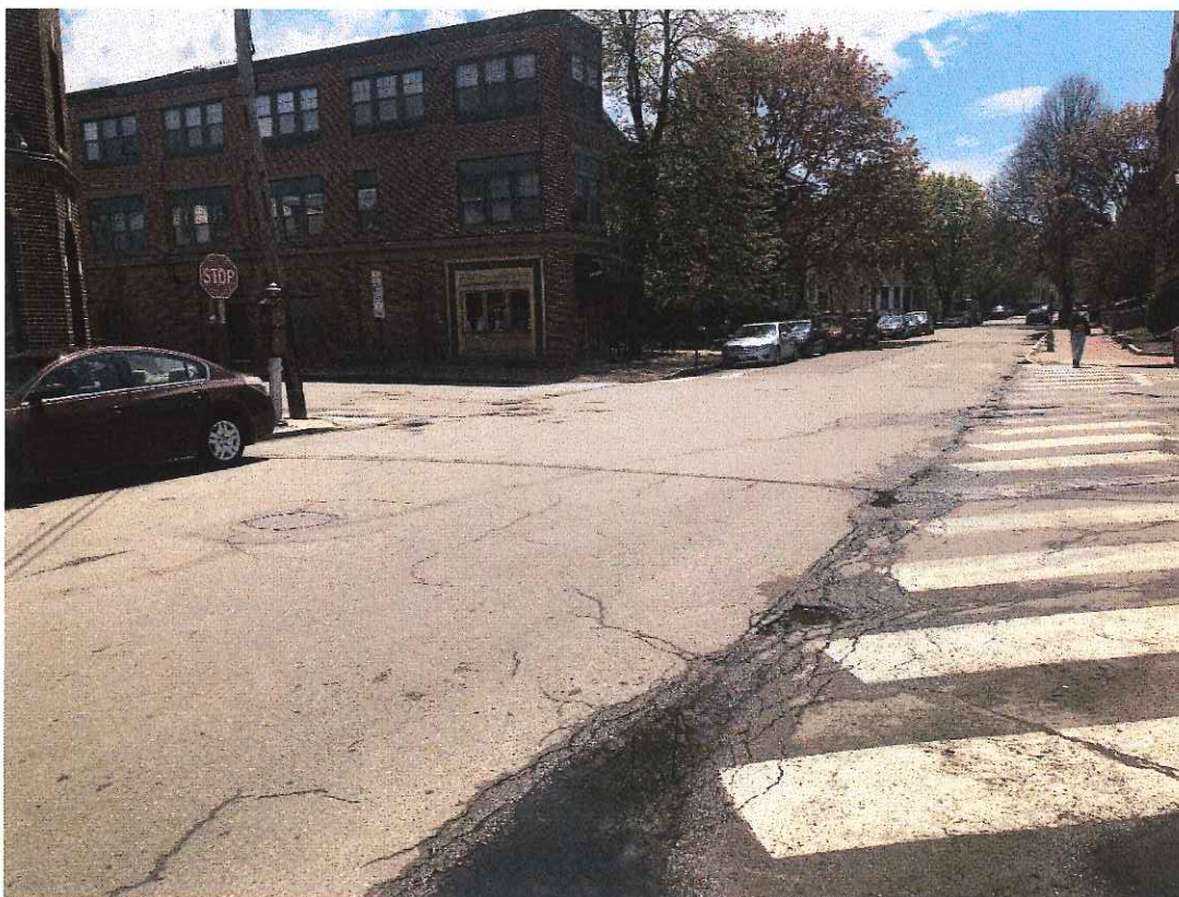
Photo 2: Looking northwest toward Clark Street and Pine Street.
