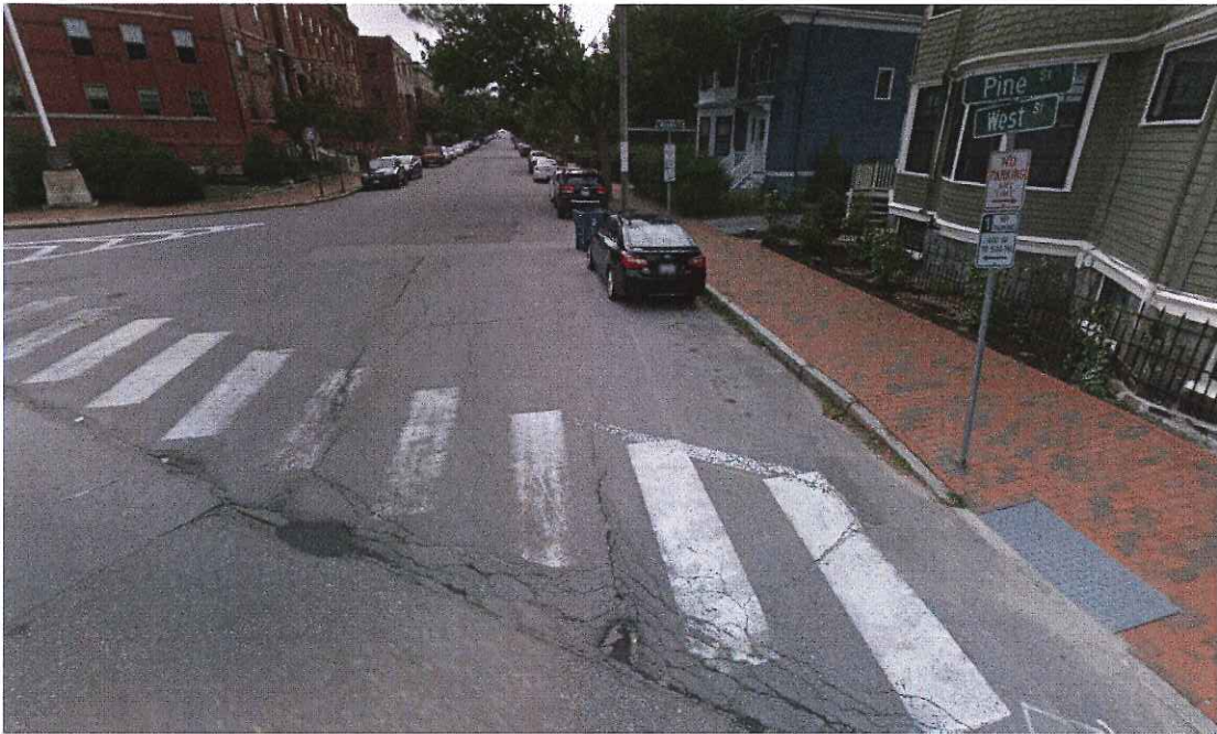
Photo 3: Composite detectable warning panels, granite curbing, and brick materials currently in place.
