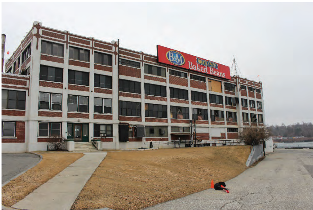
1. B&M Factory, West Elevation, looking southeast.
