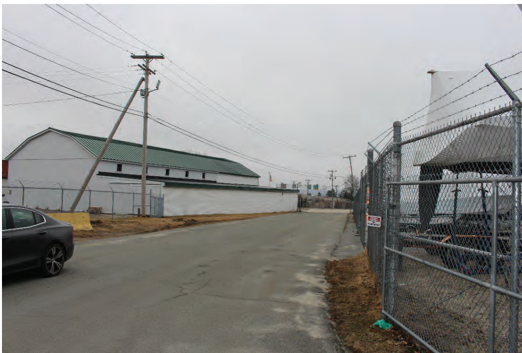
16. Site, Entrance and Woodworking/Storage Building looking south.
