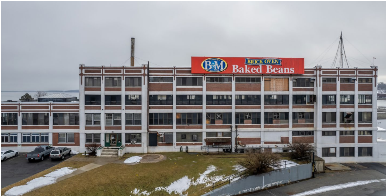
Existing conditions- west façade
