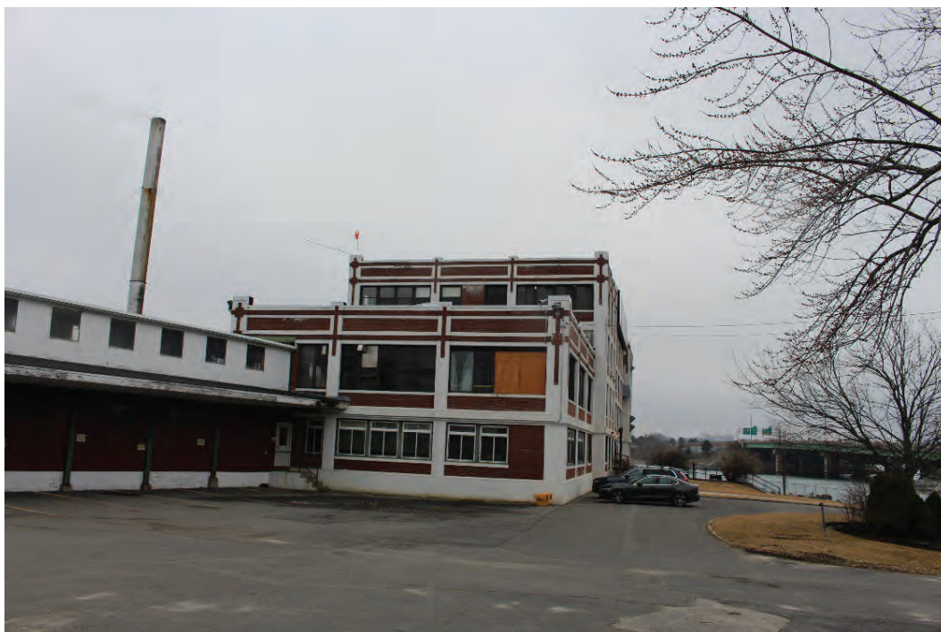
4. B&M Factory, North Elevation, looking south.
