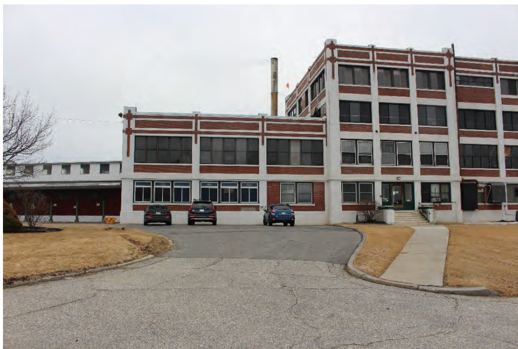
2. B&M Factory, West Elevation, looking east.
