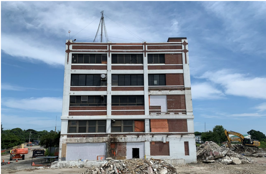
Existing conditions- south façade
