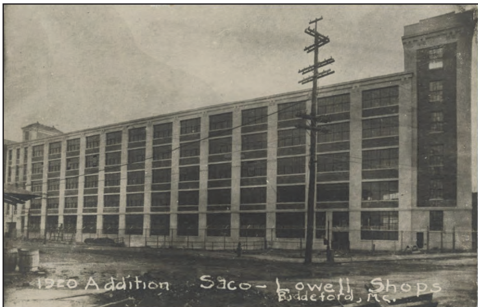
Figure 24: Saco-Lowell Shops Building 30 - Biddeford, Maine
