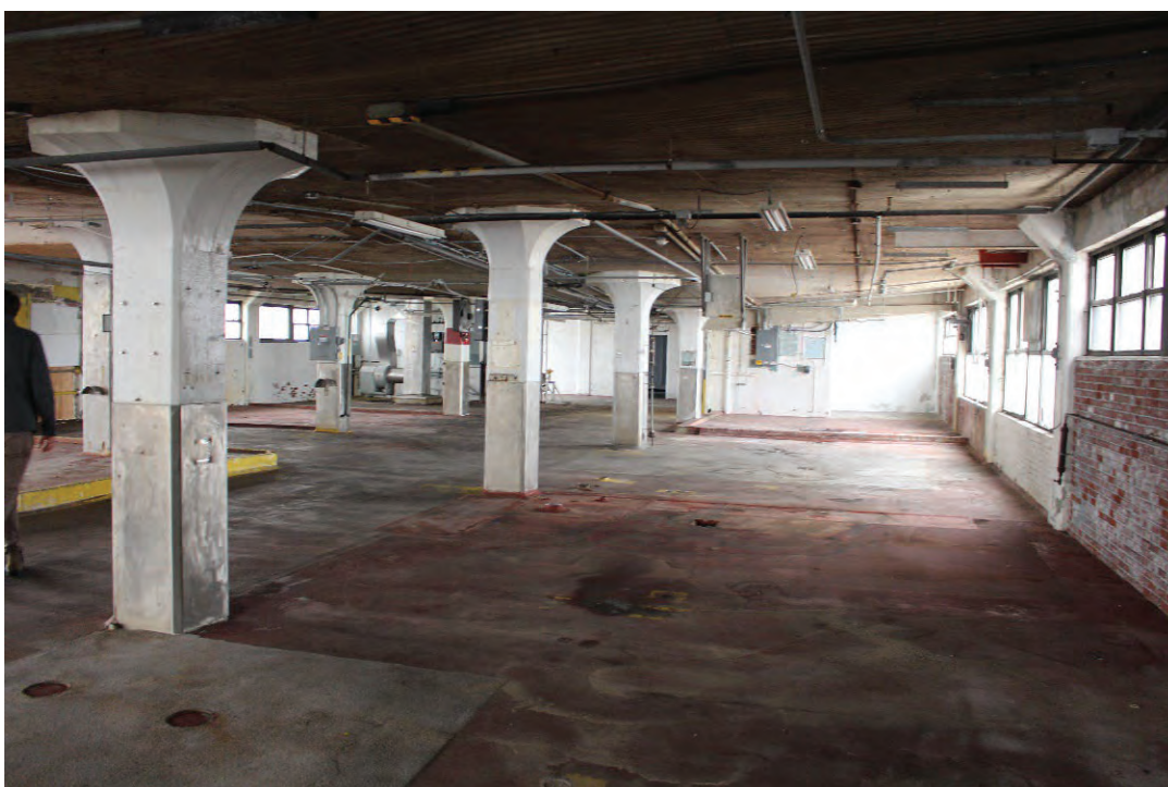
10. B&M Factory, Fourth Floor, looking south.
