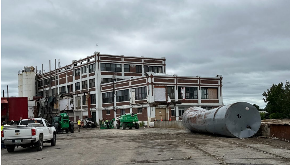
Existing conditions- north facade
