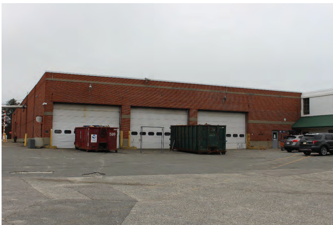
14. Site, Storage/Labeling Building looking northwest.
