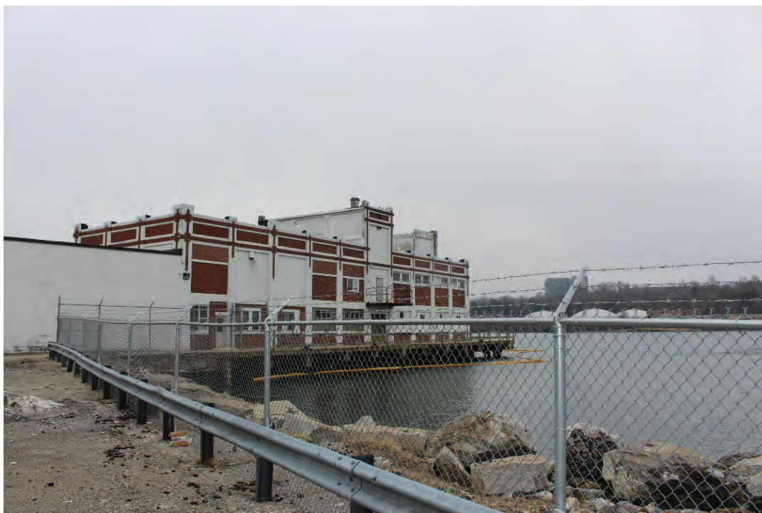
11. Site, Codfish Canning Building, looking southeast.
