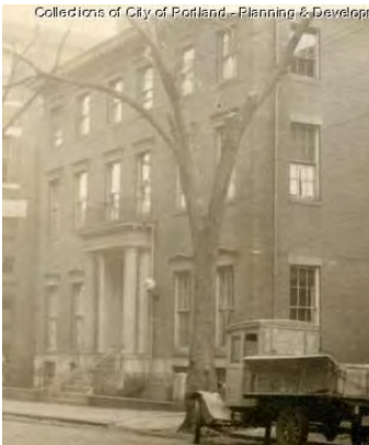
120-24 Free Street Demolished after 1960
