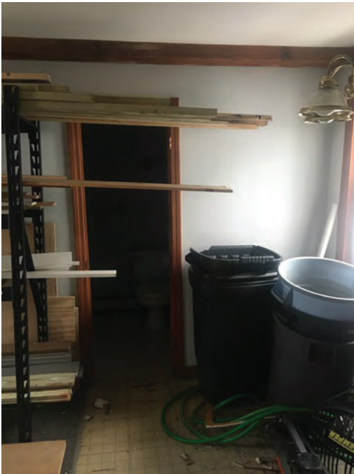
Photo #3 view of interior
