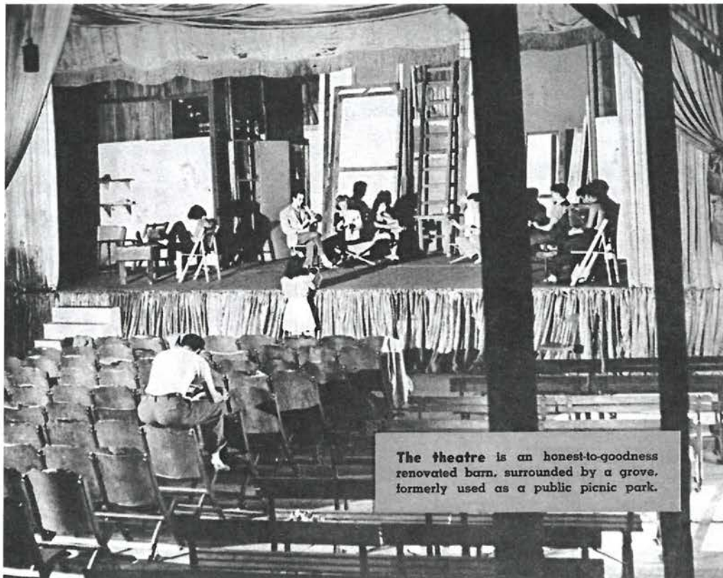
Figure 6 Theater interior, ca. 1940.
