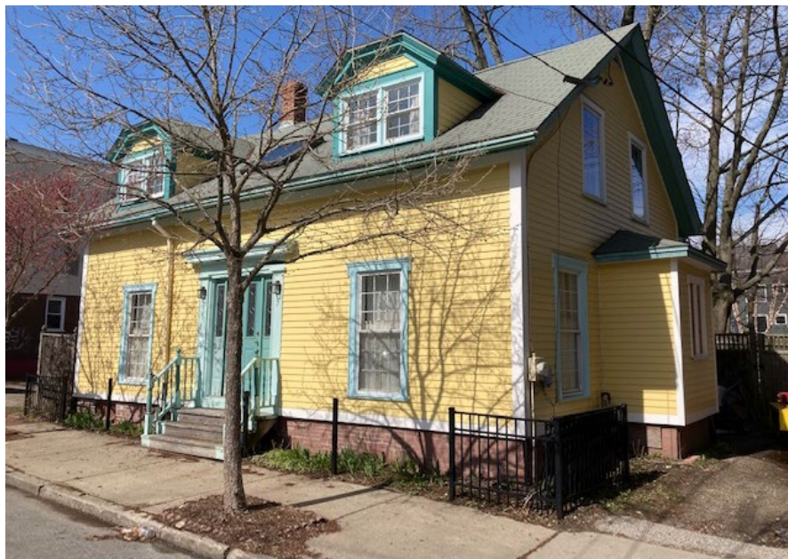
Figure 4: 7 Lafayette, 2022, after re-installation of clapboard siding
