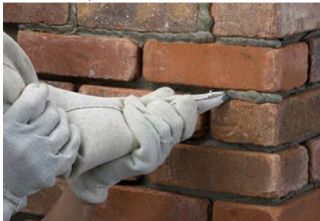
Photo 2 Mortar Placement Using a Grout Bag
