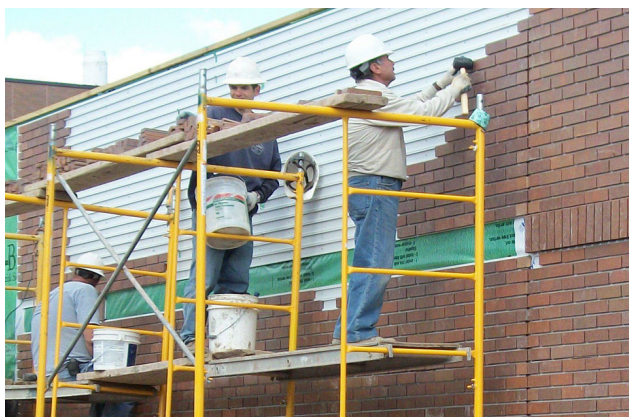
Photo 3 Installation of Modular Panel
