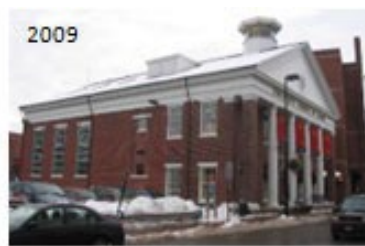
2009 142 Free Street as it appeared when it was designated as a contributing structure in the Congress Street Historic District.
