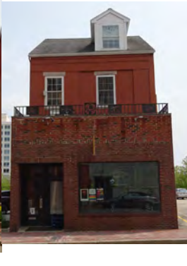
128 Free Street (extant; non-contributing)
