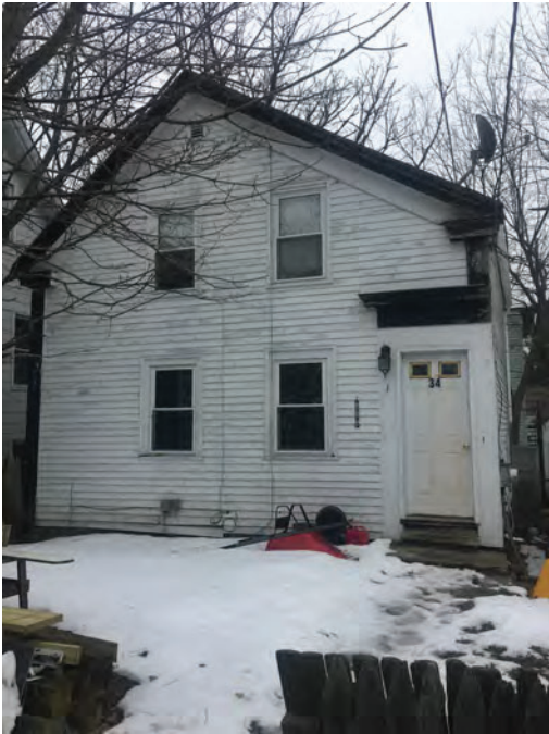
Photo #1 view of exterior of building
