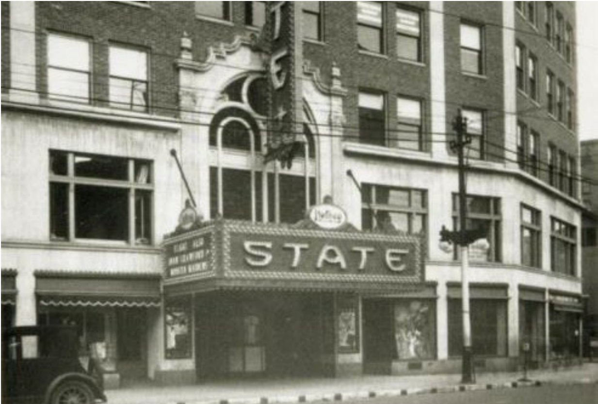
Figure 2: Detail from a circa 1930 image of the State Theater entrance from the collections of Maine Historical Society (Item 12894). Note the presence of the ticket booth beneath the marquee.
