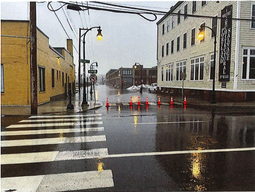
Figure 5: Bayside flooding as a result of excess stormwater runoff and record high tidal heights on January 13th, 2024.
