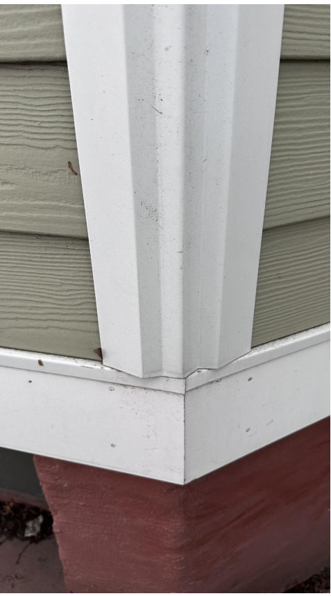
LEFT: NEW MDF WATER TABLE WITH DRIP CAP & ALUM. TRIM AT OUTSIDE CORNER OF BAY WINDOW.
