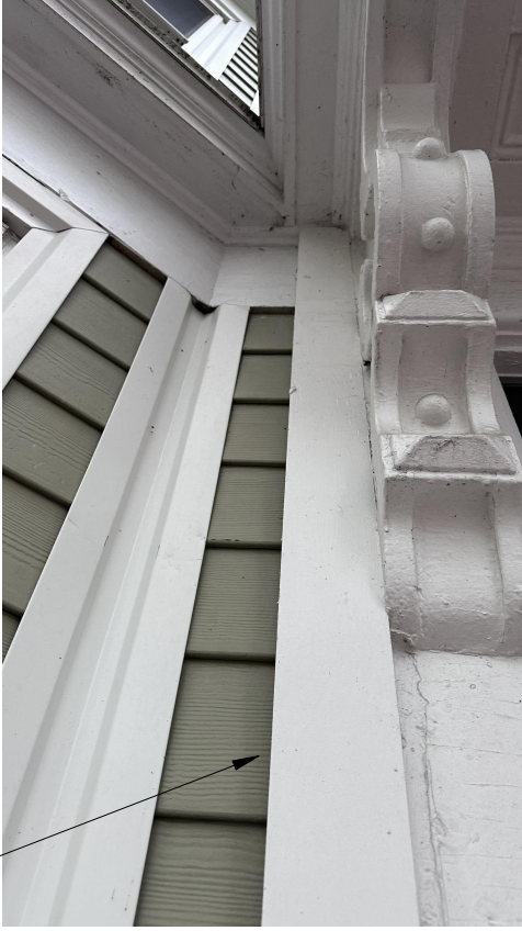
NEW TRIM PROVIDES TRANSITION @ ORIGINAL HOOD & HARDIPLANK SIDING
