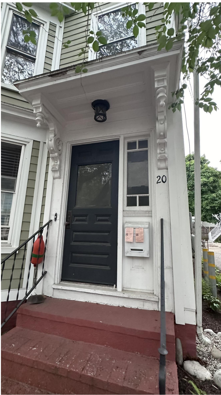
HOOD/ENTRY TRIM ASIDE FROM FACIA, CROWN MOLDING, & FRIEZE @ BAY WINDOW. FRONT STEPS ARE BRICK. IN 1924 PHOTO THEY ARE WOOD.
