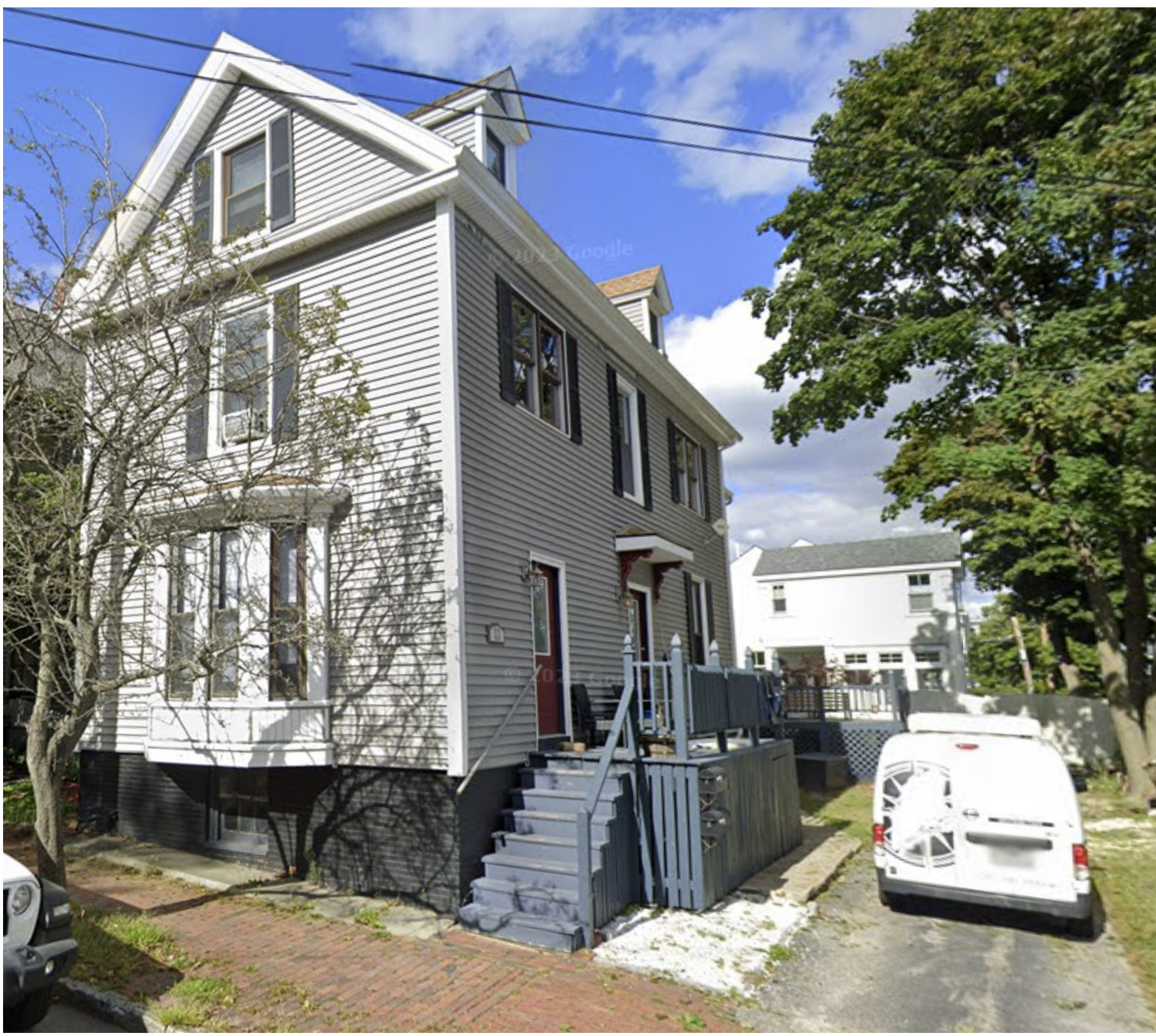
11 O'BRIEN NEW DORMERS & ADDITION W/WINDOWS CURRENTLY UNDER CONSTRUCTION. FAR LEFT: NEW DORMER EXTENDS TO STREETFRONT & STRUCTUALLY BEARS ON EXTERIOR WALL. IMMEDIATE LEFT: GOOGLE STREET VIEW CAPTURED SEPT. 2023 ILLUSTRATING CONDITION PRIOR TO ALTERATIONS IN PROGRESS.
