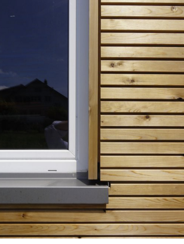
OPEN RAIN SCREEN EXAMPLE AT WINDOWS
