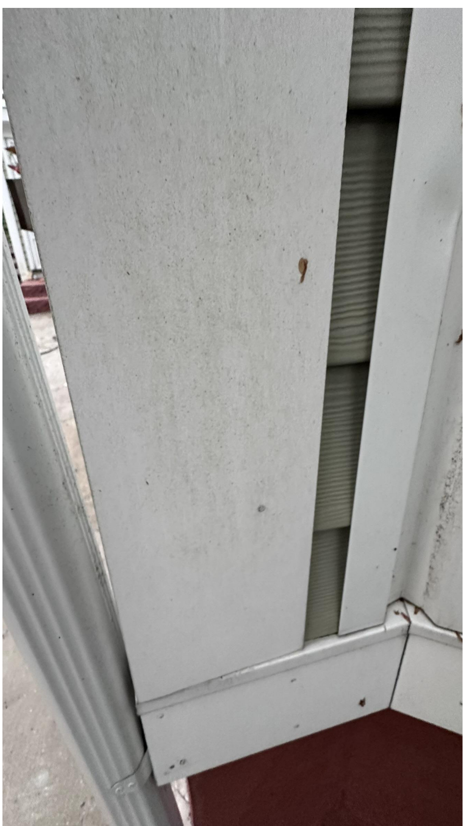
CORNER BOARD AND WATER TABLE & FRONT CORNER (DRIVEWAY SIDE)
