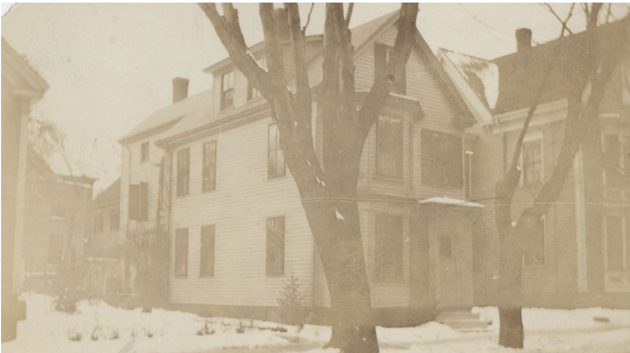
Figure 2: 1924 Tax Photo for 20 Morning Street.
