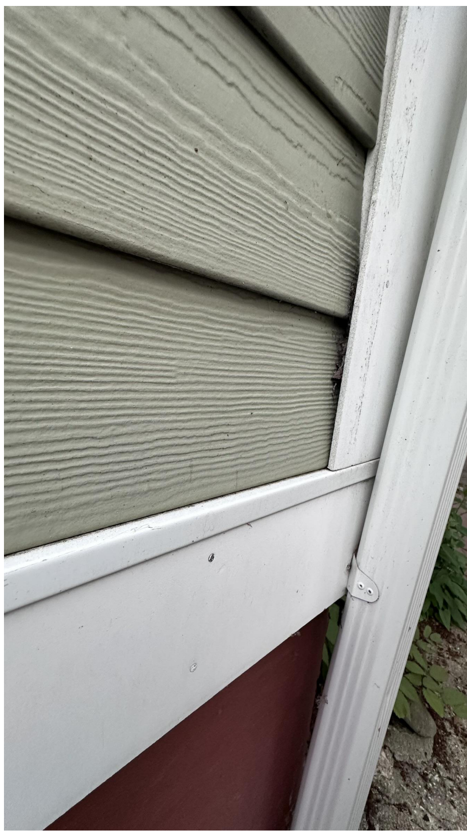
TEXTURED HARDIPLANK INSTALLED W/5" REVEAL. DRIP CAP & 5.5" WATER TABLE & NEW 5.5" CORNER BOARD.
