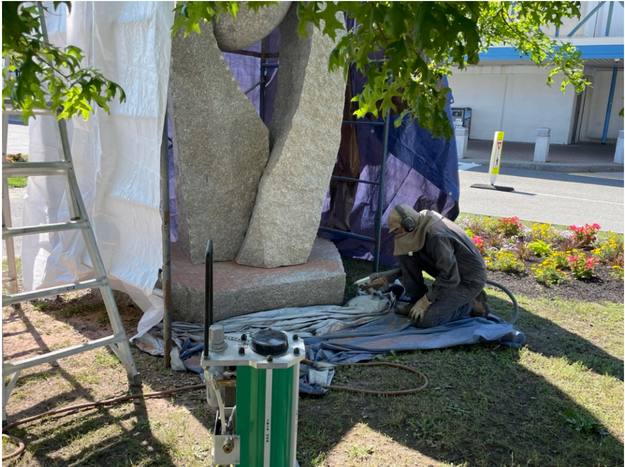
Photo of sand blasting with 230 grit restoration grade garnet. The entire sculpture was cleaned including paint and rust left after the collision and also lichen and moss that was growing on the sculpture. Additionally the car debris that remained stuck between the base stone and the sculpture was carved flush with the surface to make it less noticeable.
