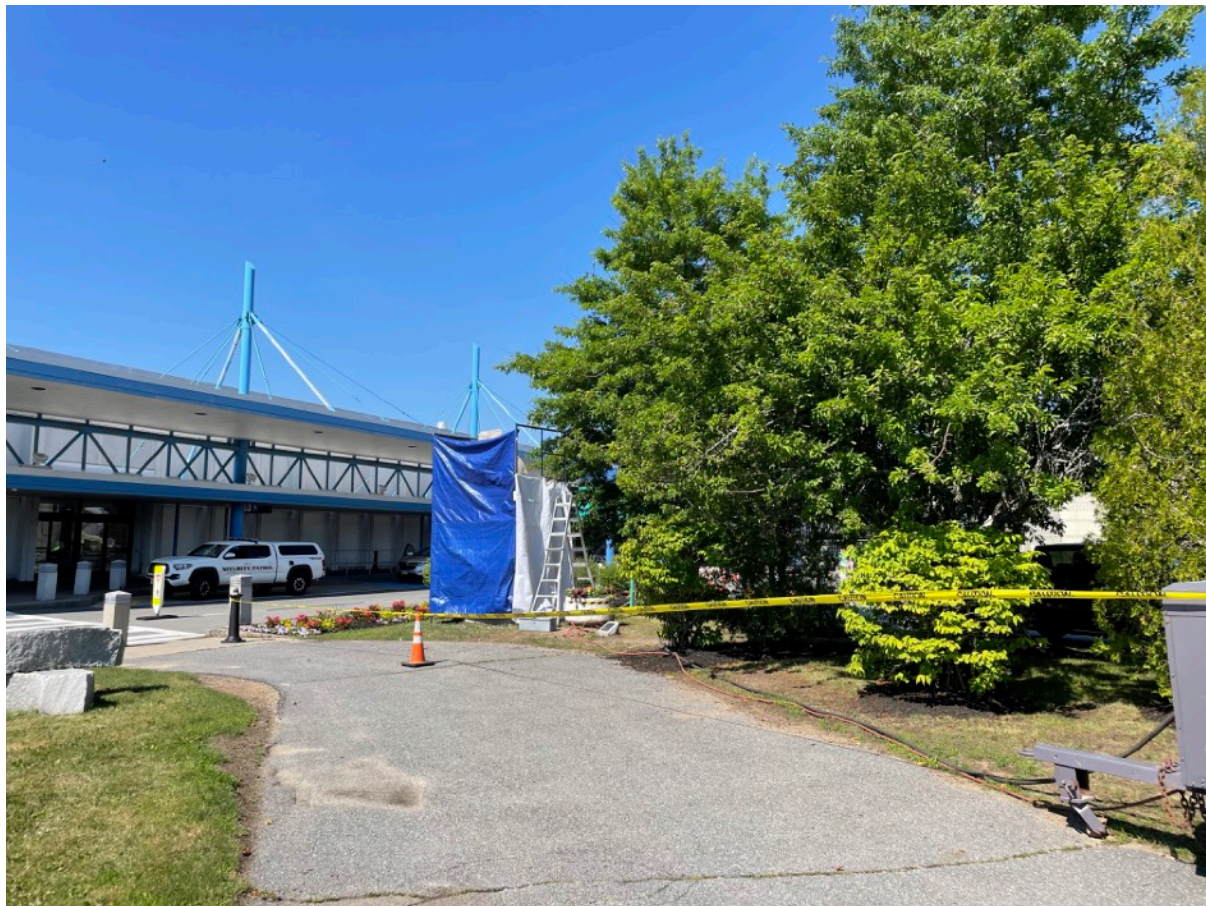
Photo of sculpture tented in to protect pedestrian traffic from dust and debris during cleaning. An additional perimeter was established with cones and DO NOT CROSS tape.
