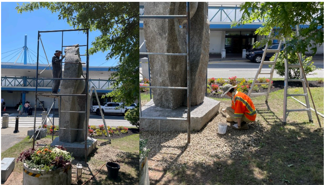
Photo of sand blasting with 230 grit restoration grade garnet. The entire sculpture was cleaned including paint and rust left after the collision and also lichen and moss that was growing on the sculpture. Additionally the car debris that remained stuck between the base stone and the sculpture was carved flush with the surface to make it less noticeable.
