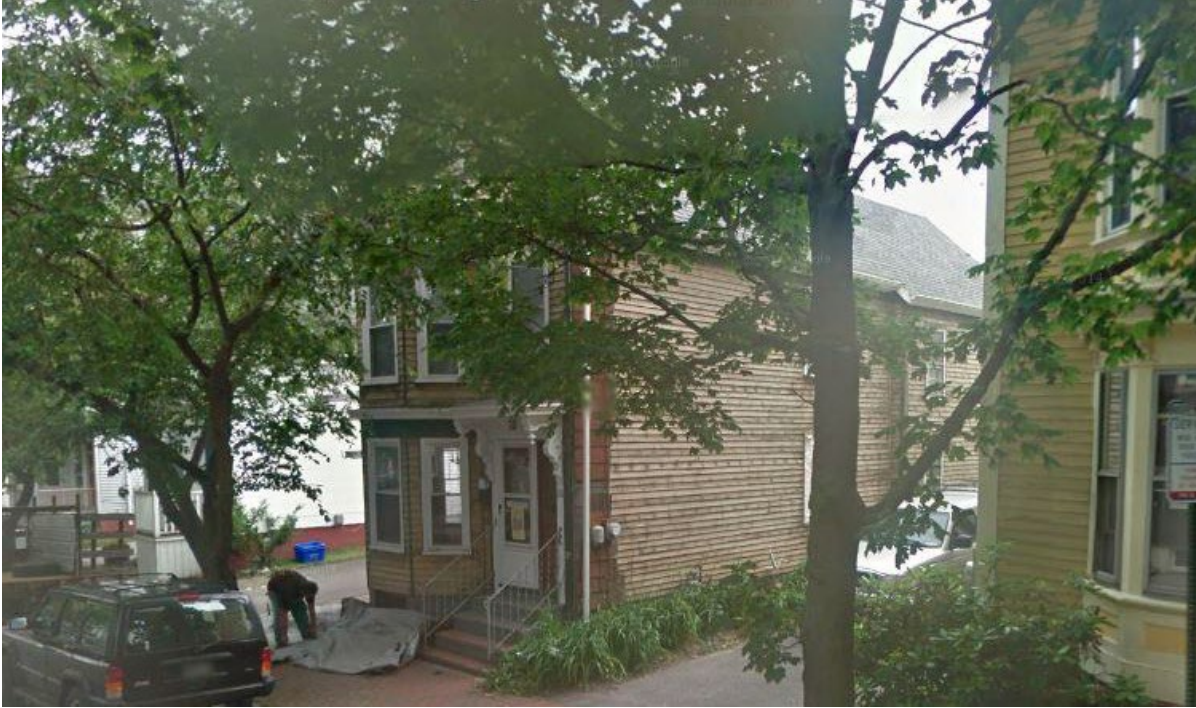
Figure 4: 2011 Google street view showing the shingle siding being removed.
