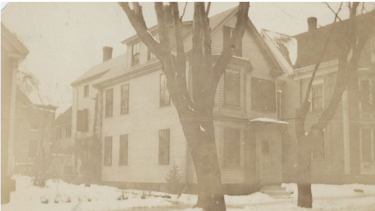
Figure 2: 1924 Tax Photo for 20 Morning Street.
