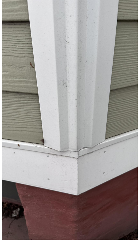
LEFT: NEW MDF WATER TABLE WITH DRIP CAP & ALUM. TRIM AT OUTSIDE CORNER OF BAY WINDOW.
