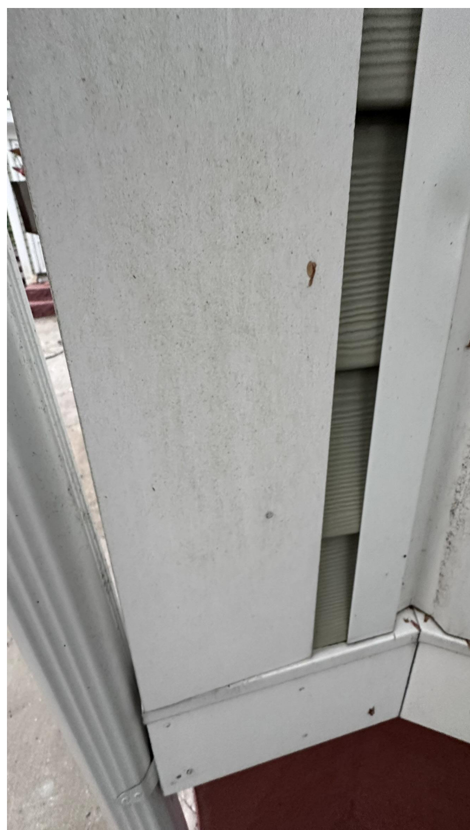
CORNER BOARD AND WATER TABLE & FRONT CORNER (DRIVEWAY SIDE)
