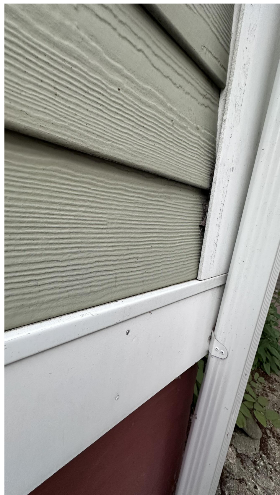
TEXTURED HARDIPLANK INSTALLED W/5" REVEAL. DRIP CAP & 5.5" WATER TABLE & NEW 5.5" CORNER BOARD.
