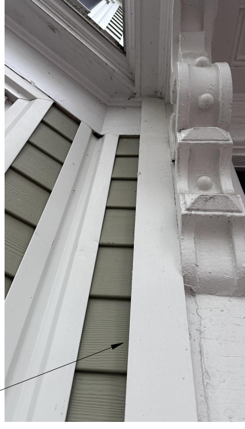
NEW TRIM PROVIDES TRANSITION @ ORIGINAL HOOD & HARDIPLANK SIDING
