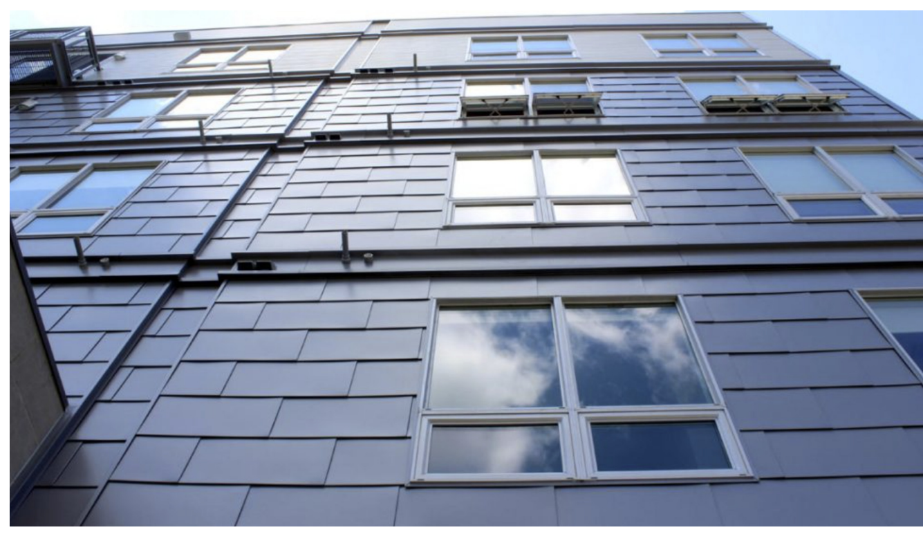
EXAMPLE OF METAL SINGLES (VERSA-LOK PANEL SHOWN)
